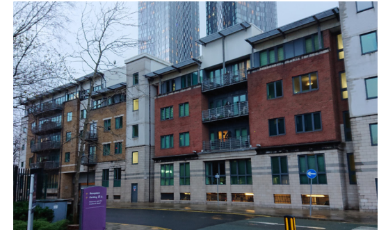
View of the rear of City South taken from River Street.
