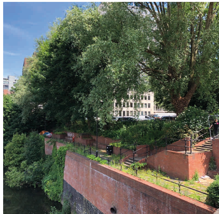
Figure 6.10 Low level pedestrian area facing the River Irwell
