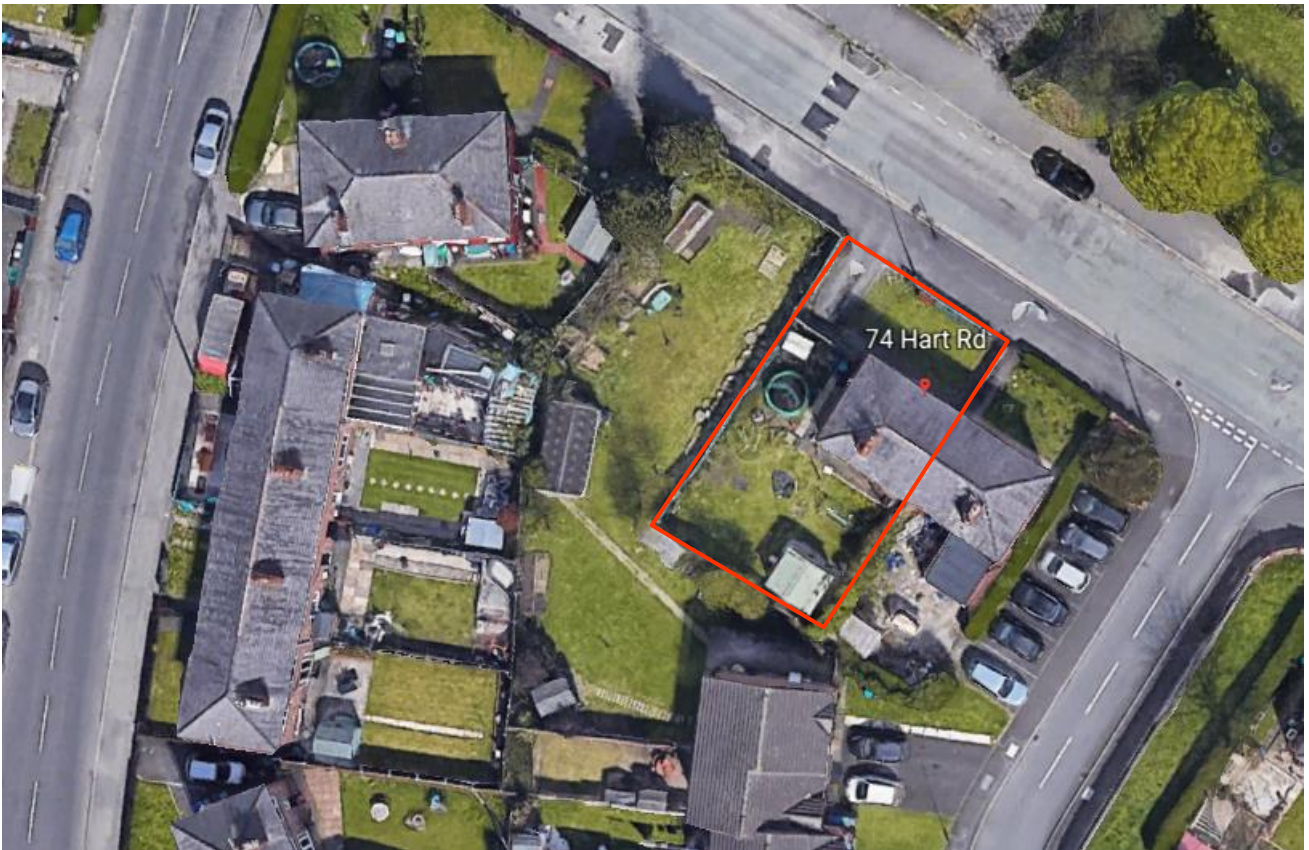
Figure 7. Screenshot from Google Earth, illustrating the immediate surroundings of No.74 Hart Road.
