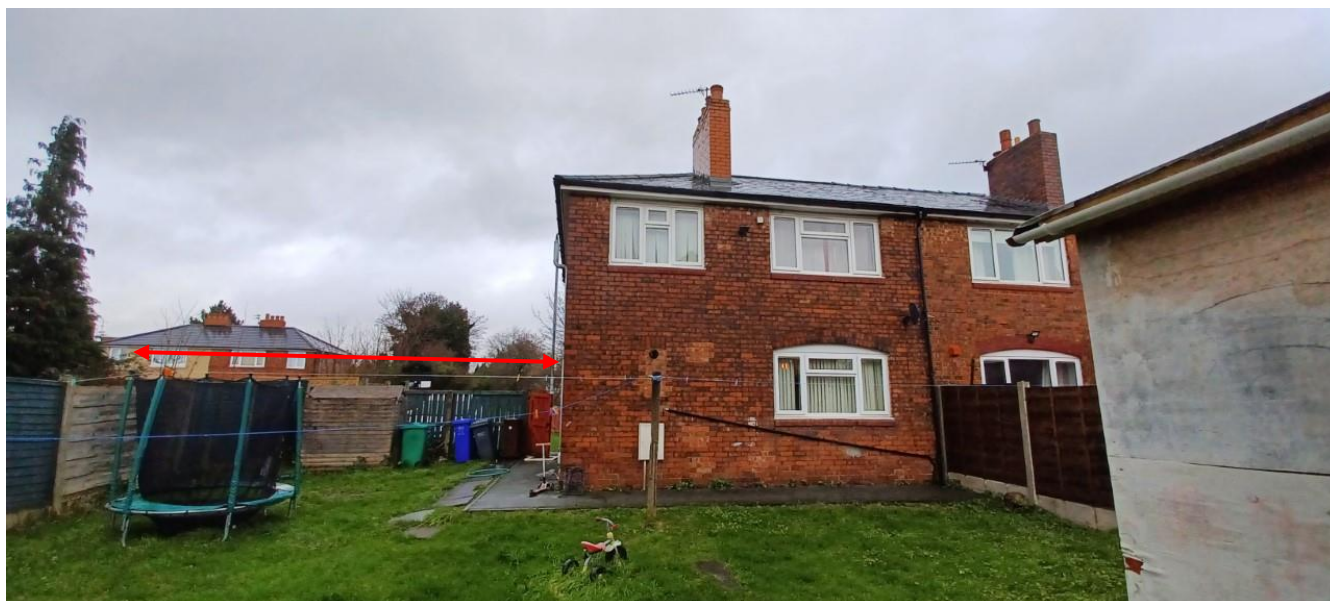
Figure 4. Photograph of No.74 Hart Road, depicting the substantial gap to the boundary shared with No.2 Plattbrook Close.
