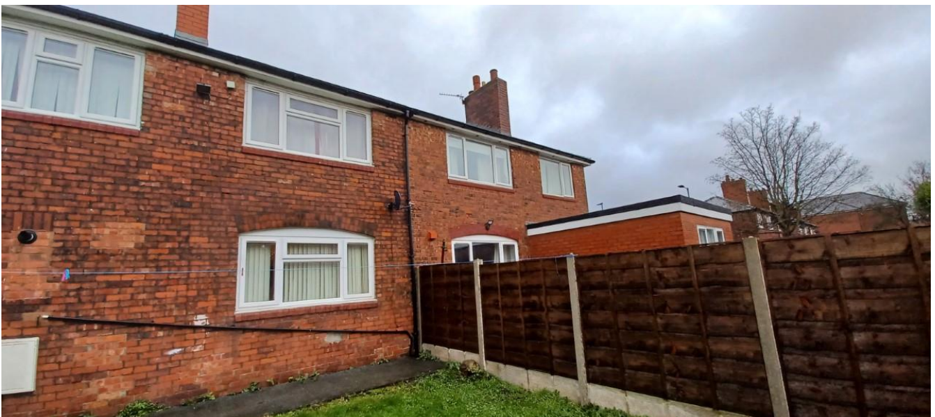
Figure 8. Photograph of the shared boundary between No.74 and No.76 Hart Road.
