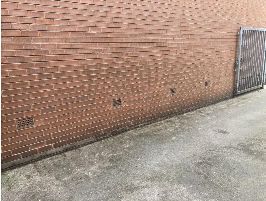
Photo 10. Wall of adjacent building to west showing air bricks
