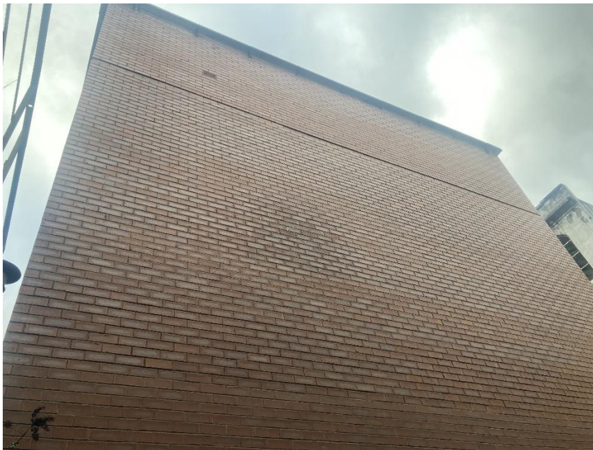
Photo 11. Wall of adjacent building showing slight eaves overhang and high-level air brick
