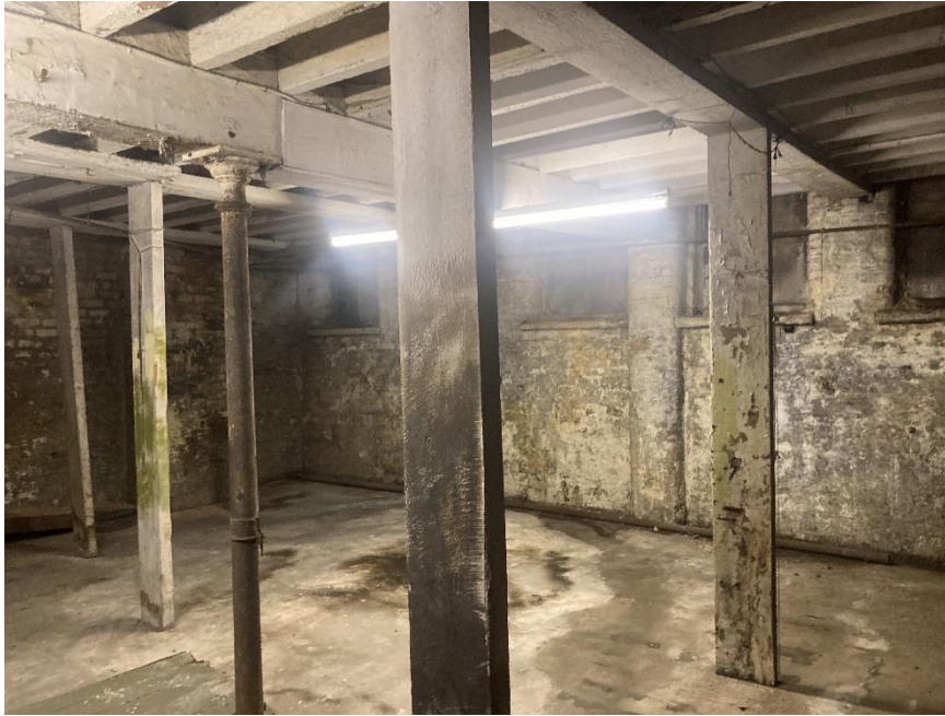
Photo 12. Ground floor construction visible within basement
