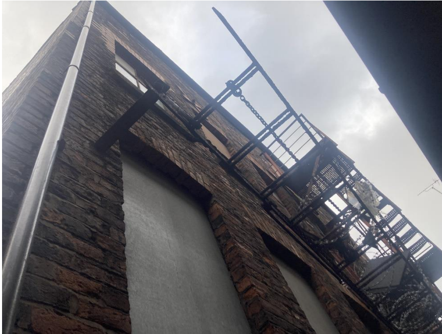
Photo 8. Rear (south) elevation
