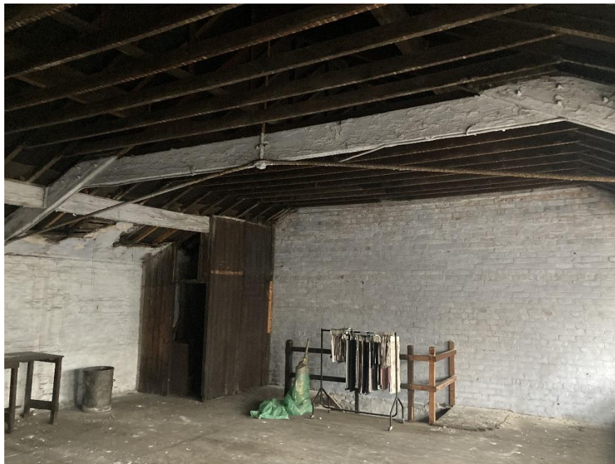
Photo 21. Roof structure visible at second-floor level
