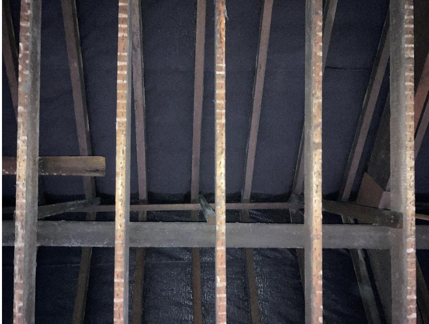
Photo 22. Timber roof racking to one side
