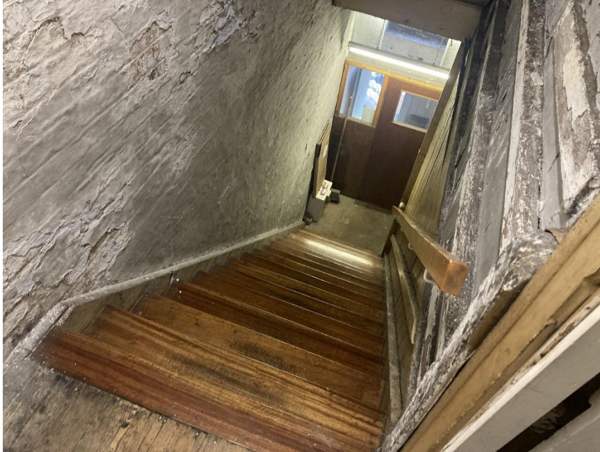
Photo 18. Stair adjacent west elevation
