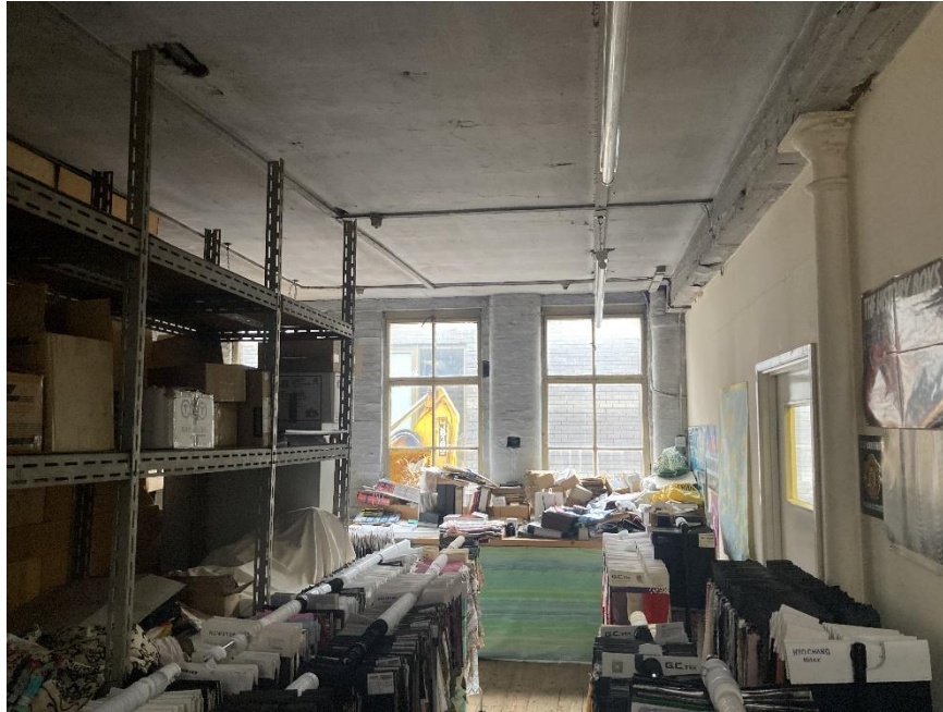
Photo 20. First-floor showing single cast-iron column
