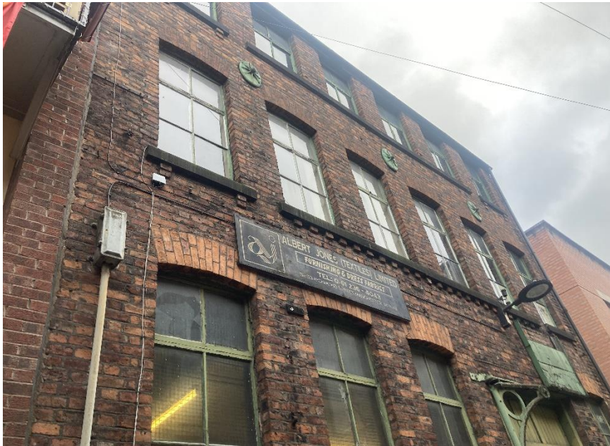
Photo 2. Front (north) elevation
