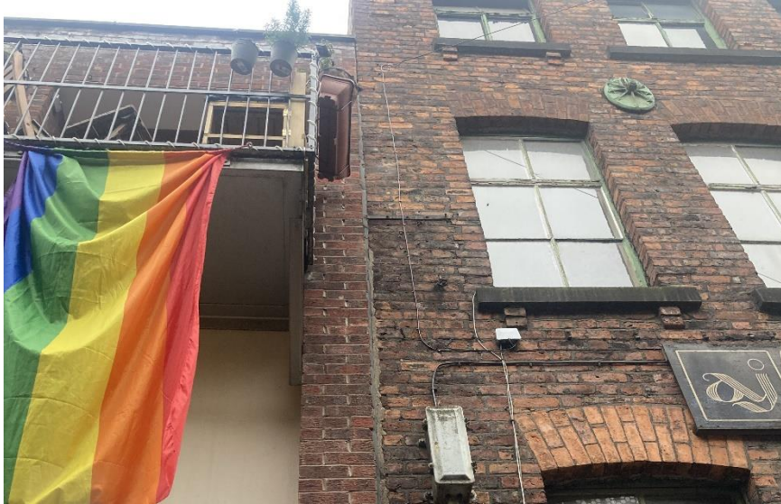
Photo 4. Full-height movement joint to left-hand party wall
