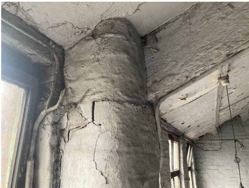
Photo 26. Cracking at spring point of roof truss to front elevation
