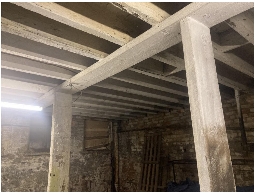
Photo 13. Historic timber propping to mid-span of ground-floor joists
