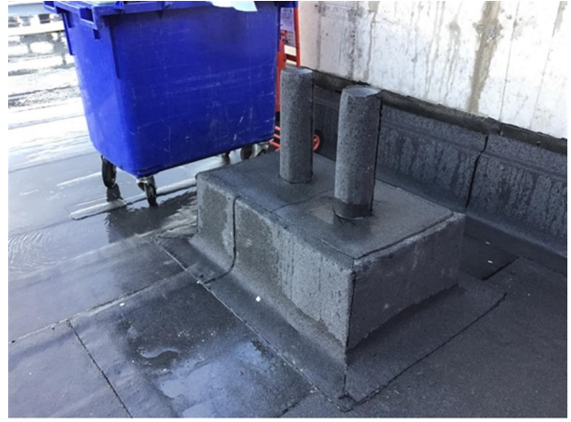
Photo 8 - View of SVP detail to section 1
