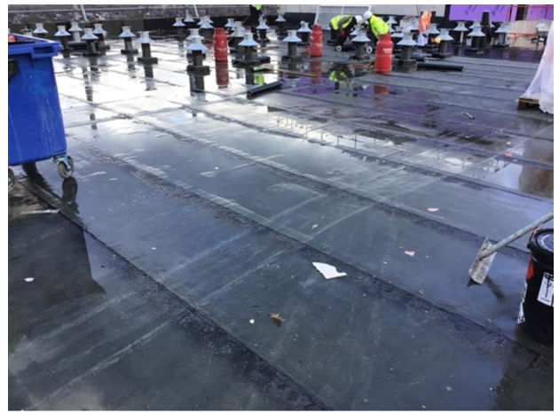
Photo 4 - View of AVCL to section 3
