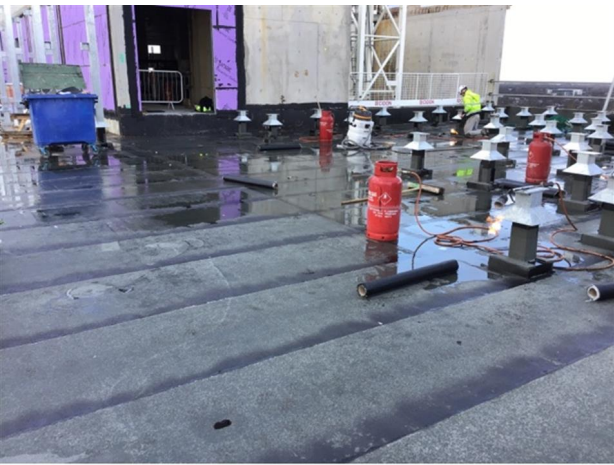
Photo 3 - View of AVCL to section 3
