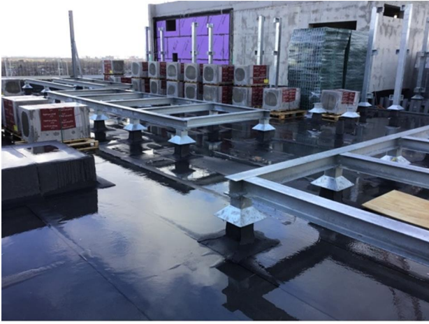
Photo 7 - View of section 1
