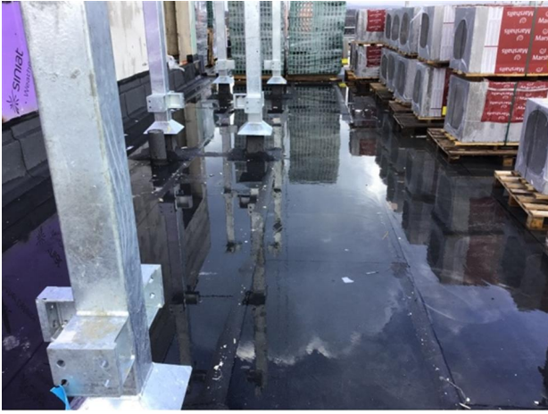
Photo 13 - View of section 1
