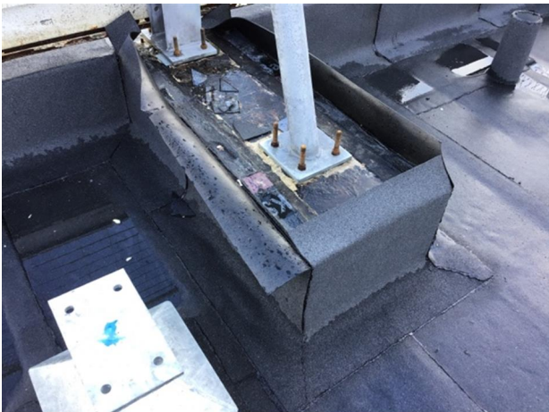
Photo 11 - View of perimeter plinths to be completed
