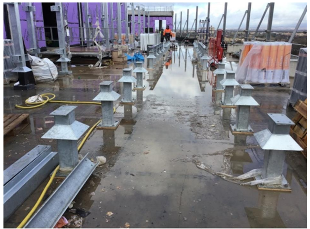
Photo 16 - View of section 2
