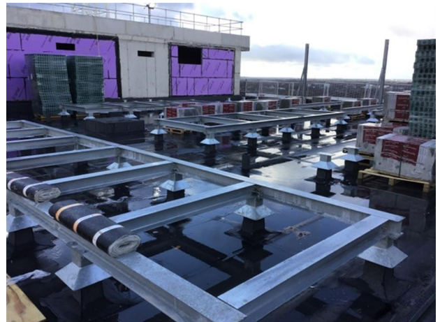
Photo 6 - Overview of section 1
