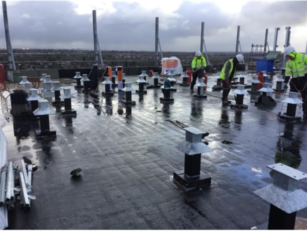
Photo 1 - View of progress to section 3
