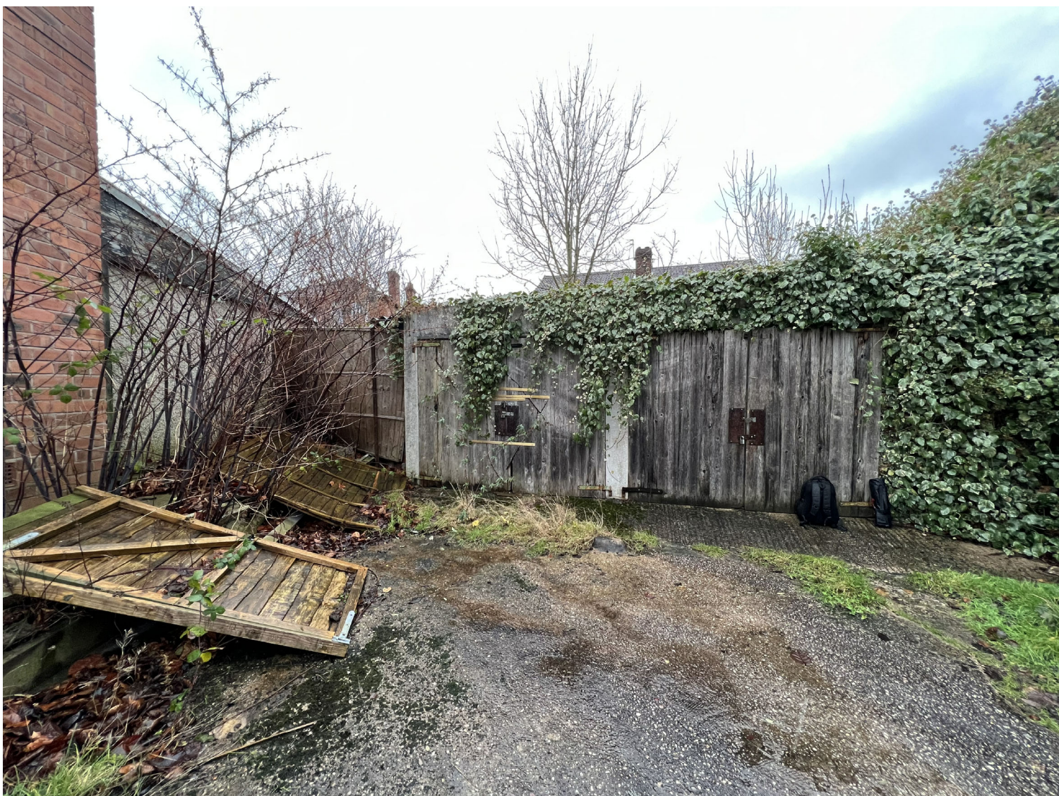
04 SITE PHOTOGRAPH Existing dilapidated double garage structure to rear of site
