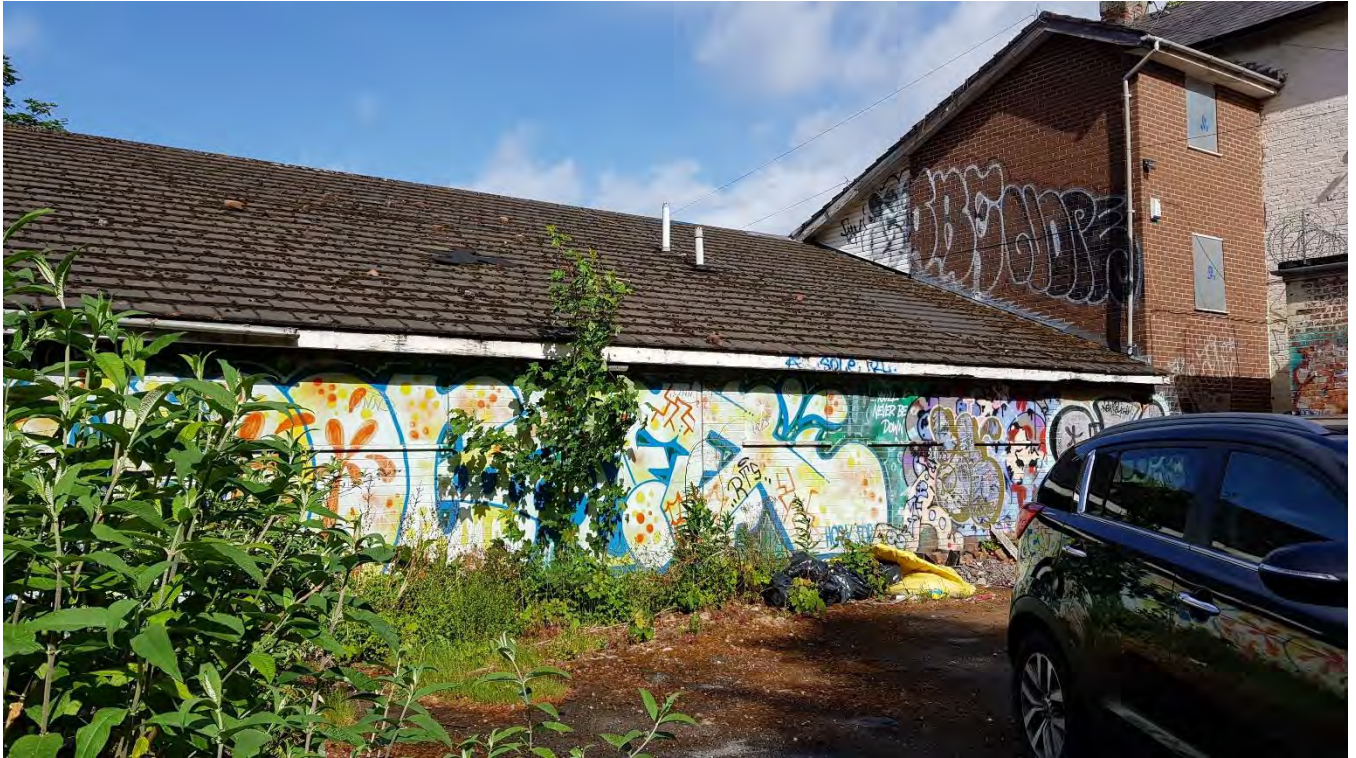
Rear SE extension – single storey with two storey link against the original building
