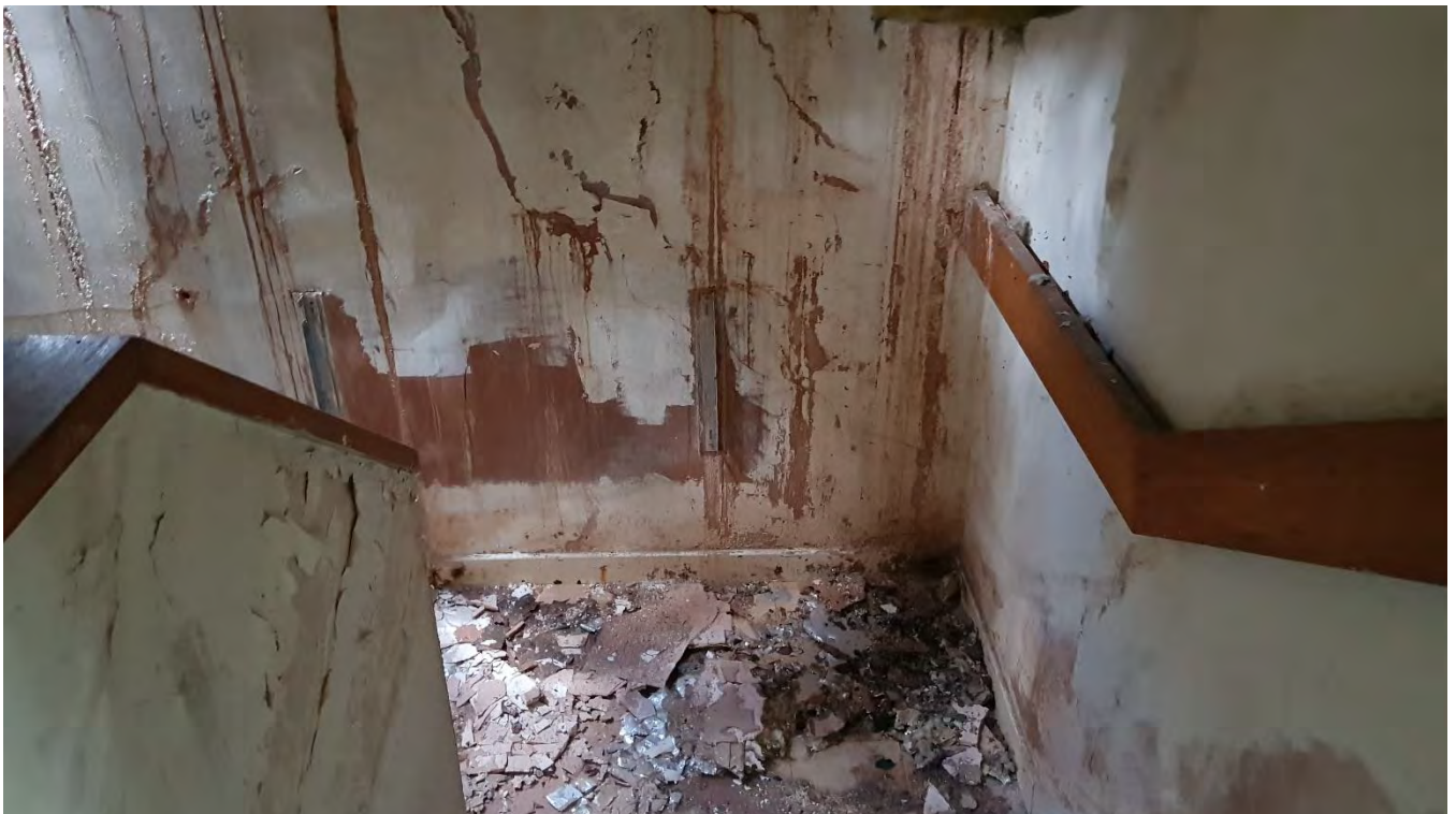
The stair below the previous photo
