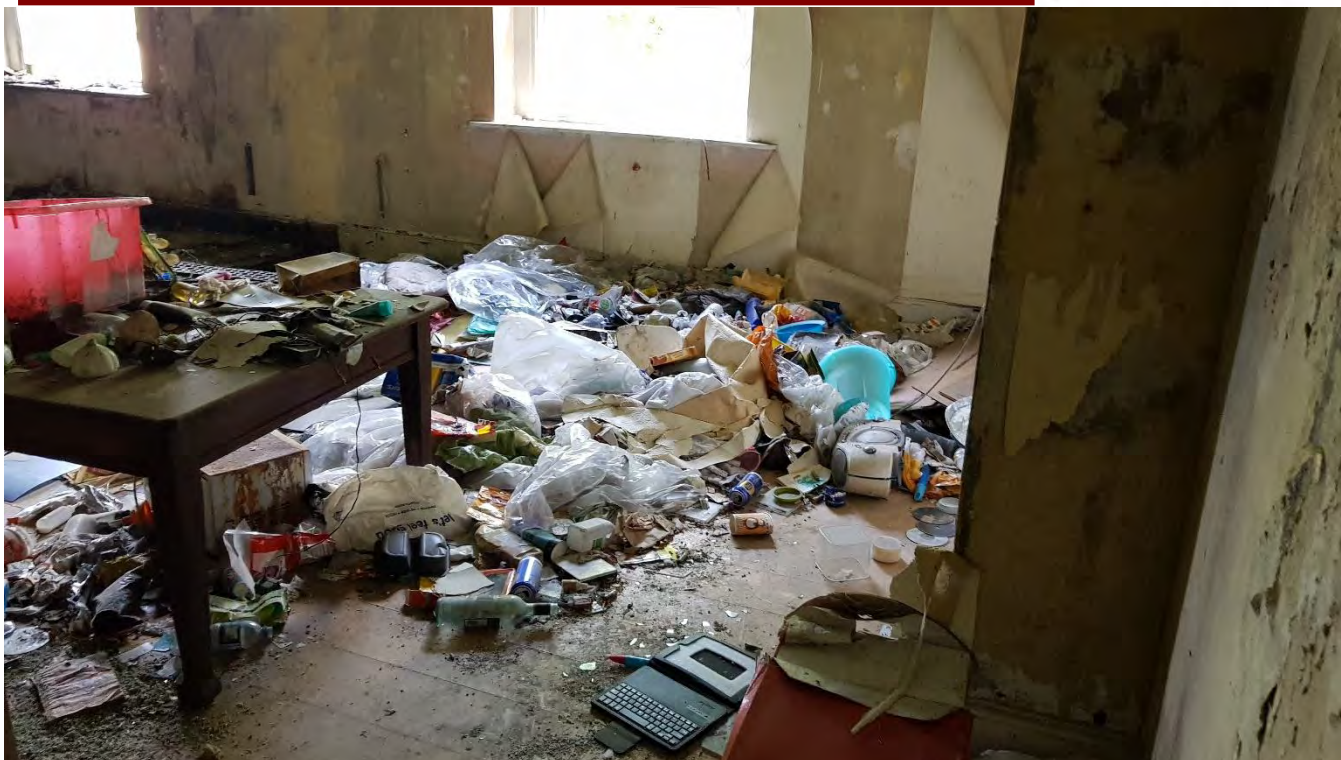
Debris to first floor
