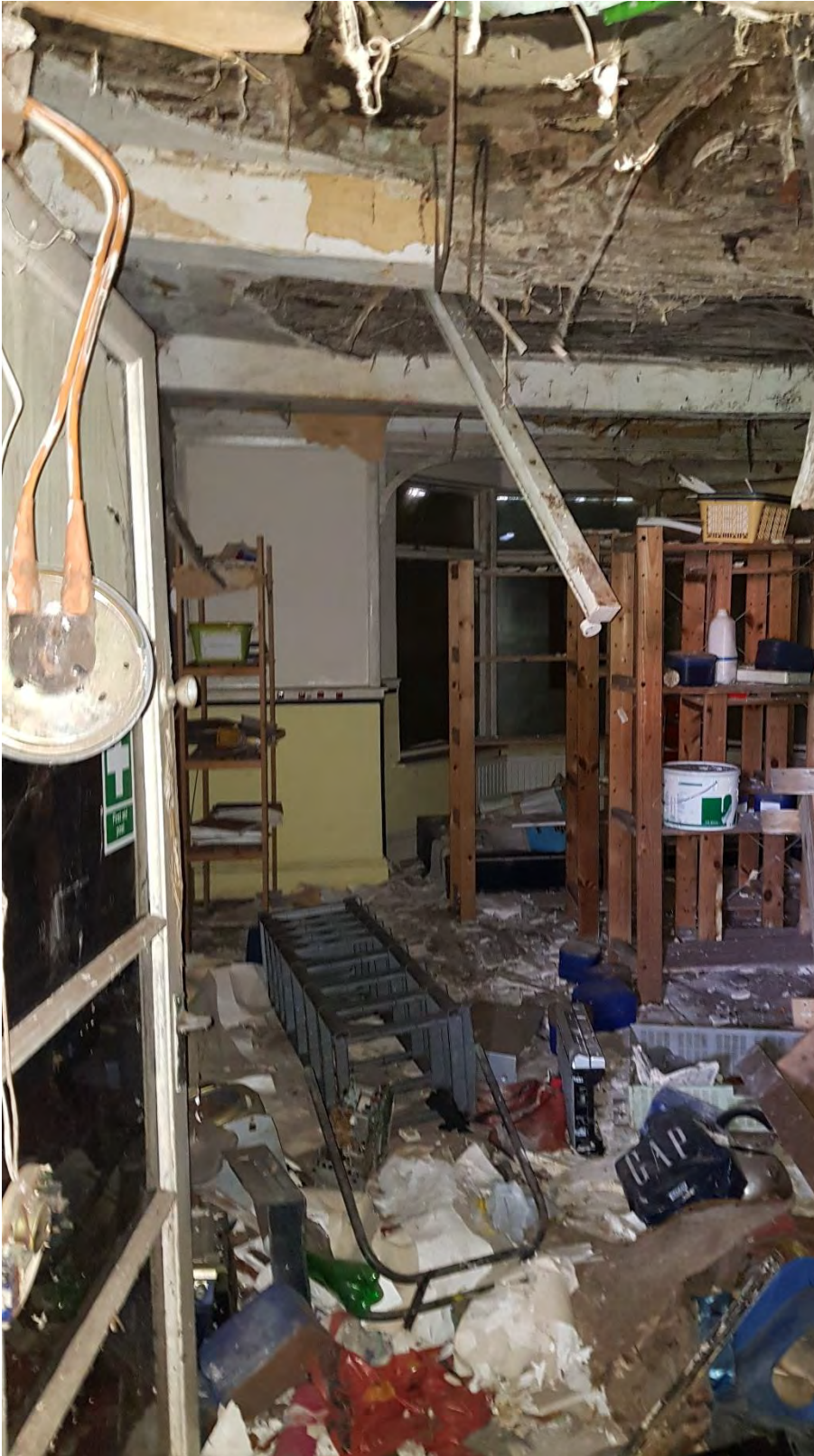
Ground floor – original house – east end of north wing.
