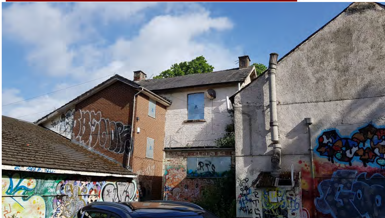
Original building to the right and in the background – possible asbestos flue in the foreground
