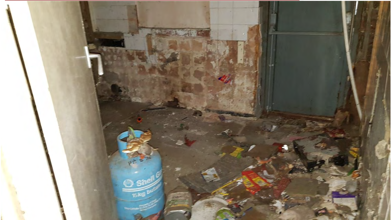
Kitchen area behind west facing door of the south wing of the original house
