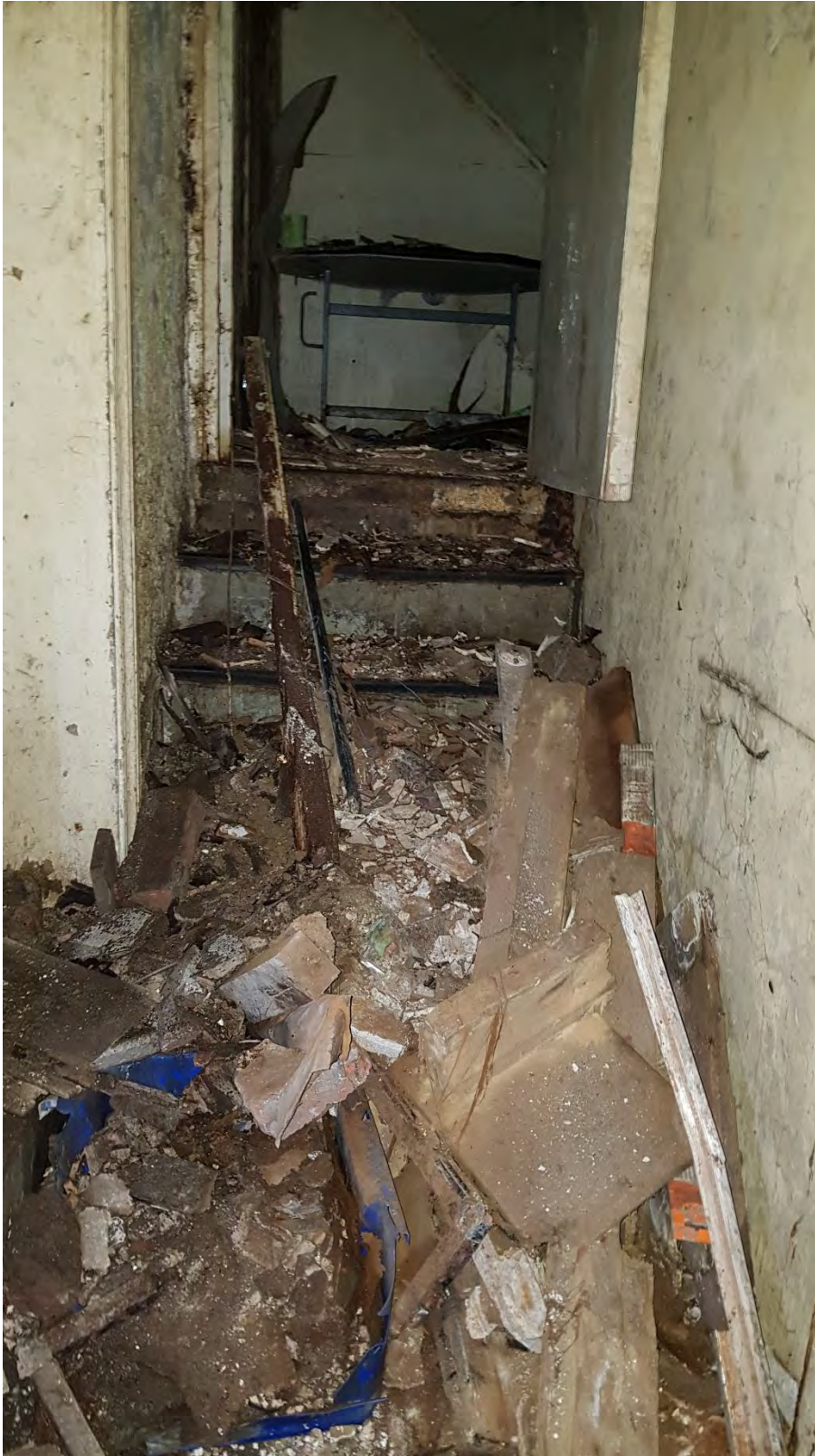
Stairs up from basement area
