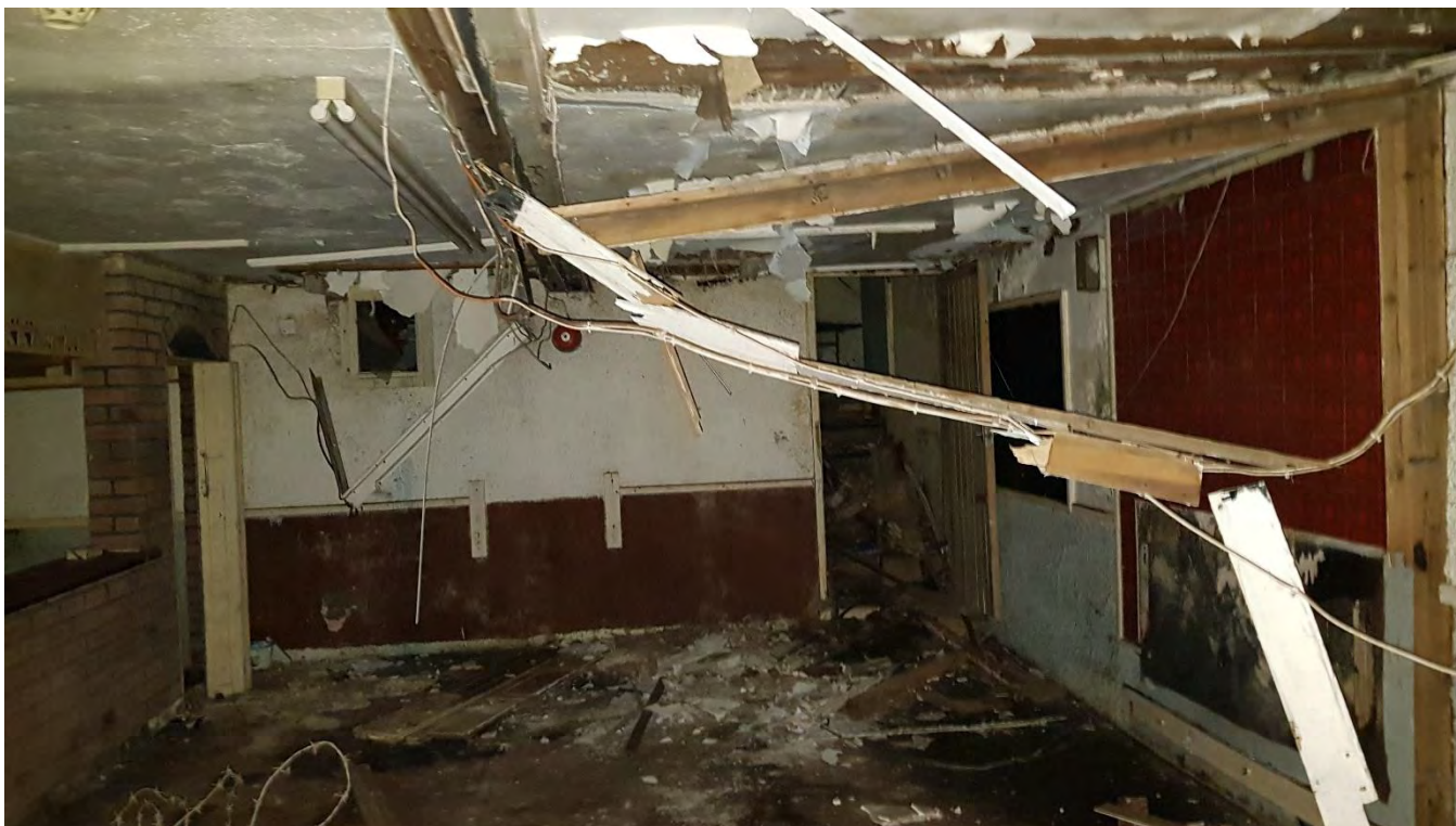
Partial basement area of original building
