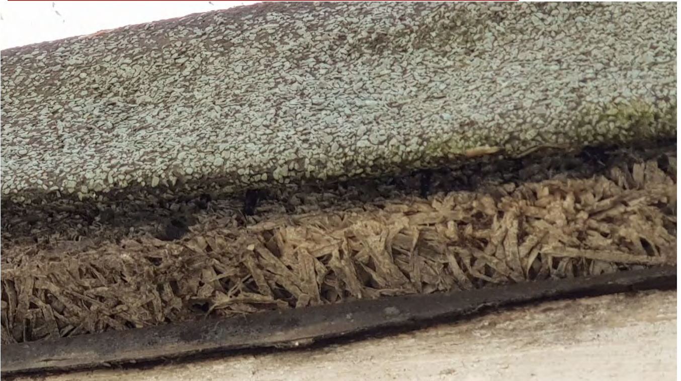
Woodwool slabs used to the flat roof of the original west entrance.
