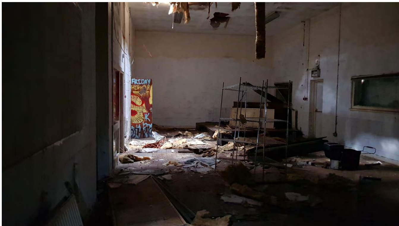
Single storey extension
