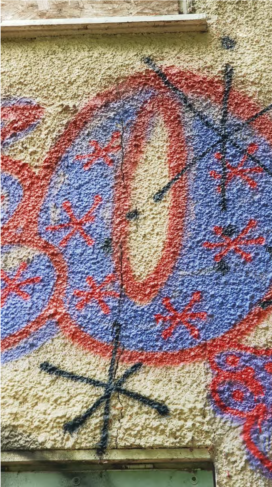
Cracking to external render – east elevation
