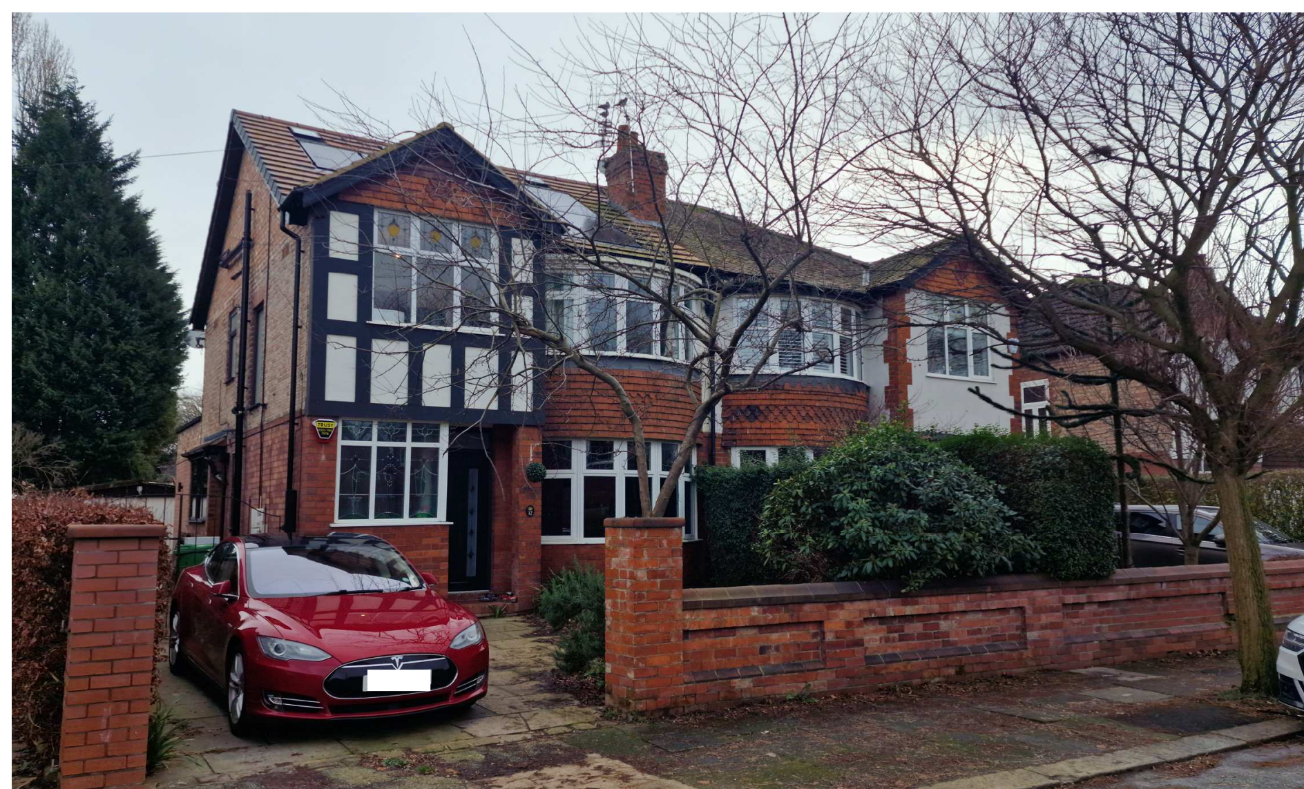
Existing Site Photo 11/01/23
