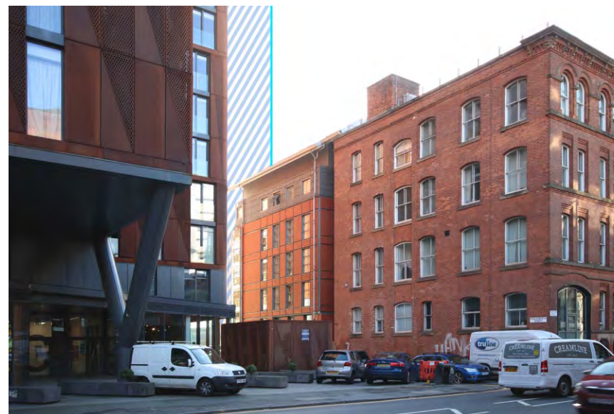
View 11 - Oxid House
