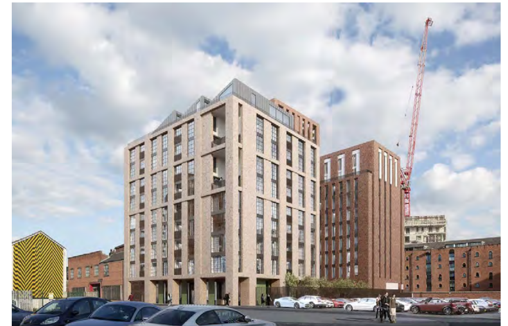
Scheme CGIs (Source: 5Plus Architects ( http://5plusarchitects.com/projects/tariff-street/ ))
