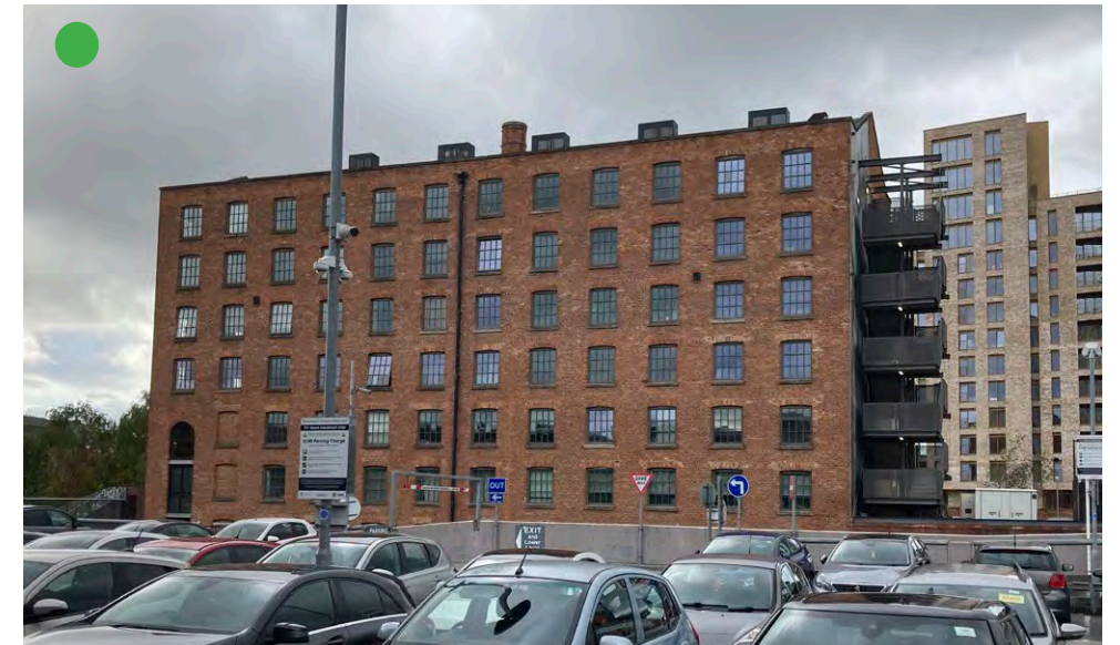
PRESENT : Exterior view of Jackson's Warehouse
