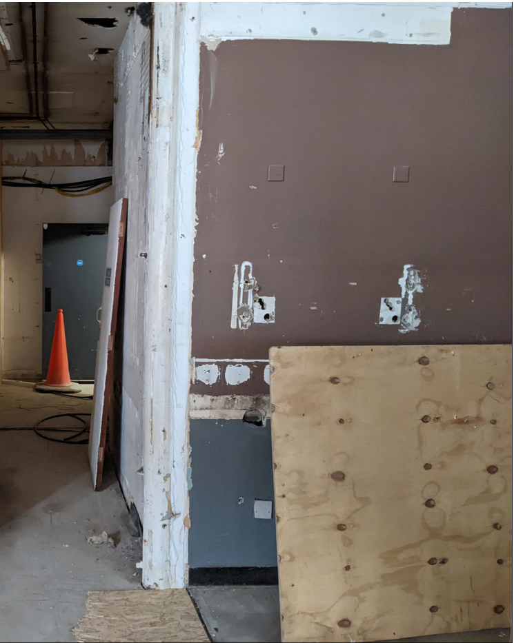
IMAGE SHOWING EXISTING BUT NON-ORIGINAL STUD WALL
