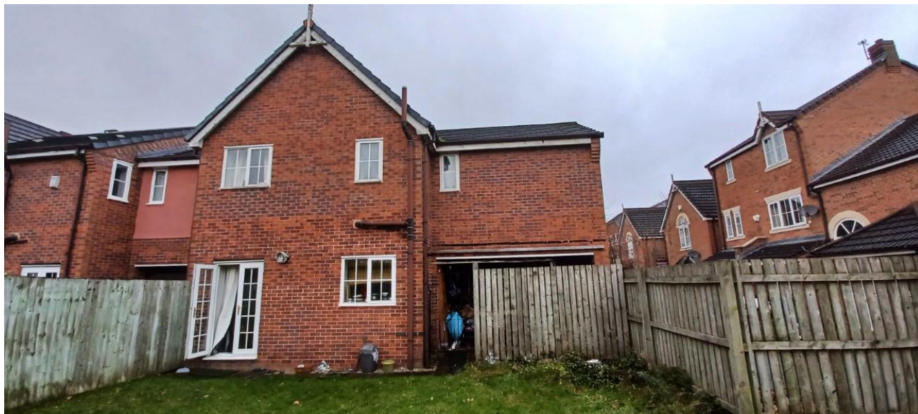
Figure 2. Photograph of the rear elevation of No.34 Chervil Close.
