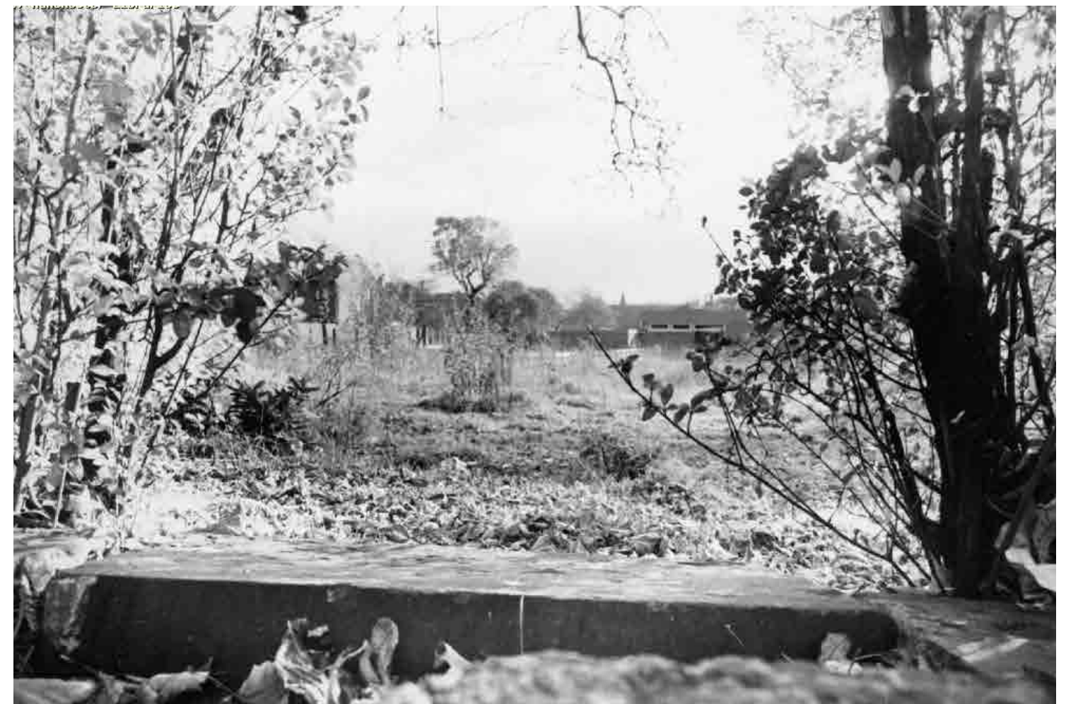
SITE AFTER STAFFORD HOUSE DEMOLISHED 1974
