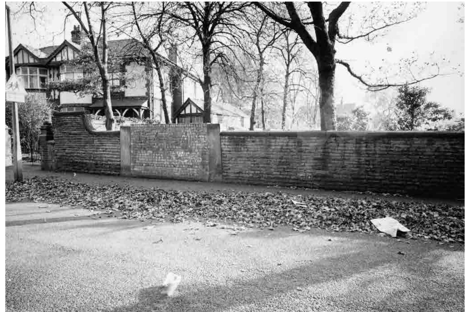
BOUNDARY OF SITE AFTER STAFFORD HOUSE DEMOLISHED 1974
