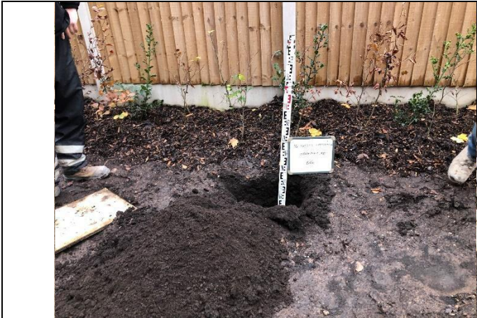
P19: Shared Landscaping – Validation Location 2
