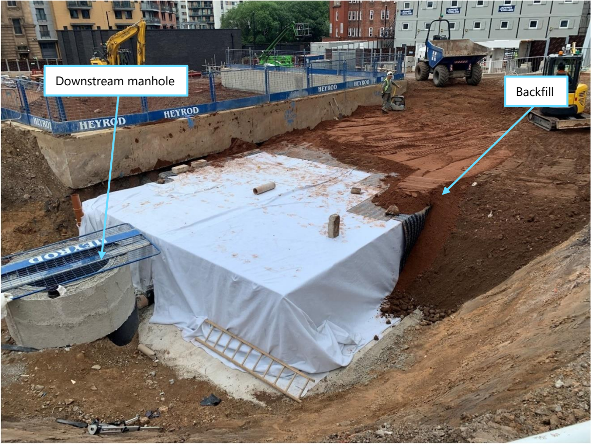
Figure 2-3 Backfilling on Attenuation Tank 1
