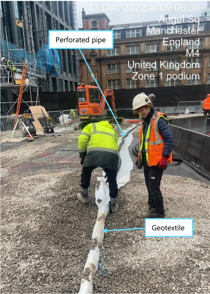
Figure 2-4 Perforated pipe installation in permeable paving system
