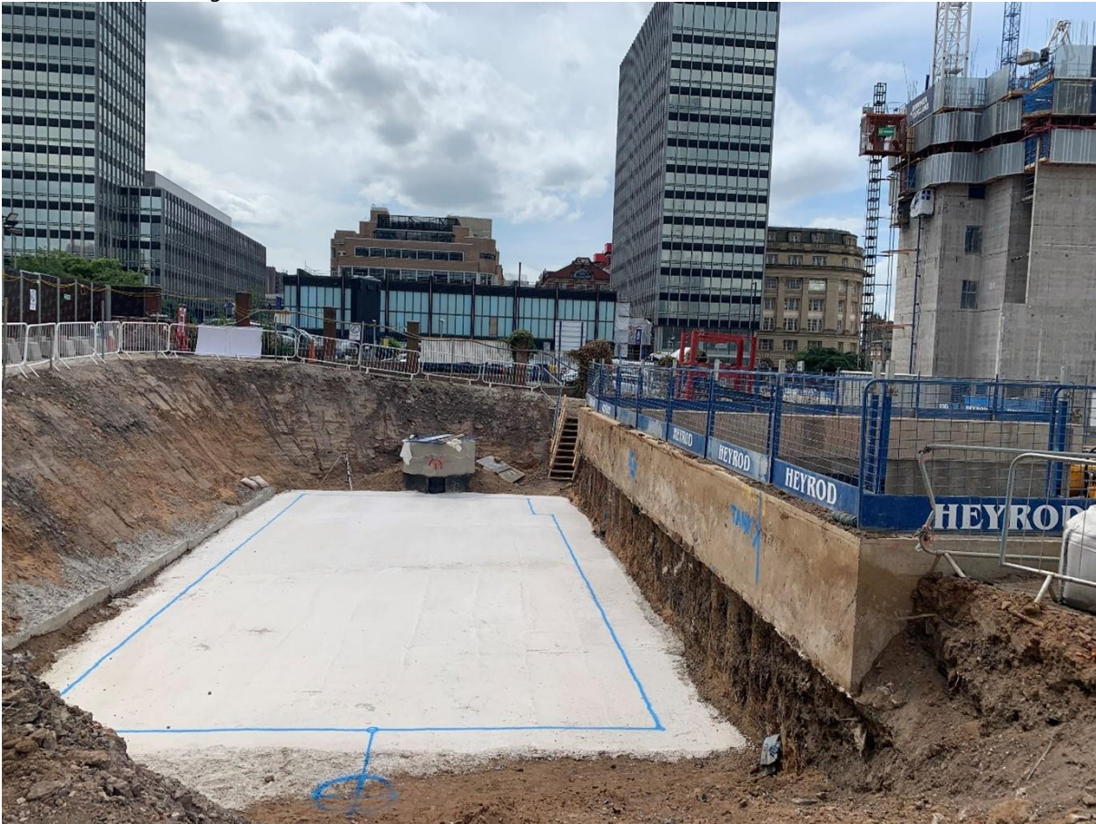
Figure 2-1 Ground preparation for Attenuation Tank 1
