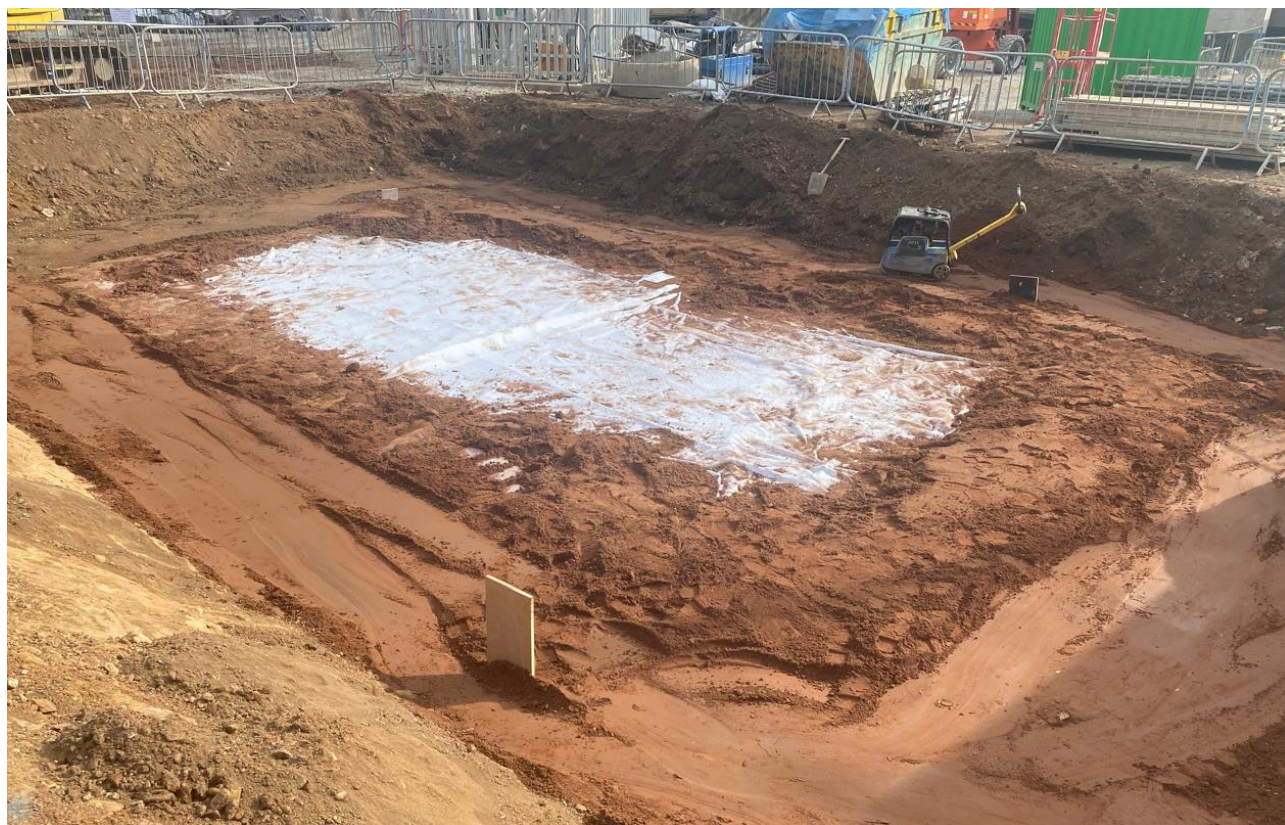
Figure 2-8 Backfilling of Attenuation Tank 2
