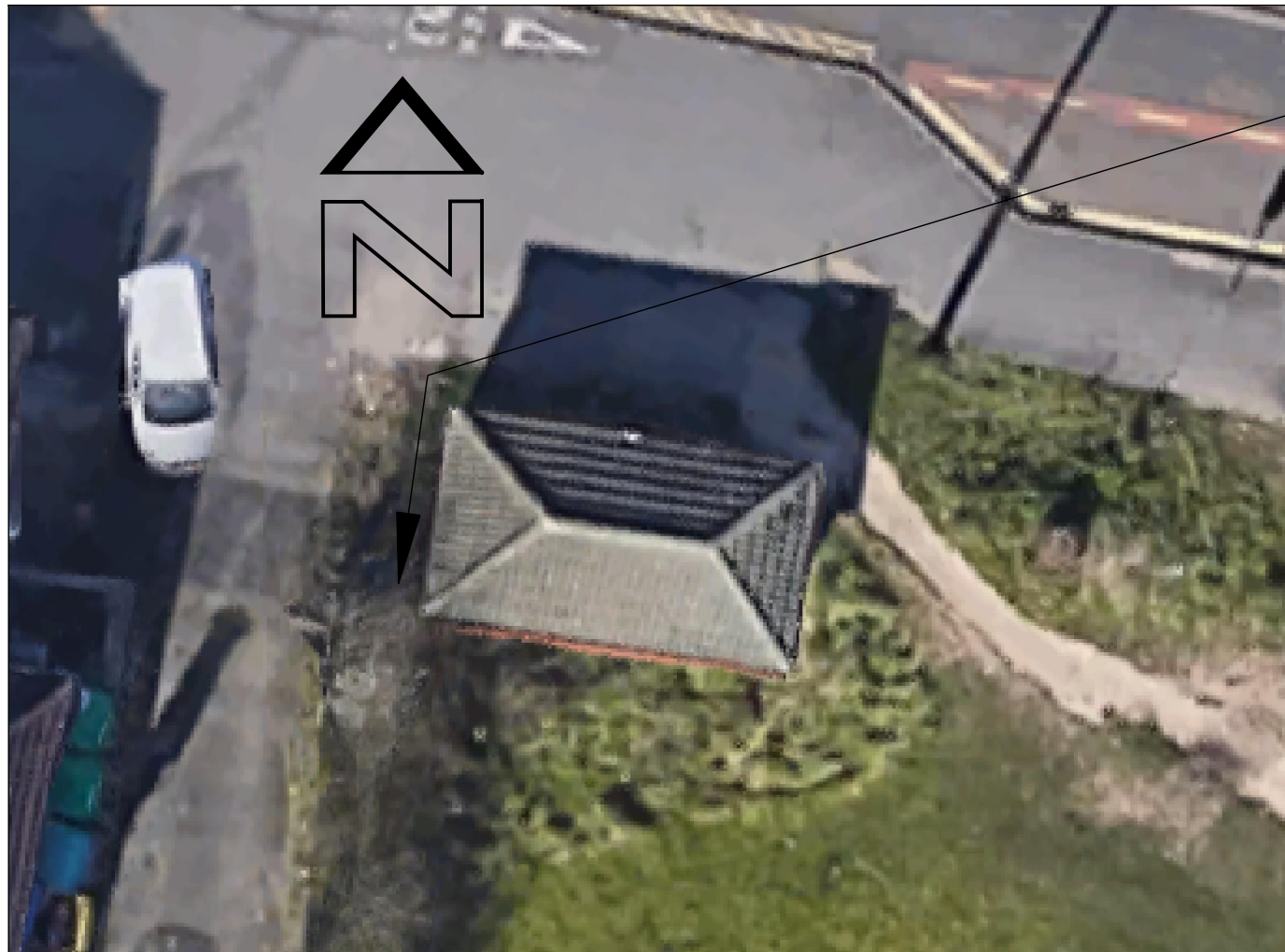
Existing Building in Location
