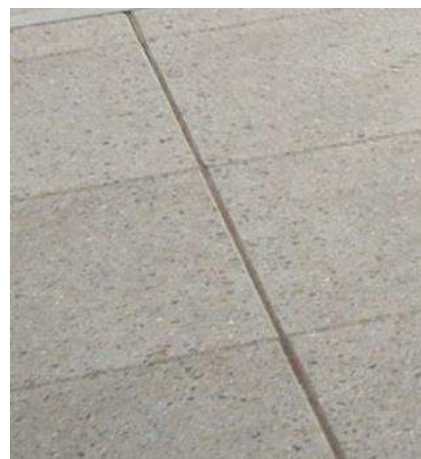
4 Paving: Concrete paving slabs Smooth concrete finish
