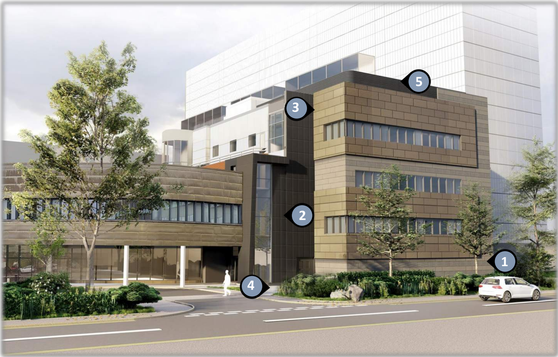
3 Feature Cladding: Brass rainscreen cladding system to match existing Oak Road facades
