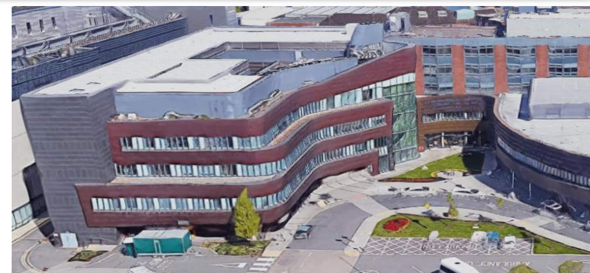
‘Bookend’ to Oak Road Treatment Centre to the West
