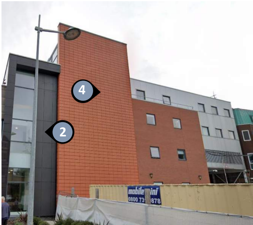
View of proposed extension location currently hidden by Cabins
