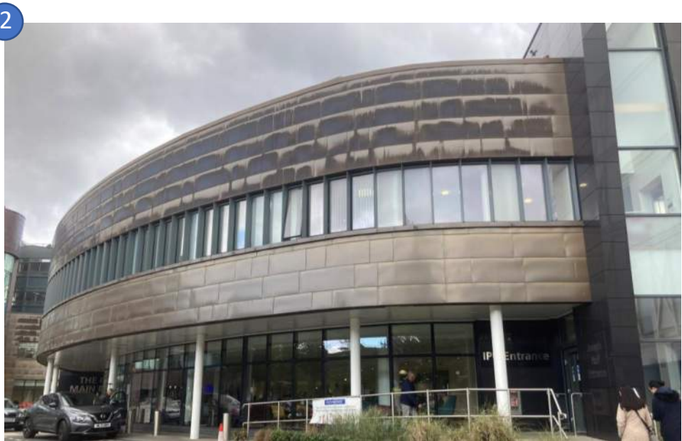
Photographed North-easterly view, highlighting the existing brass cladding along the Oak Road Entrance (note: brass affixed to the Oak Road Treatment Centre is also the same product but weathering alters the appearance as the buildings age)
