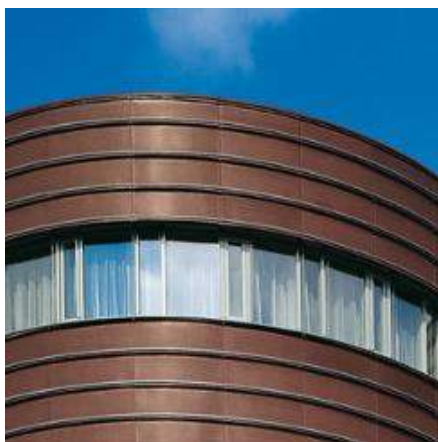
3 Feature Cladding: Brass rainscreen cladding system to match existing Oak Road facades
