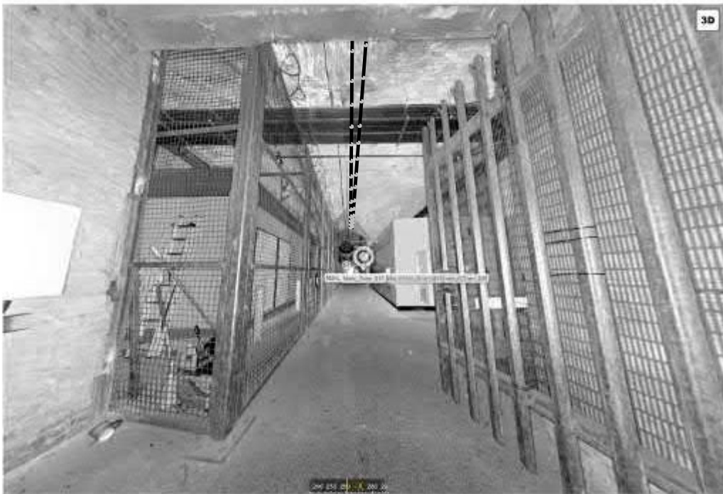
PHOTOGRAPH 05 CLEATED CABLES REACH GATEWAY
