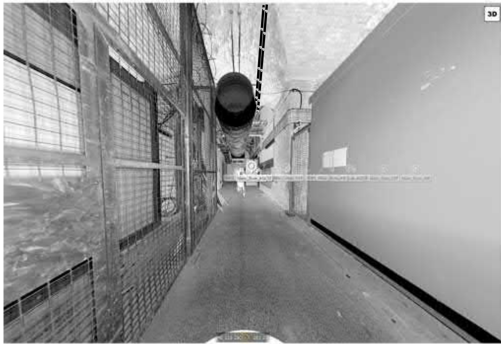
PHOTOGRAPH 03 CLEATED CABLES RUNNING ACROSS ROOF
