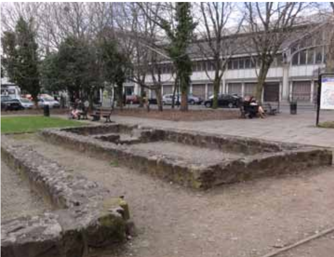
Figure 2.4: Representative building foundations of three Roman buildings have been reconstructed alongside the Roman Road
