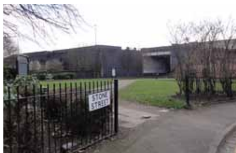
Figure 4.2: Pedestrian access into the site from Stone Street
