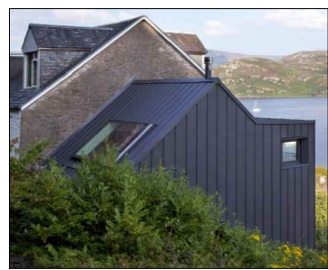
Anthracite (RAL 7016) standing seam zinc roof and wall cladding
