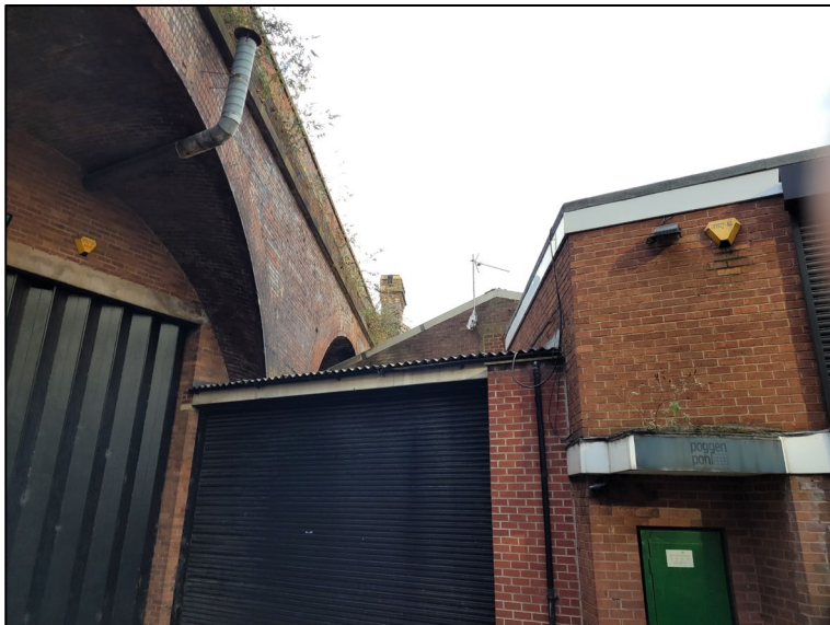
Photograph 3 Another view of the rear of the structures
