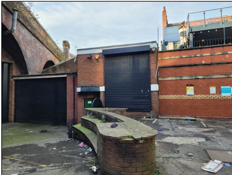
Photograph 2 The rear of the structures
