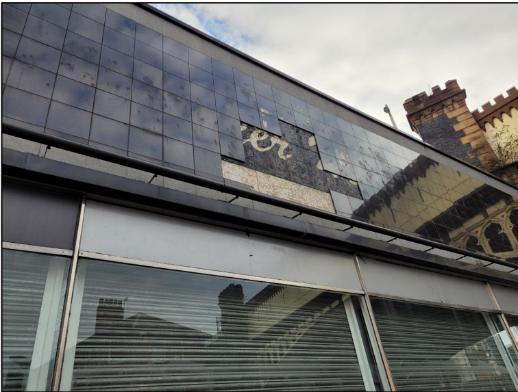
Photograph 5 Tiles removed at the front of the structure. No PRF present
