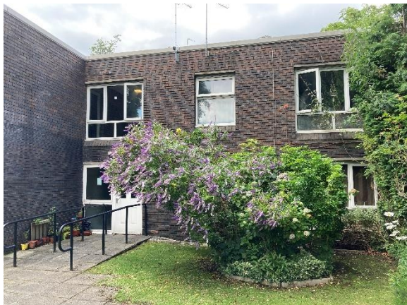
Fig 2.4: Rear annex taken from adjacent to rear boundary.
