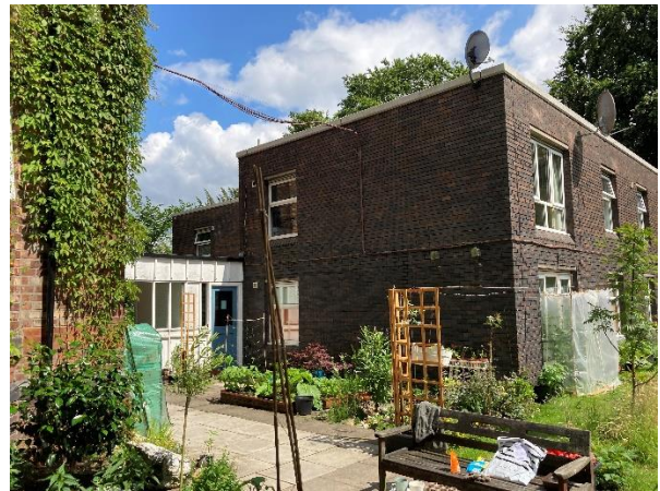
Fig 2.7: Rear annex building and small single storey link to villa.
