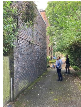
Fig 2.5: Access route running to side of property.
