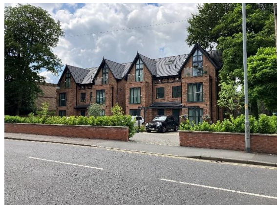
Fig 2.9: Modern development on the corner of Queenston Road and Palatine Road.
