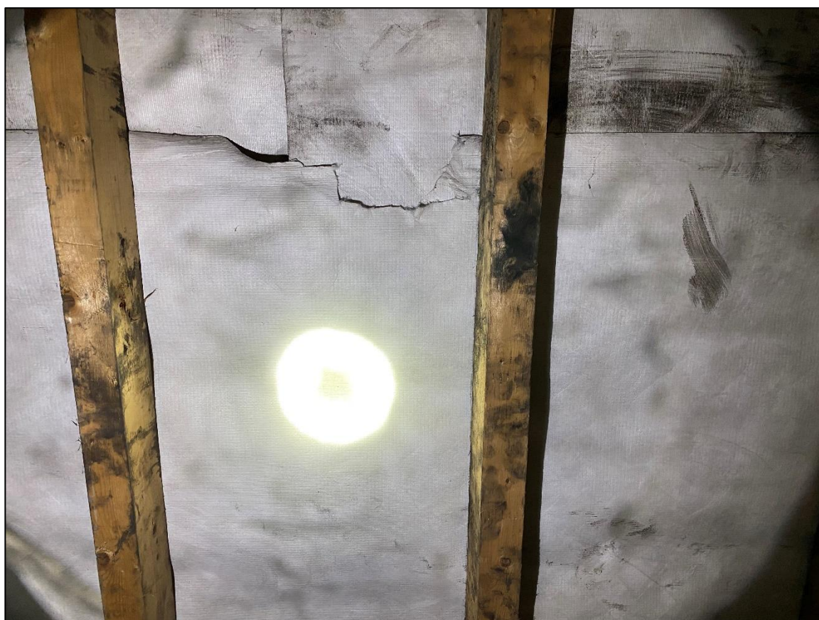
Plate 6 – Breathable roof membrane present beneath roofing materials
