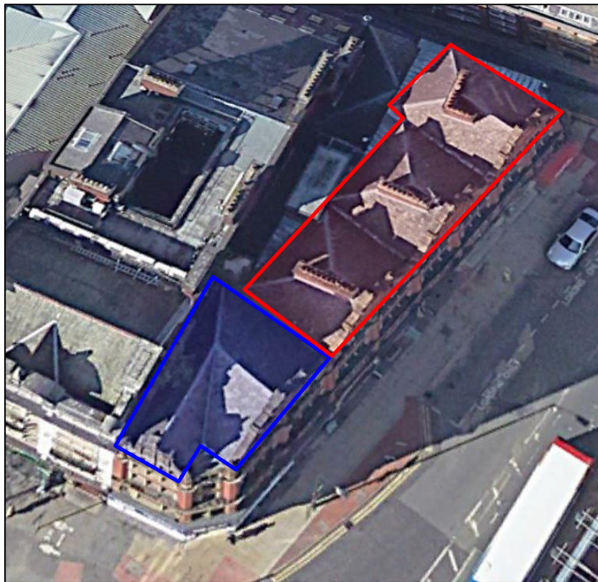
Figure 7.1 - Aerial view of the building indicating the accessed loft space in blue and inaccessible spaces in red
