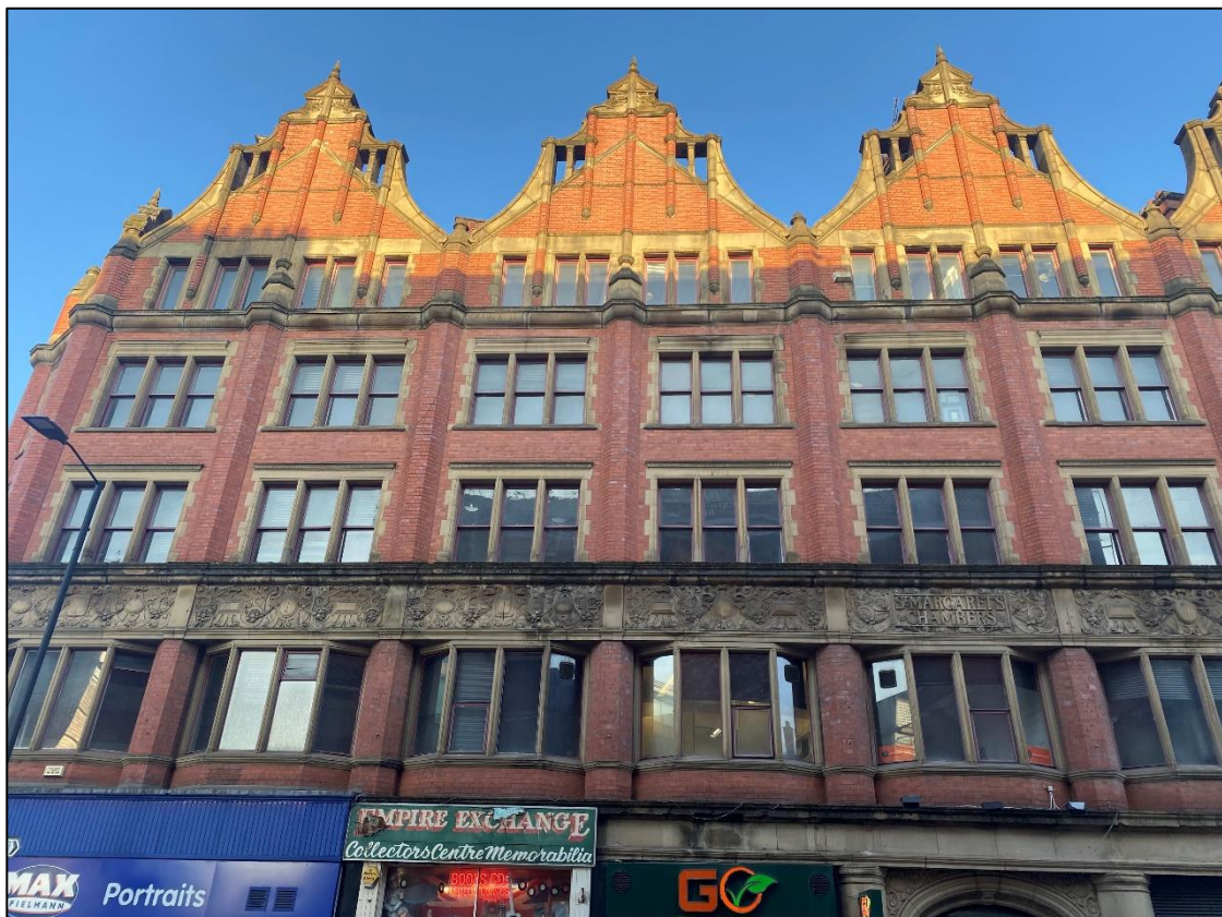
Plate 2 – South-eastern elevation of the building
