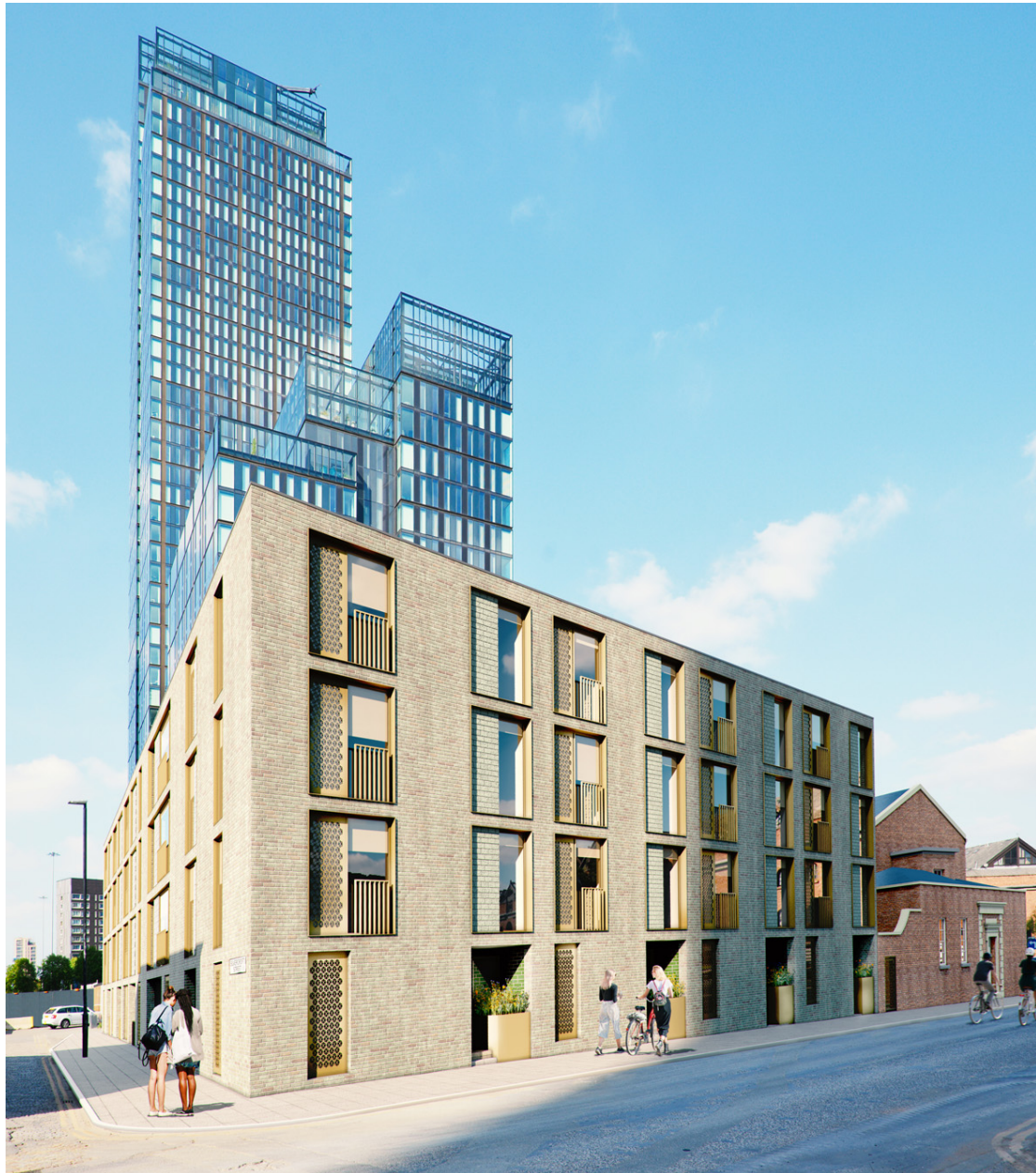
Figure 42 - The vibrant colours of the new build development
