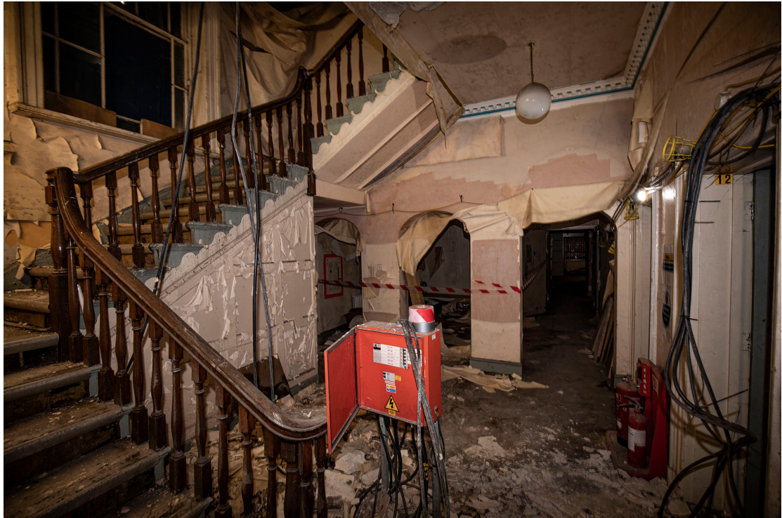
Figure 11 - The original staircase to the east house showing the 19 th century hardwood balustrade
