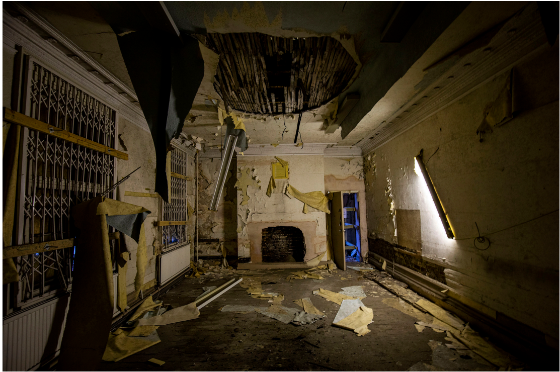
Figure 13 - Typical condition of a room (late 18 th century former dwelling - ground floor)
