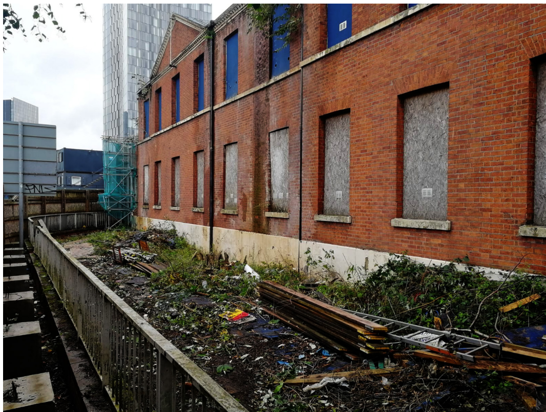
Figure 10 – North elevation of Bridgewater House (Chester Road) now cleared of overgrown vegetation
