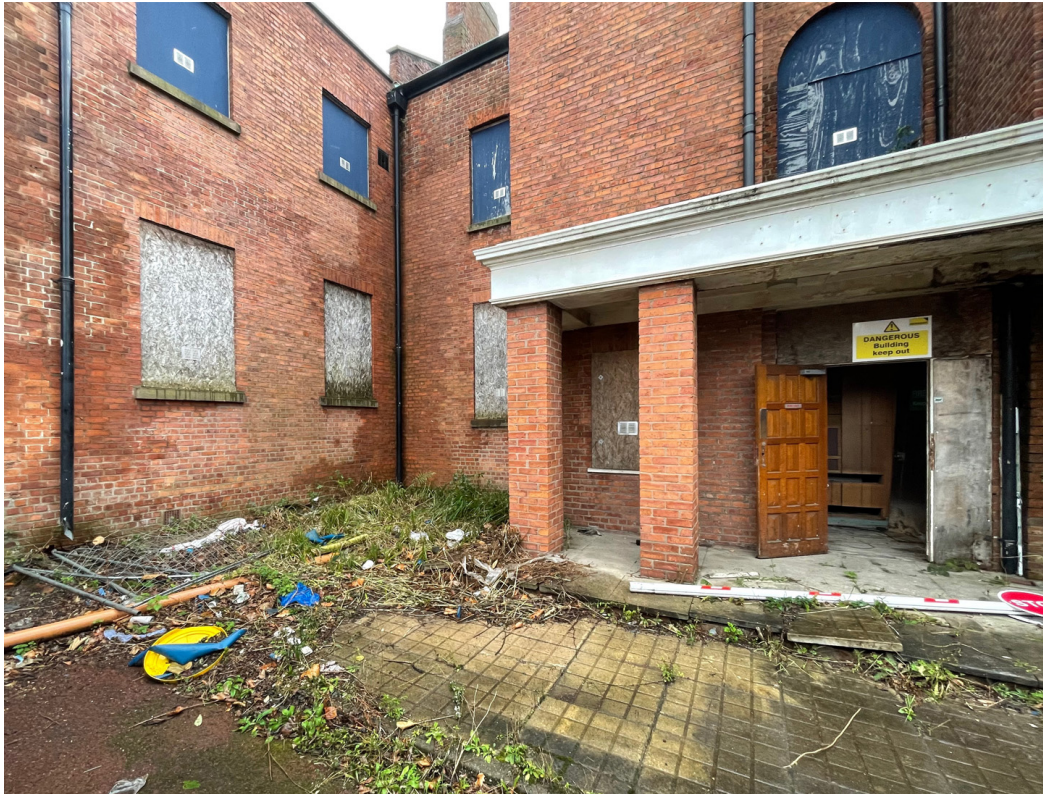
Figure 9 – South elevation of Bridgewater House (courtyard) now cleared of overgrown vegetation
