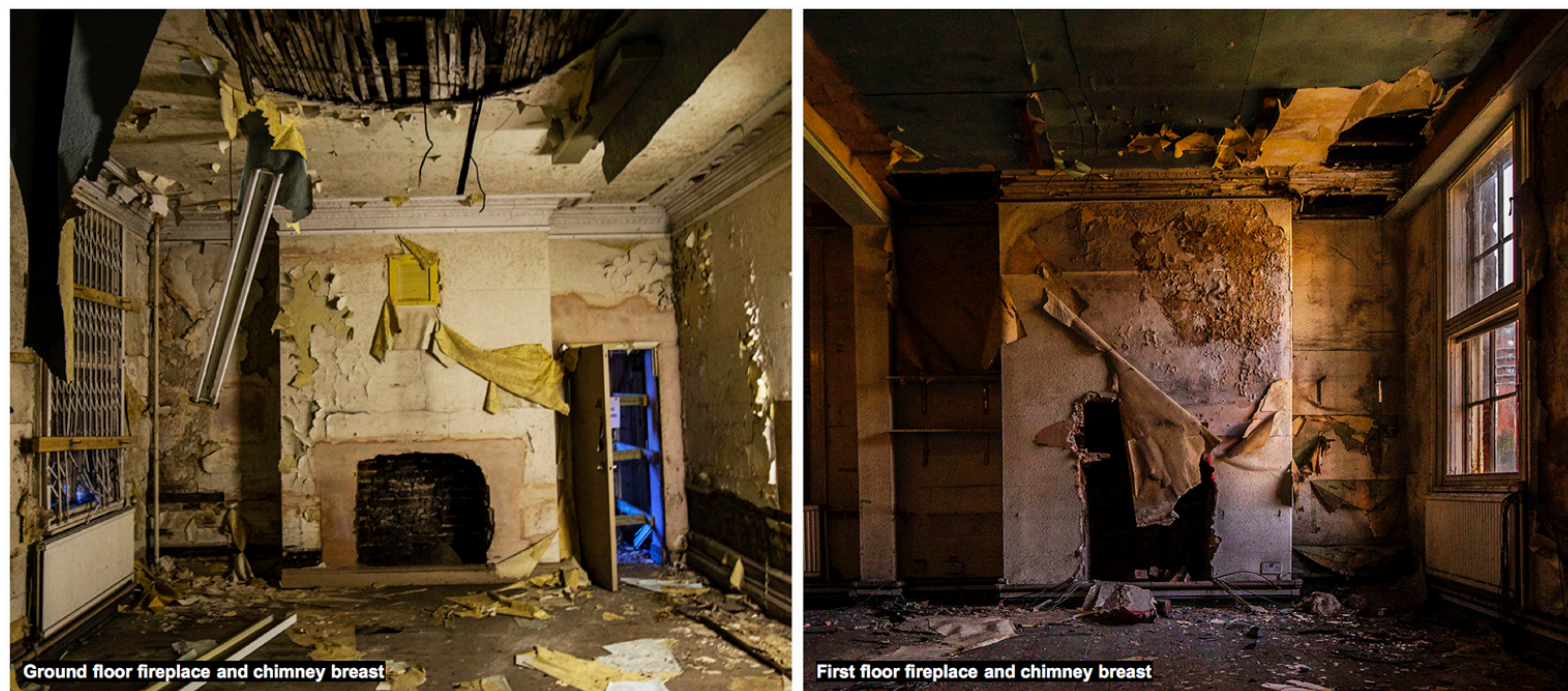
Figure 39 - Fireplaces and chimney breasts in Bridgewater House
