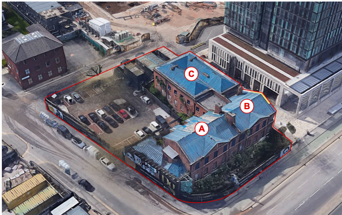
Figure 3 - View looking south across the Site (outlined in red)
