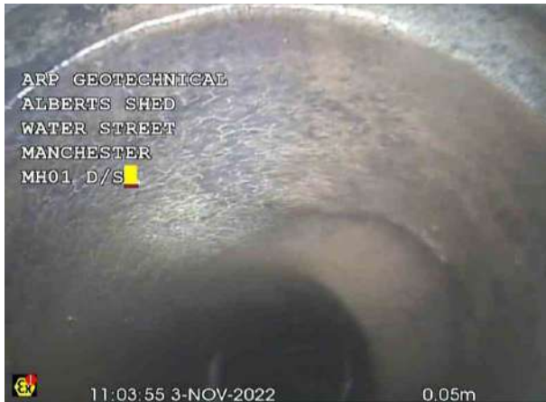
MH01X_ec86657f-0657-4975-9eda-e6d809d3f18a_20221103_111458_128.jpg, 00:00:01, 0.05 m Junction at 2 o'clock, 100mm dia
