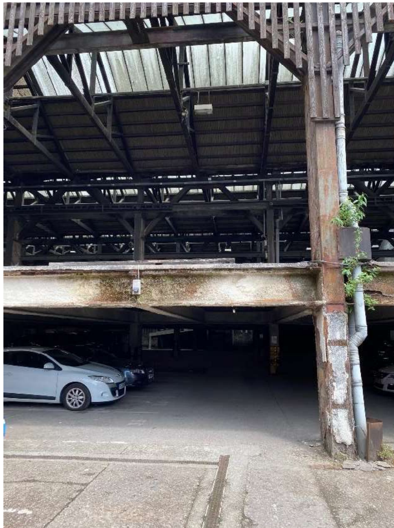
Photograph 3. View on southwest elevation, showing existing basement parking level, existing Ground Floor level and interior of roof.
