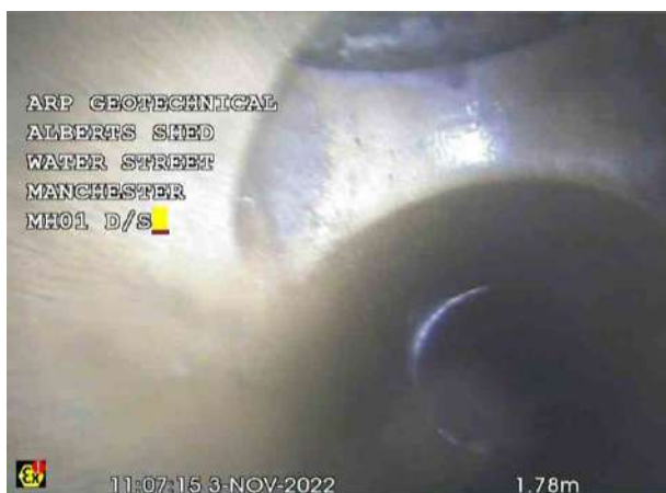
MH01X_73f03247-50e8-4c4d-a11c-fd4f8848867a_20221103_111802_241.jpg, 00:00:09, 1.78 m Junction at 11 o'clock, 100mm dia
