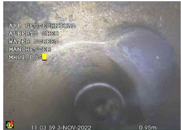
MH01X_7edd5d05-614e-4d4e-a7f7-91b04670f24d_20221103_111518_598.jpg, 00:00:04, 0.95 m Junction at 2 o'clock, 100mm dia
