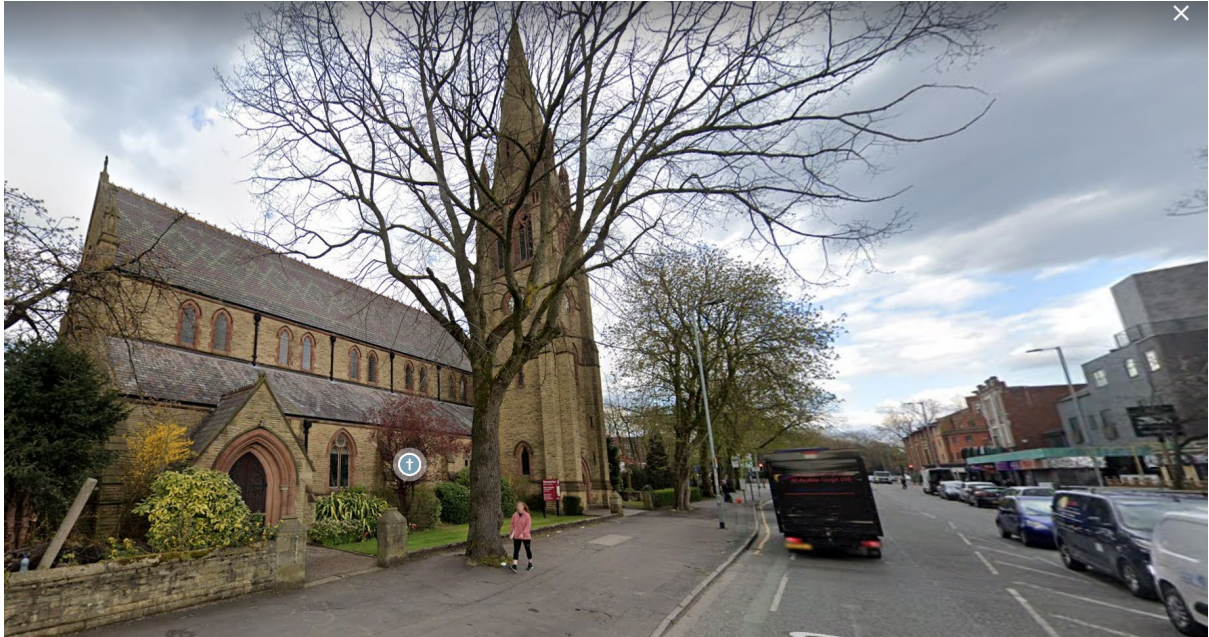
Church when viewed from Wilbraham Road.
