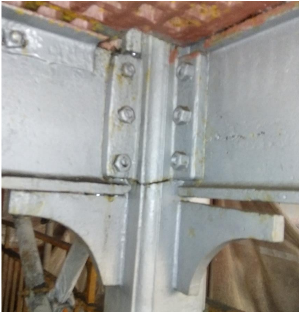
Column cracking
