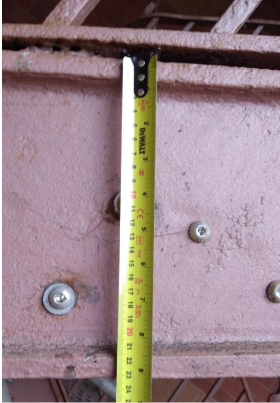
Stair stringers (supporting handrails)
