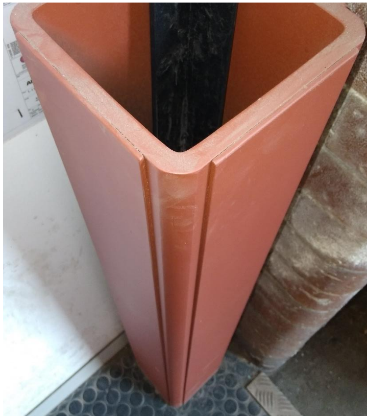
Example of replacement mild steel column
