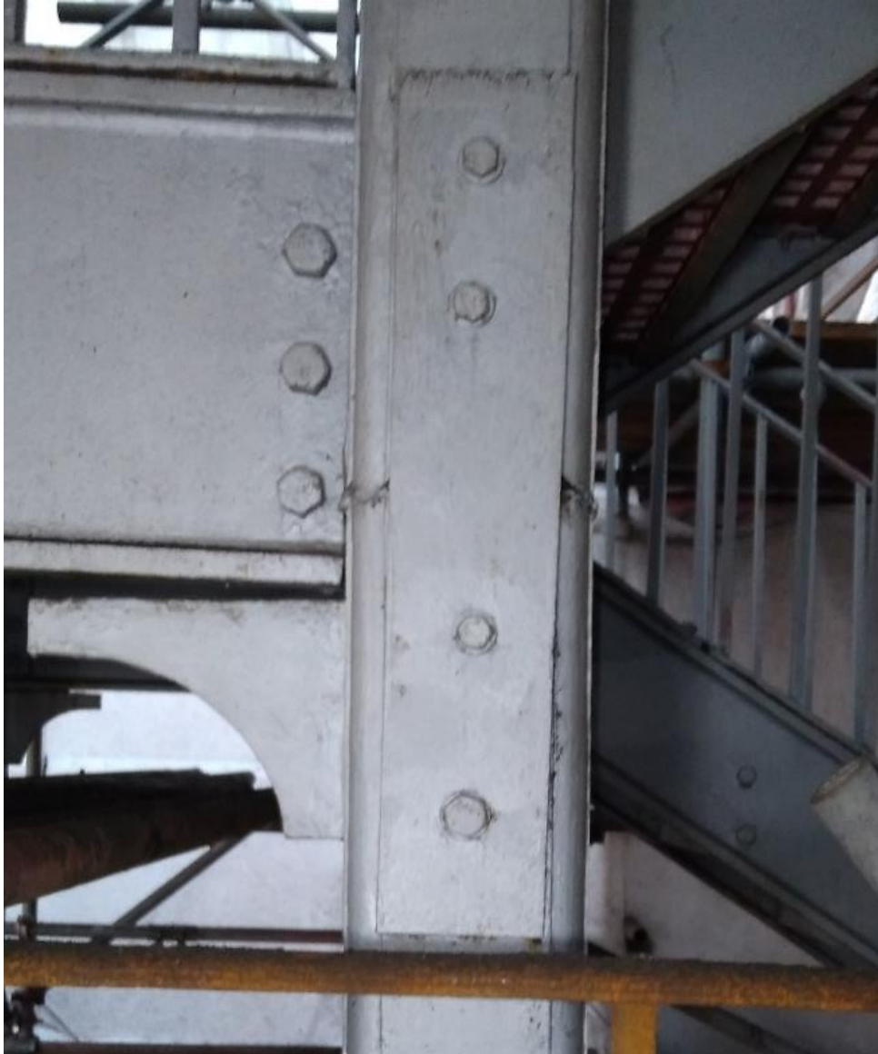
Historic bolted splice (to 1 face only).
