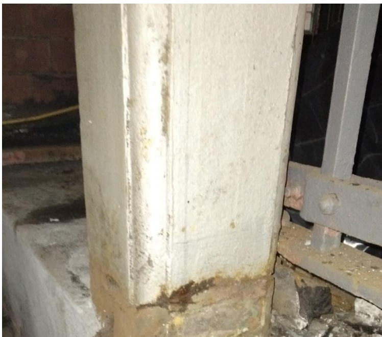
Iron columns with bevelled corners.
