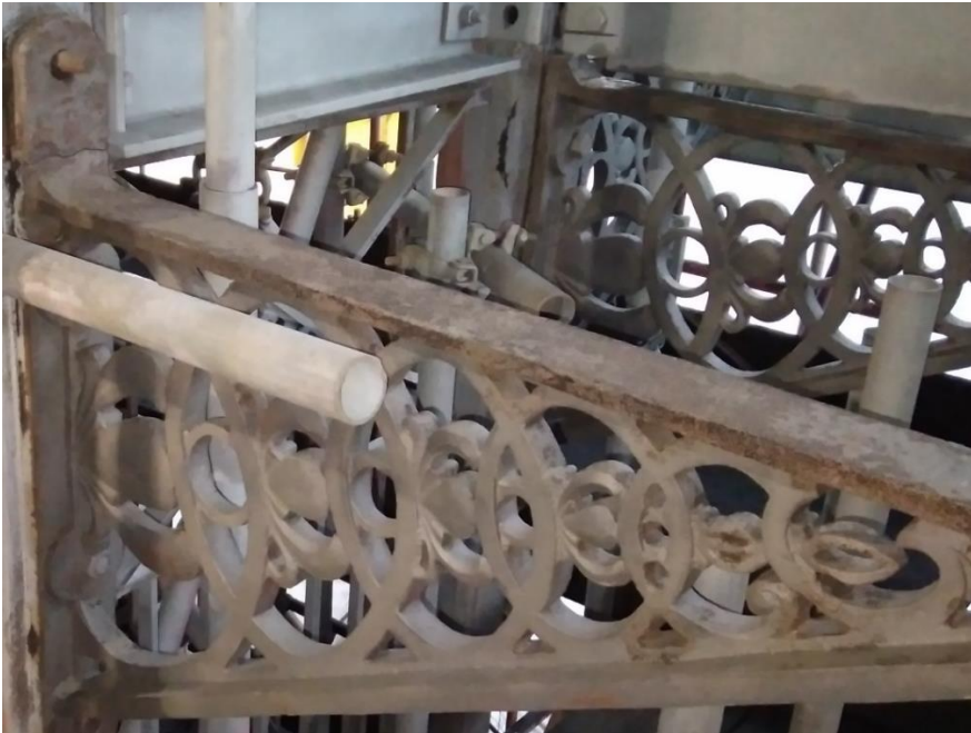
Existing Cast-iron spandrel
