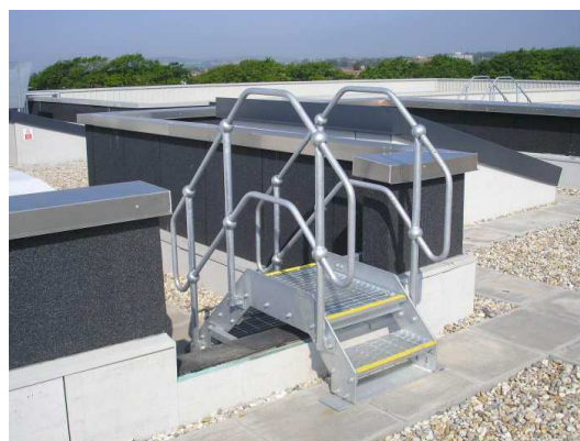
3. Steel access stair
