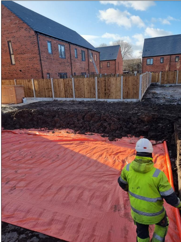
Photographs 7-9: Reduced level dig and high-visibility membrane installation within rear gardens of plots 14-17.
