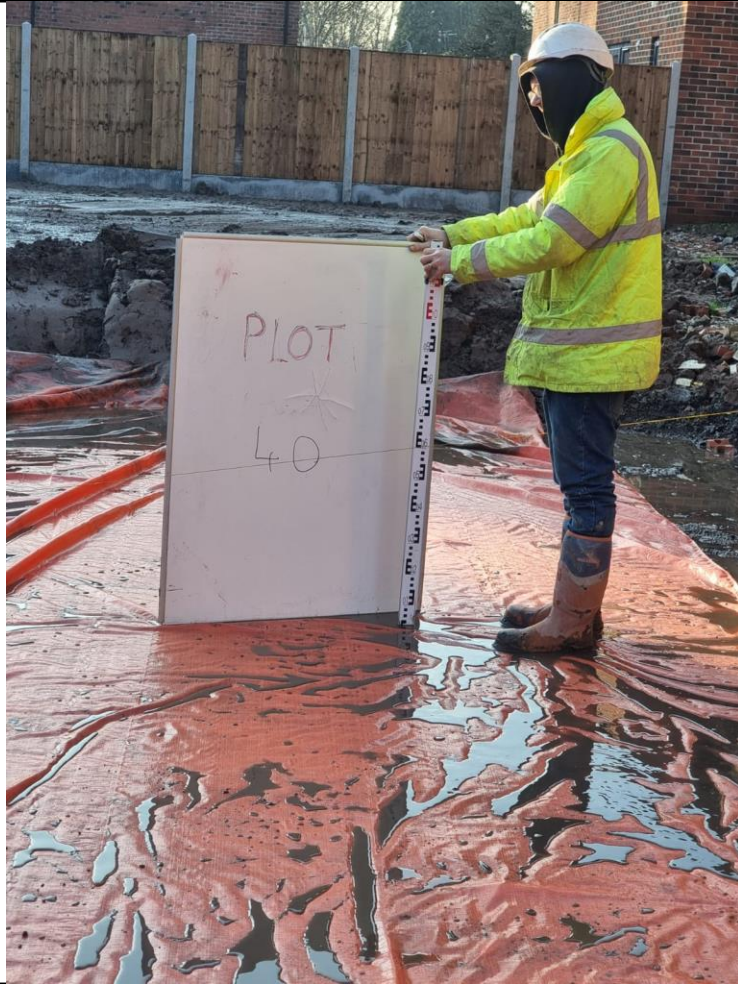
Photograph 5: Reduced level dig and high-visibility membrane installation within rear garden of plot 40.
