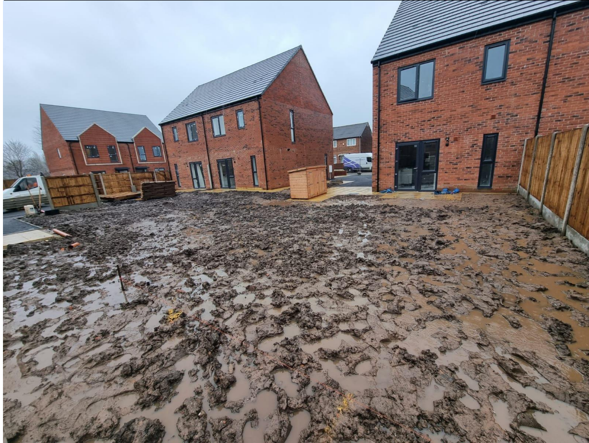
Photograph 5: Finished rear garden area of plots 15-17.
