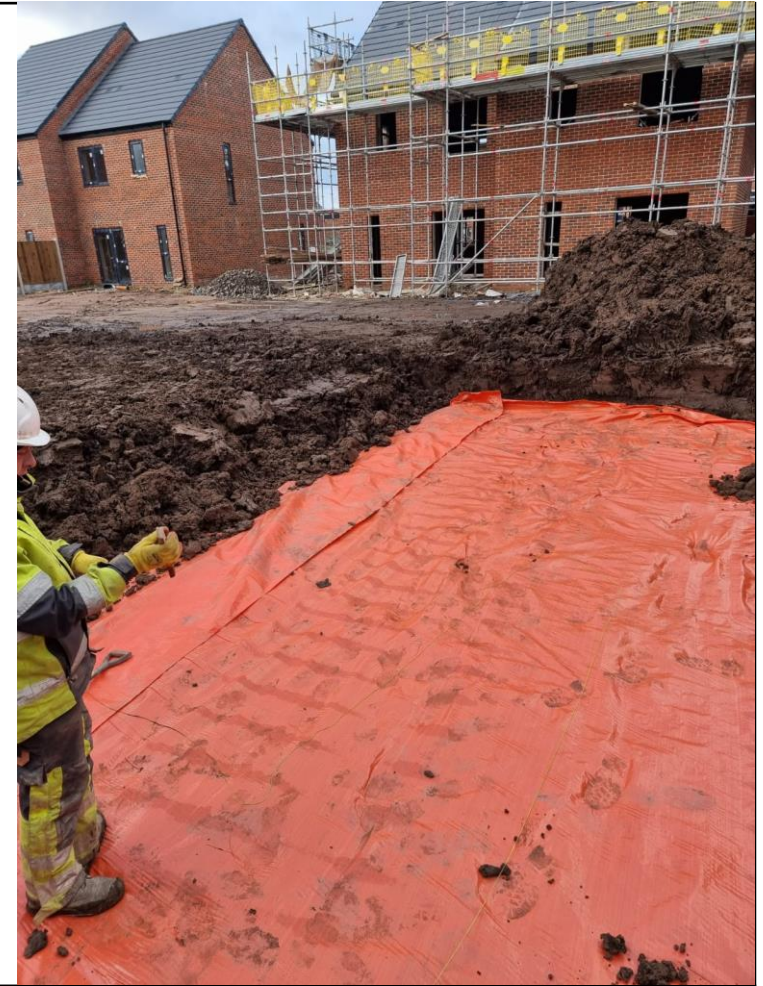
Photographs 7-9: Reduced level dig and high-visibility membrane installation within rear gardens of plots 14-17.
