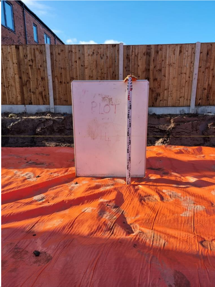
Photograph 1: Reduced level dig and high-visibility membrane installation within rear garden of plot 14.
