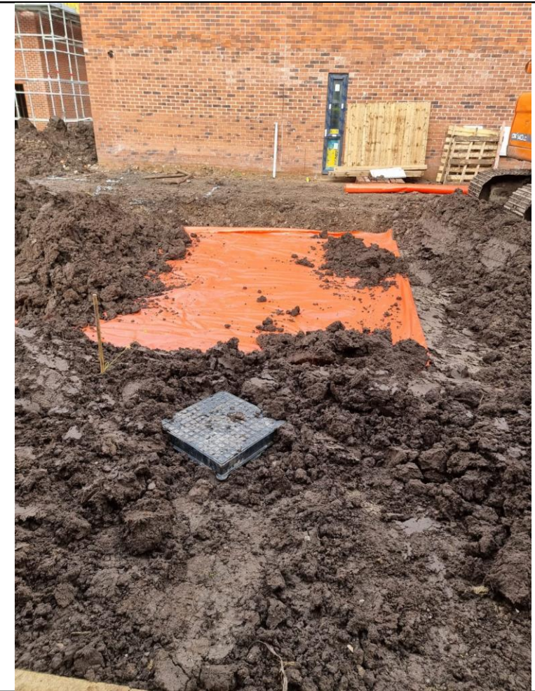
Photographs 10 and 11: Reduced level dig and high-visibility membrane installation within rear gardens of plots 14-17.
