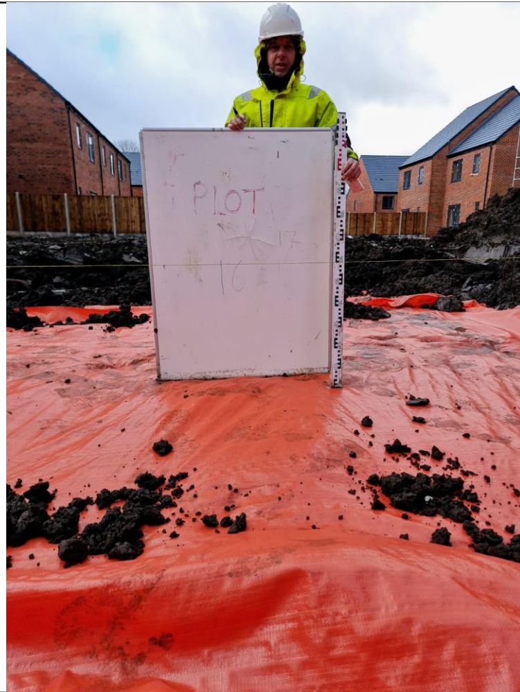
Photograph 3: Reduced level dig and high-visibility membrane installation within rear garden of plot 16.
