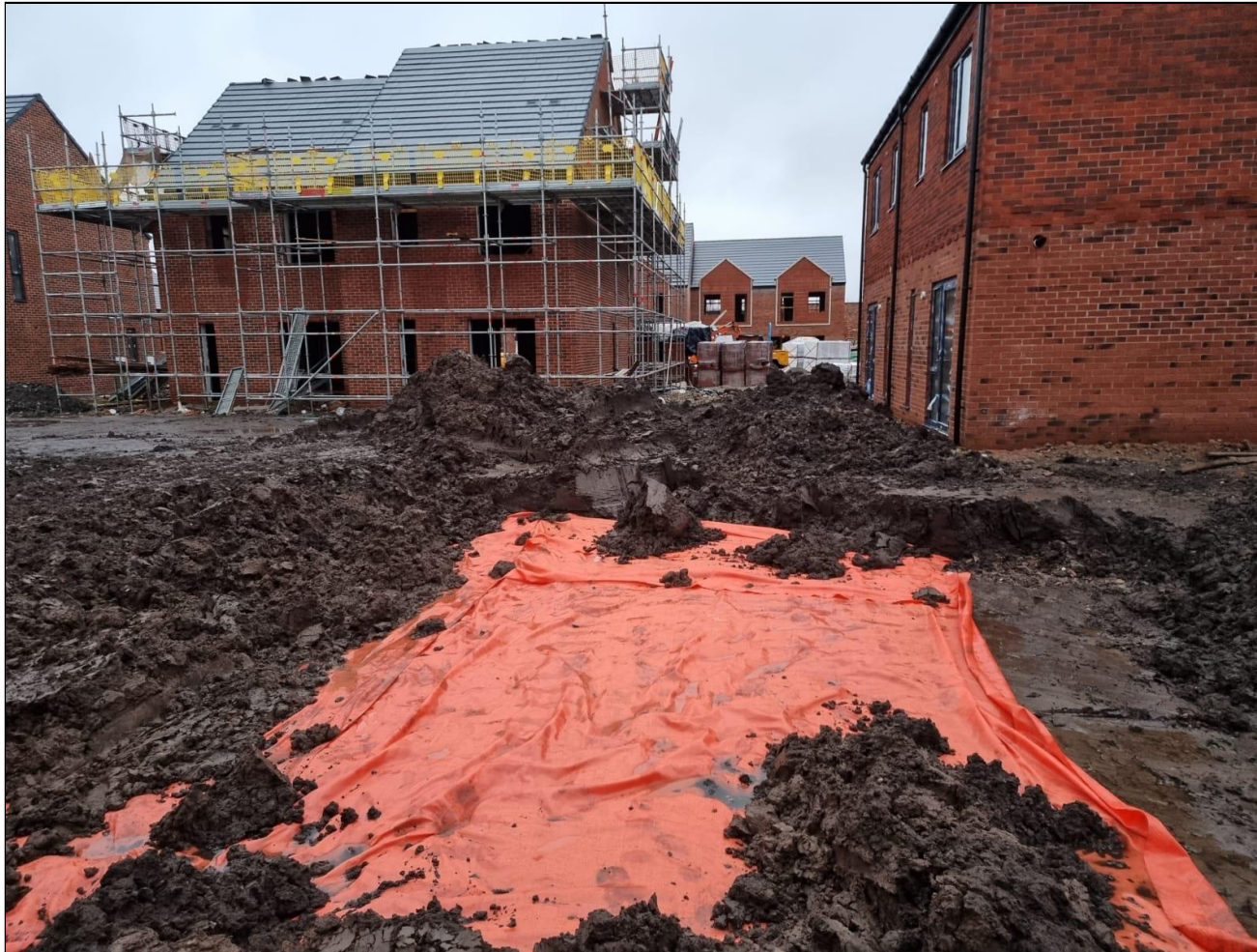
Photographs 10 and 11: Reduced level dig and high-visibility membrane installation within rear gardens of plots 14-17.
