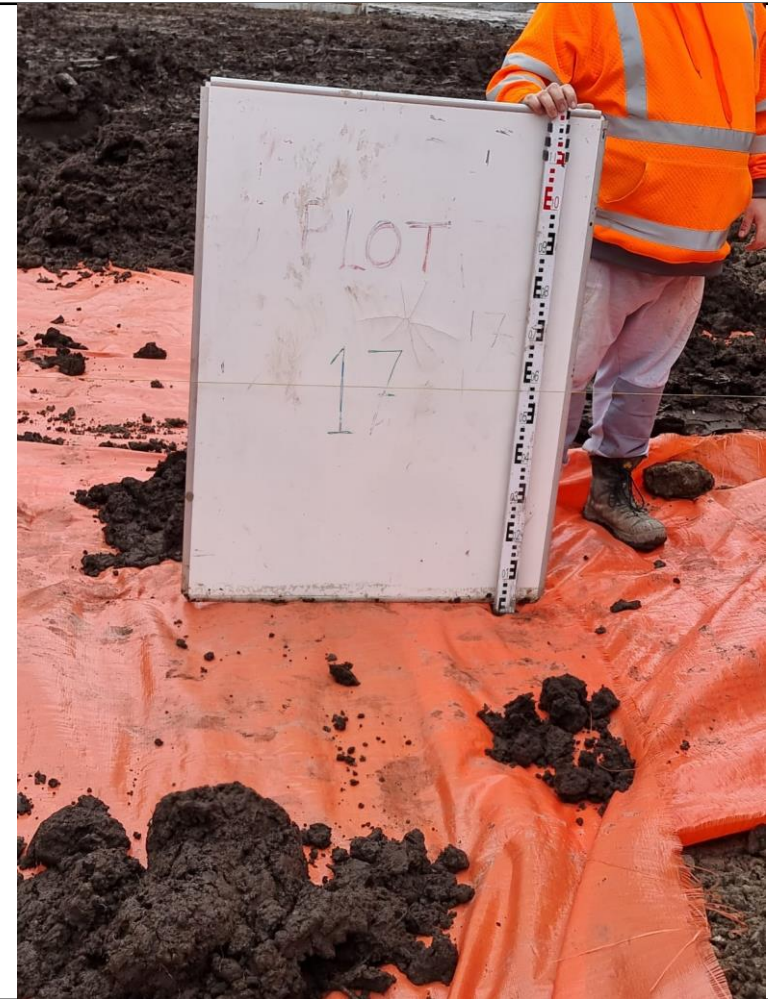
Photograph 3: Reduced level dig and high-visibility membrane installation within rear garden of plot 16.
