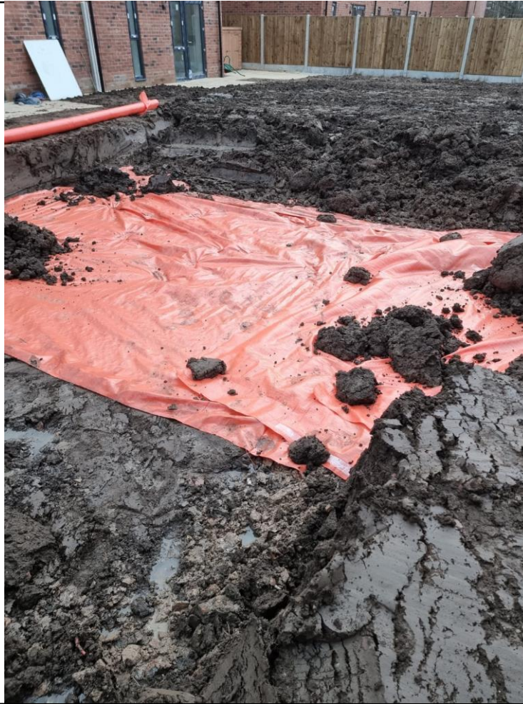
Photographs 7-9: Reduced level dig and high-visibility membrane installation within rear gardens of plots 14-17.
