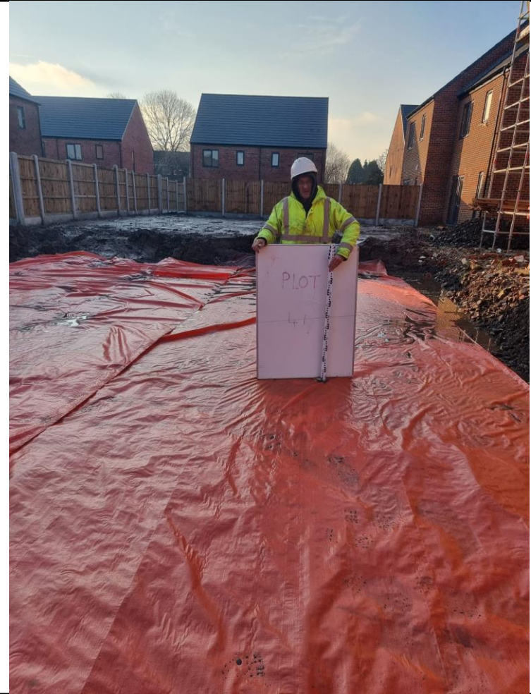
Photograph 5: Reduced level dig and high-visibility membrane installation within rear garden of plot 40.
