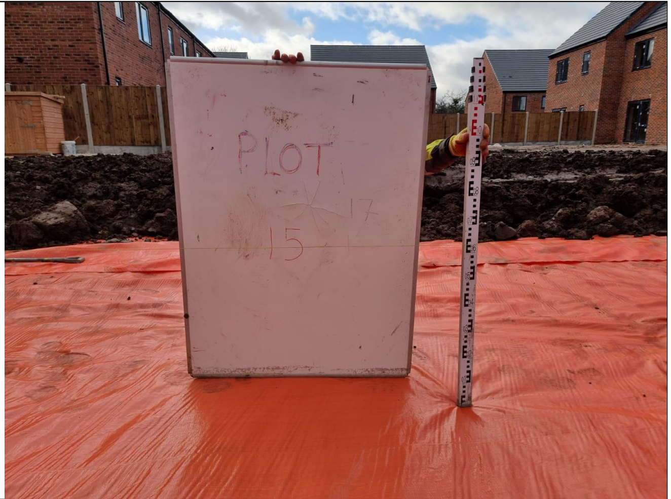
Photograph 1: Reduced level dig and high-visibility membrane installation within rear garden of plot 14.
