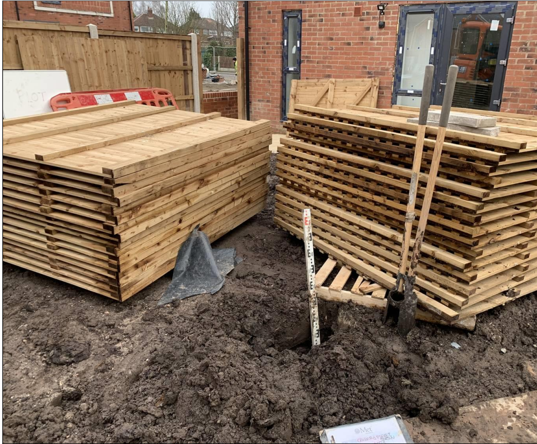
Photograph 19: Hand Dug Pit Topsoil Depth Validation – HDP14, Plot 16
