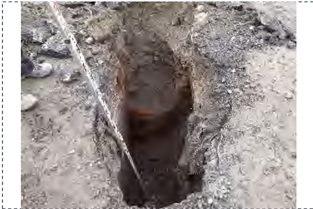
TP103 – West Facing View
