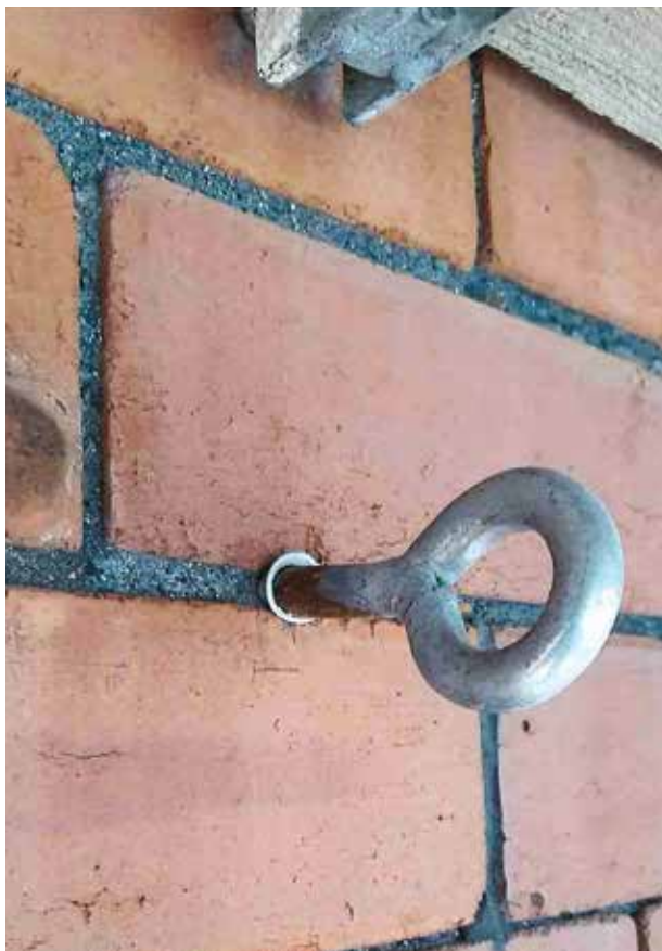
Image of system in use on listed building, (above) the narrow walkway close to the building, and (below) self tapping anchor eye-bolt fixed through mortar as a reversible fixing
