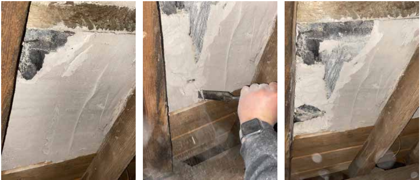
Example images of carefully tapping away to remove torching from a previous damaged area of torching.
