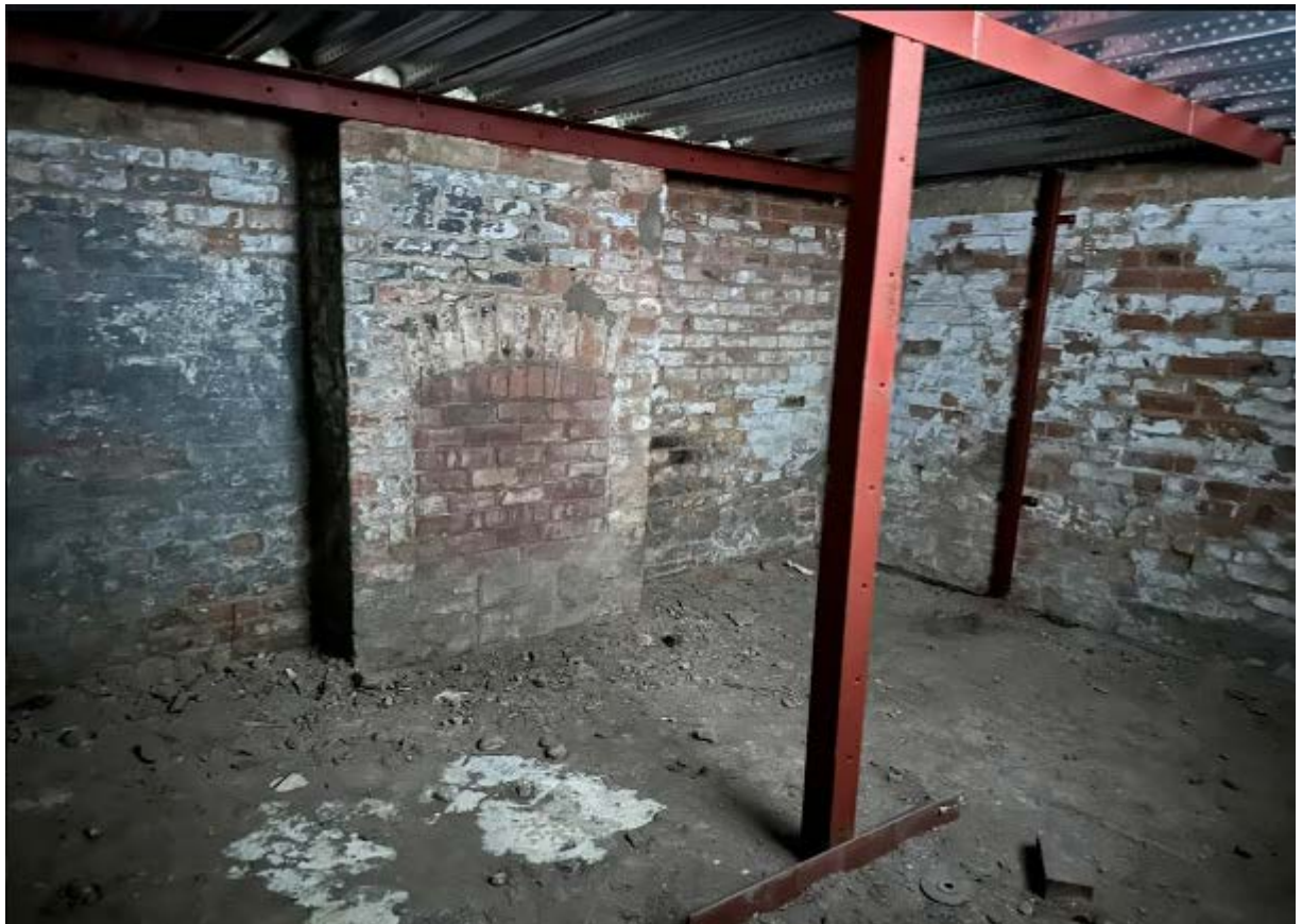
6. Room on the right of the basement
