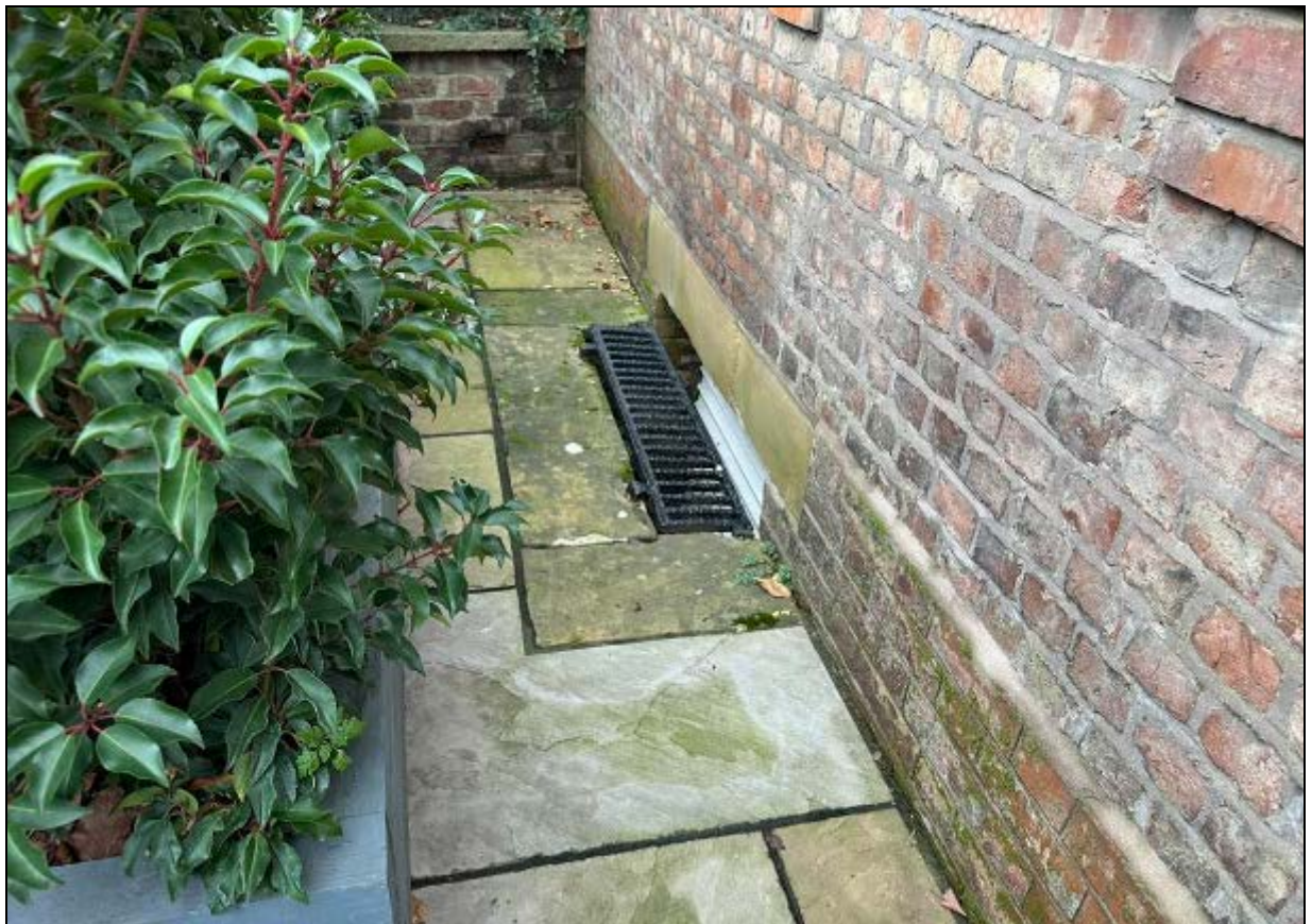
11. Similar lightwell to left basement room
