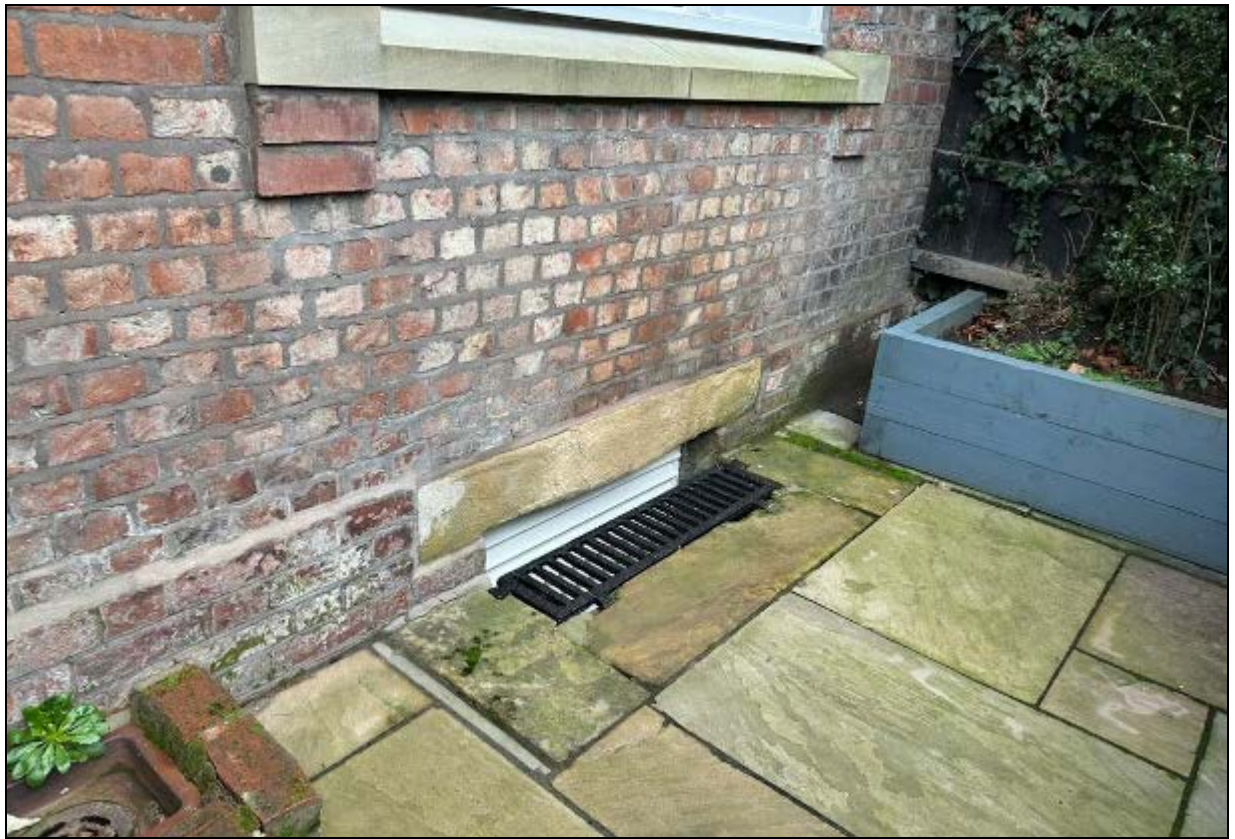
10. Paved over lightwell to right basement room
