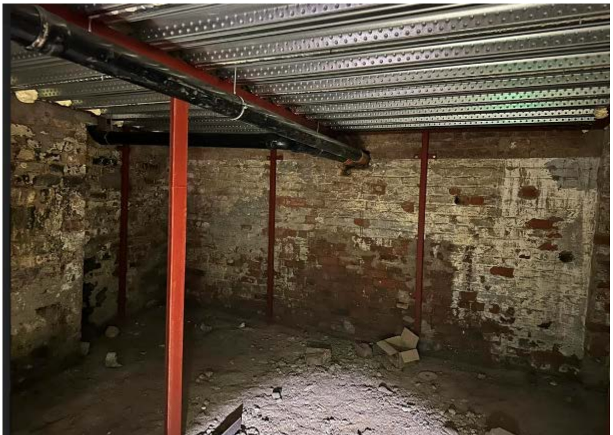
7. Room on the left side of the basement
