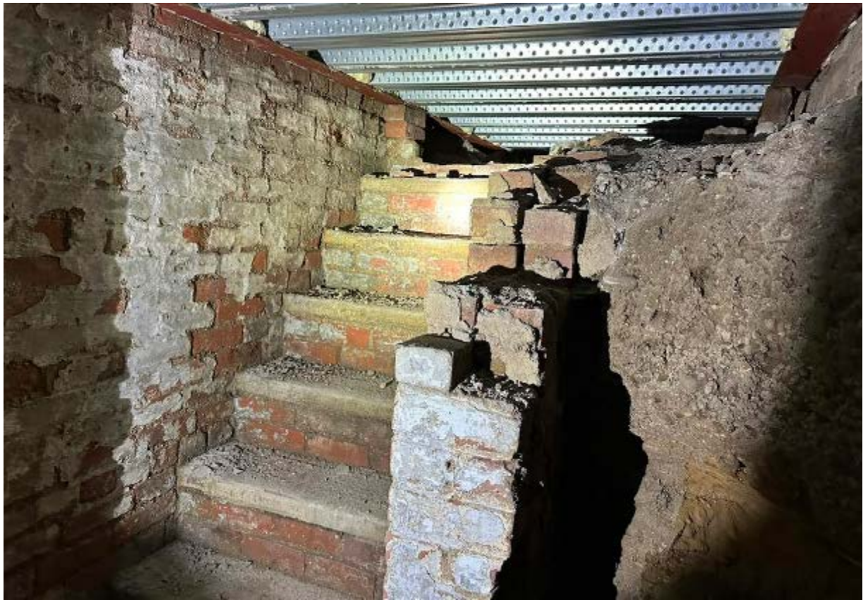
8. Remnant of original steps to ground floor
