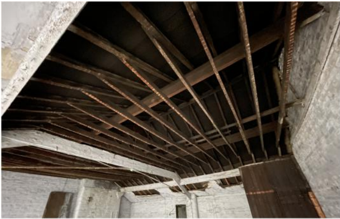
Existing 400 x 240mm primary timber beam
