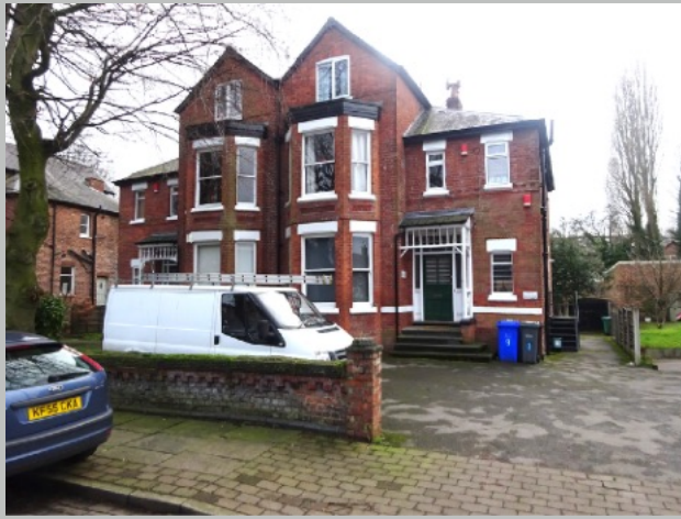
Plate 17. Front of No. 9-11
