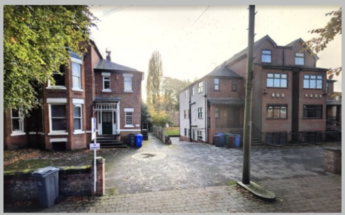
Plate 12 Accesses to 9 and 11 Vincent Avenue
