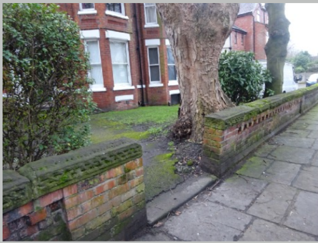
Plate 15. Brick-panelled front boundary wall with stone coping
