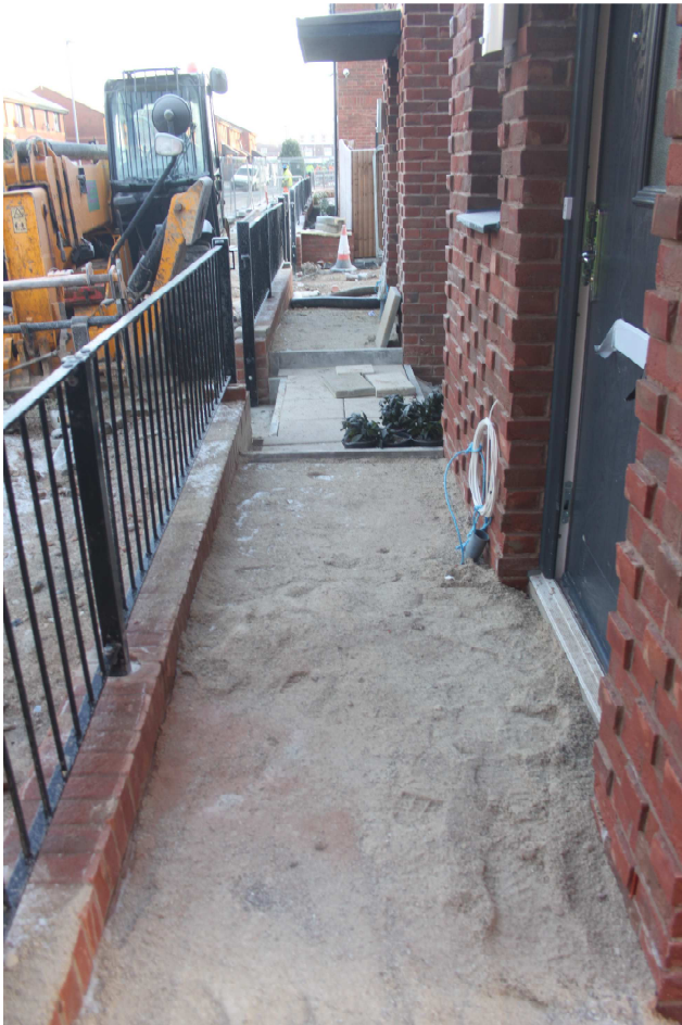
Block 1 – plots 1 and 2 – back of footpath
