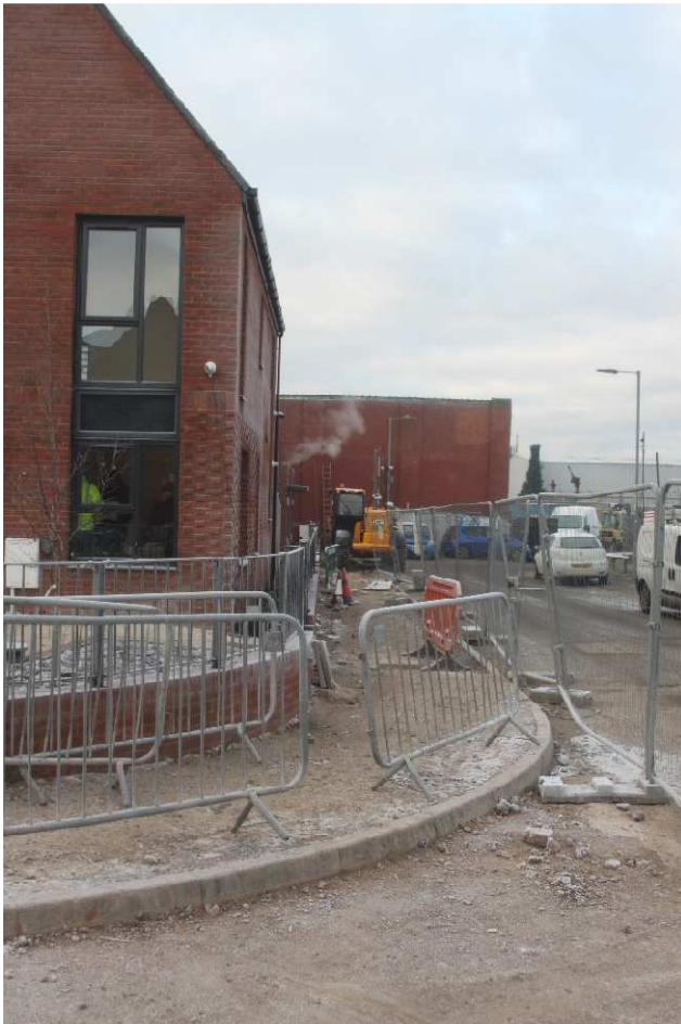
Block 1 – plot 3 – back of footpath
