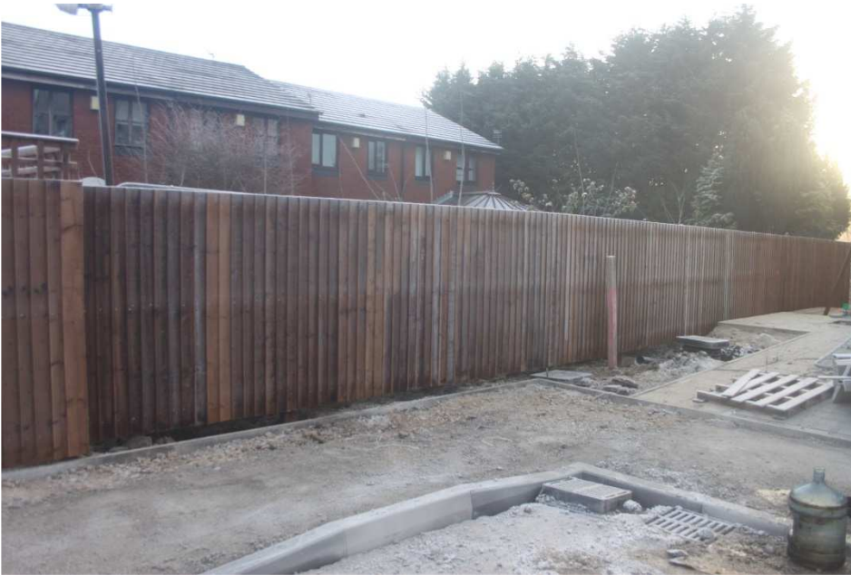
Boundary adjacent to Block 3 plot 21 and rear of no's 46, 48, 50 and 52 Dob Brook Close.
