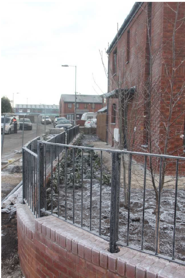
Block 4 – Plot 24 – back of footpath
