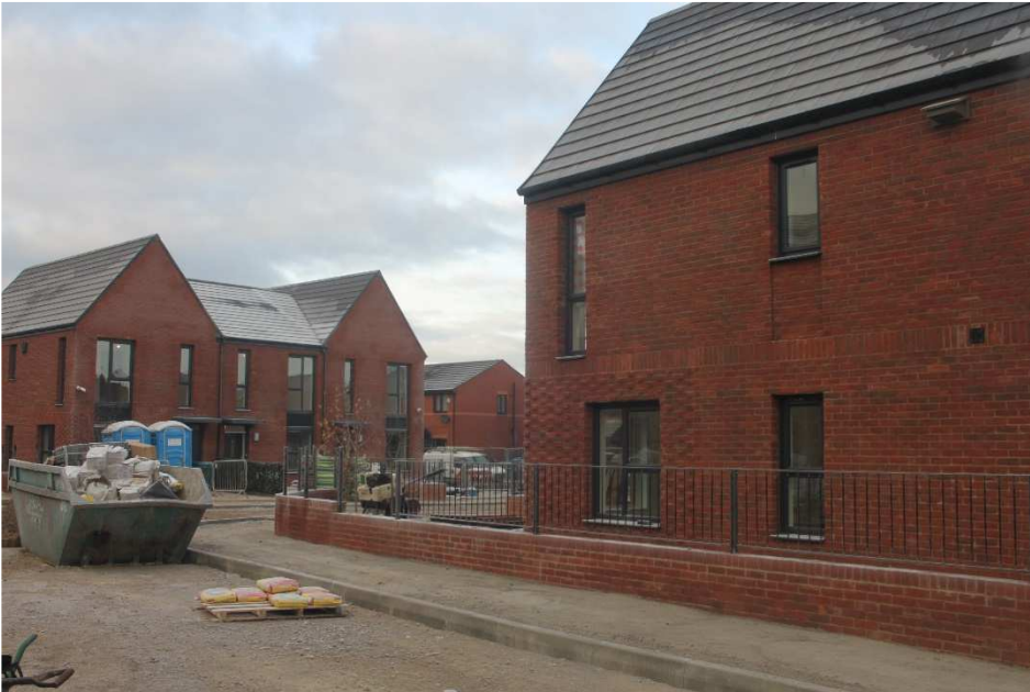
Block 2 – plot 3 – back of footpath
