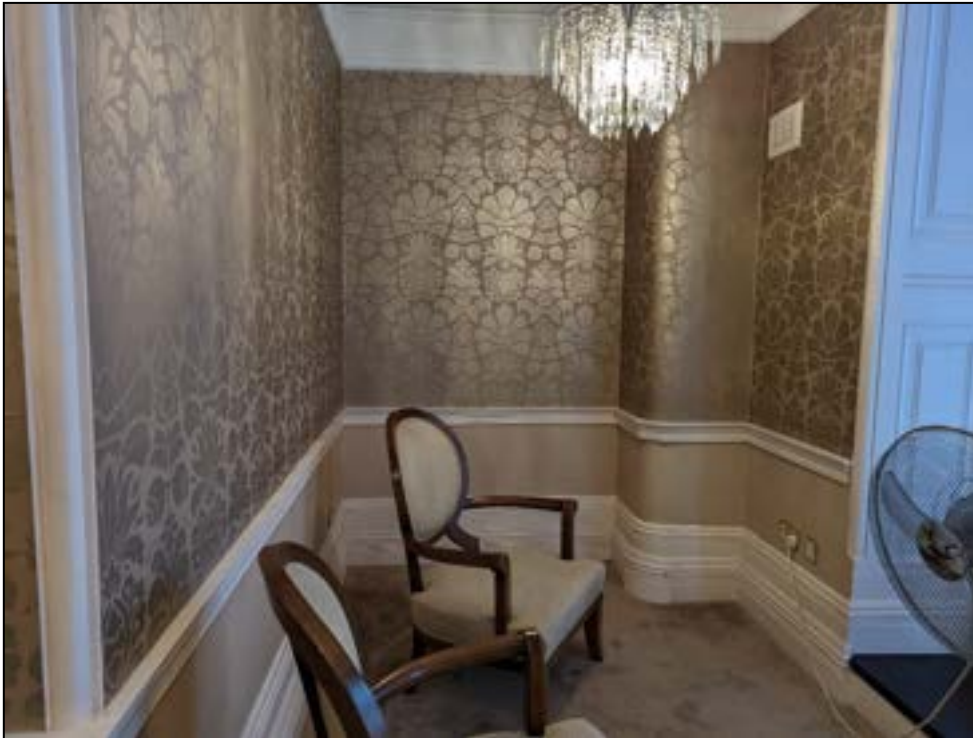
Plate 63: Stud wall to be removed (item 8)
