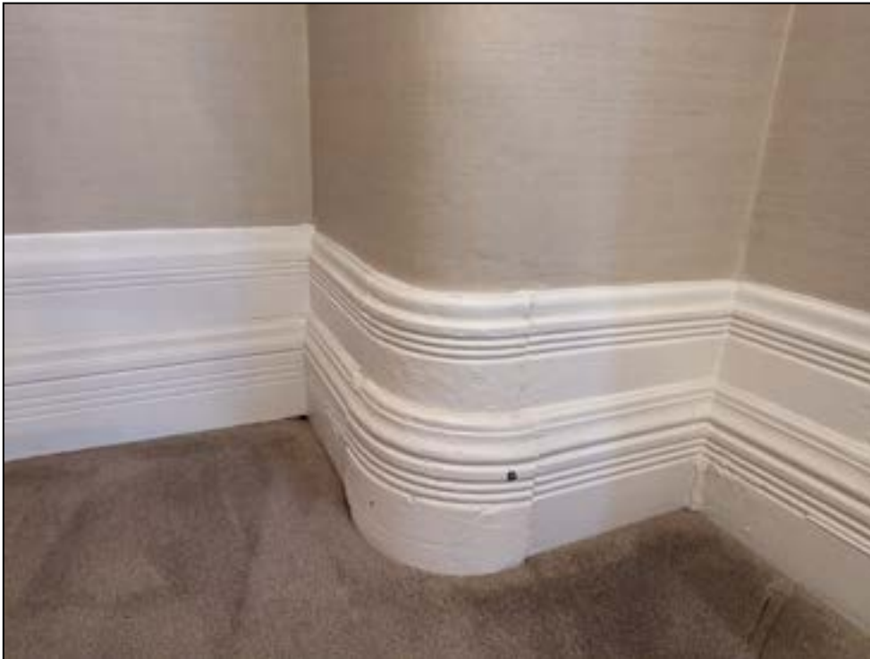
Plate 62: Wall to be removed (item 8) to the left showing skirting modern and original skirting
