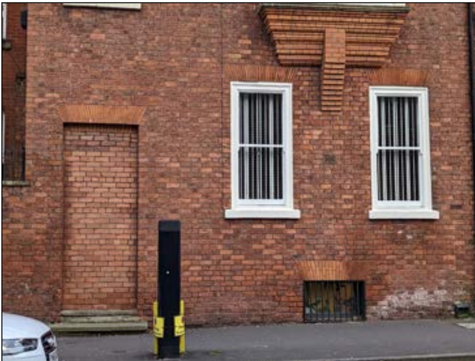
Plate 8: blocked doorway (item 1) and windows at ground floor level
