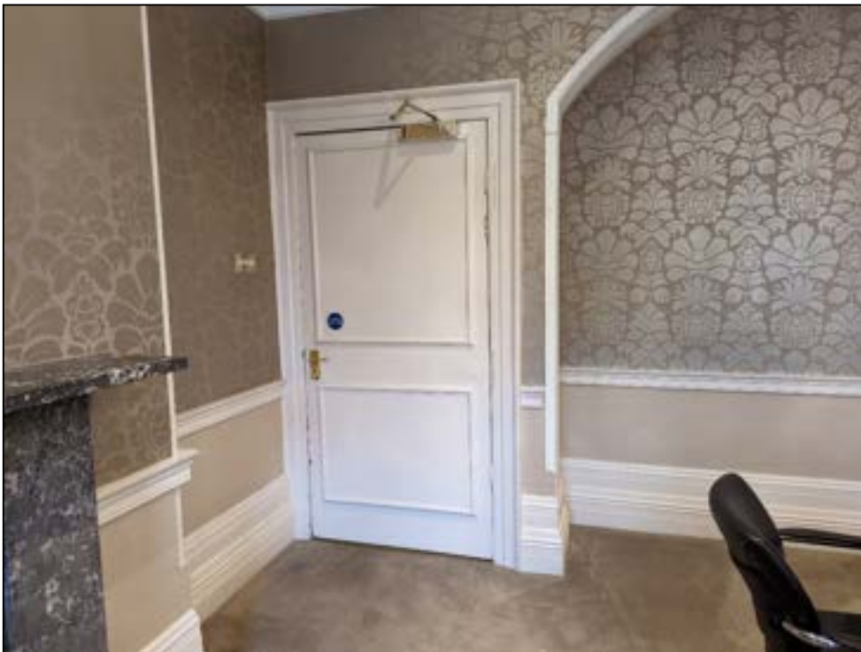
Plate 60: Flanking doorway in inserted wall
