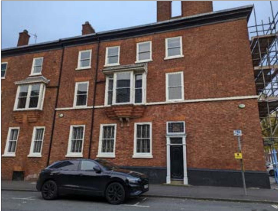
Plate 11: Southern end of west elevation of 28 St John Street
