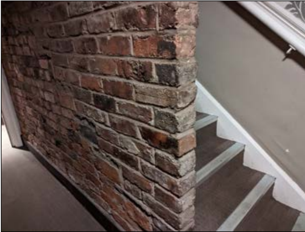
Plate 37: Staircase wall (item 3) showing ghost of former treds and rebuild above
