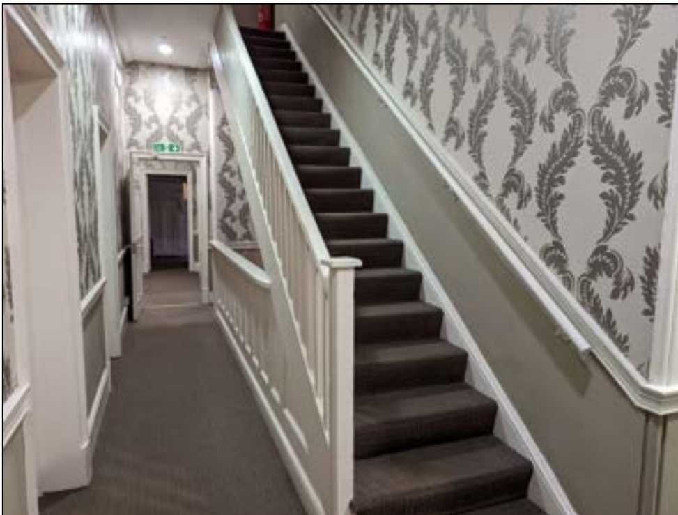
Plate 32: Simple staircase to first floor
