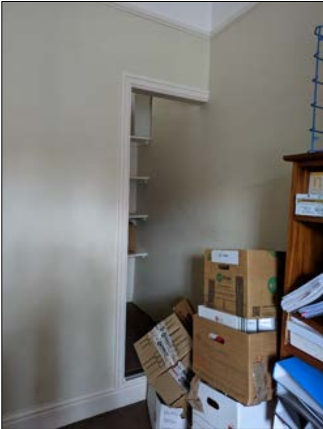
Plate 20: Inserted wall to the north
