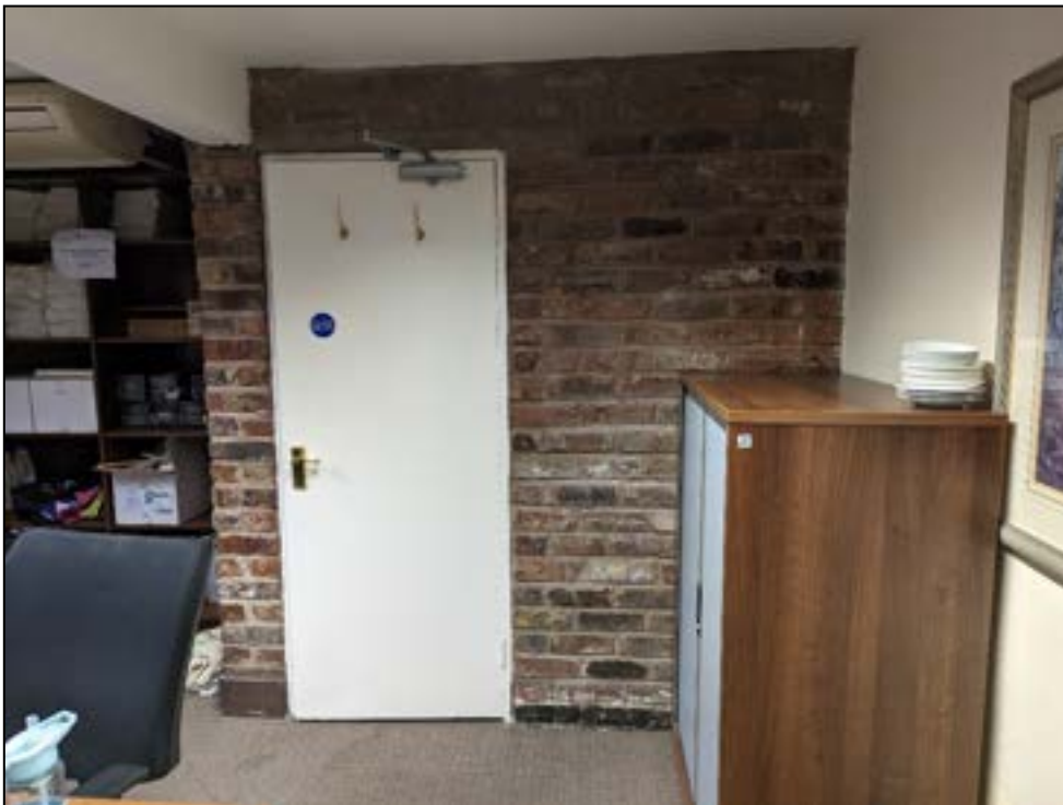
Plate 40: Wall to be removed (item 4)
