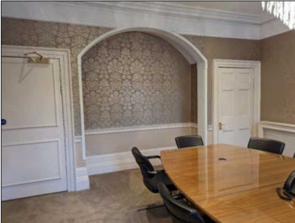
Plate 59: Inserted walls forming alcove
