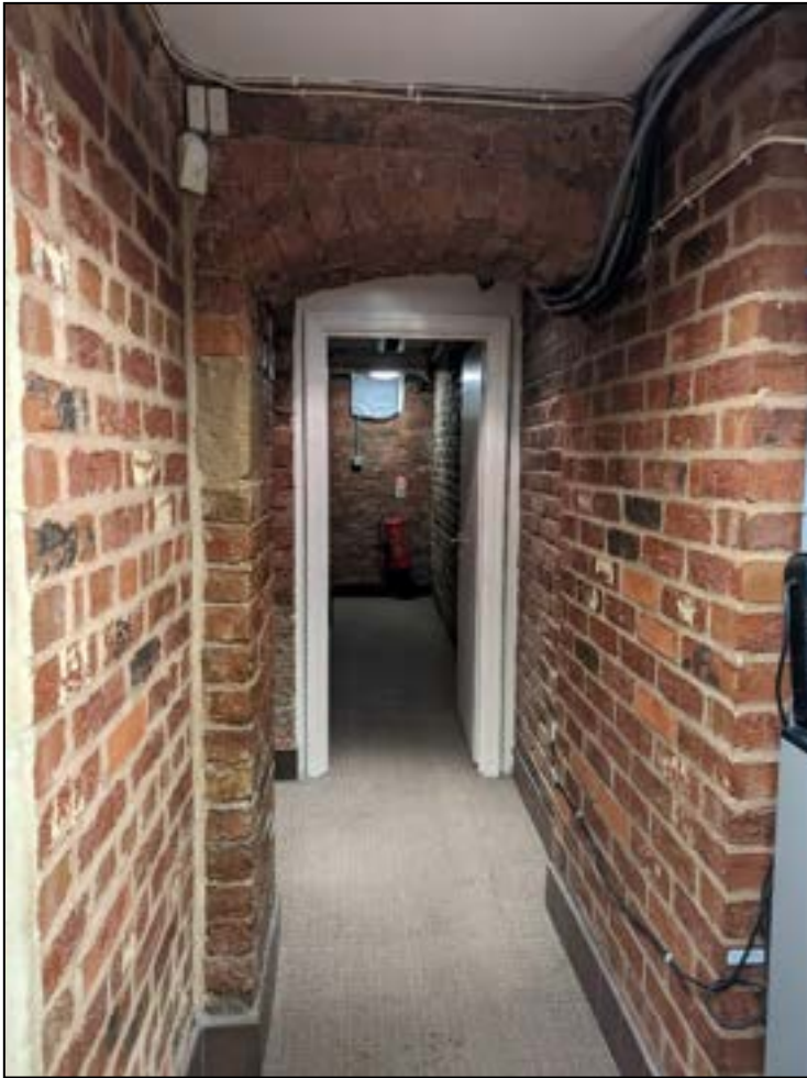
Plate 44: Corridor showing doorway to be removed (item 5)
