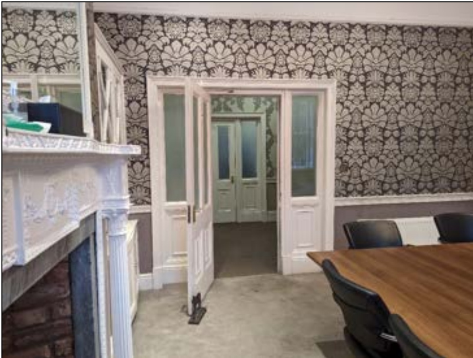
Plate 28: Inserted doorway to room 3
