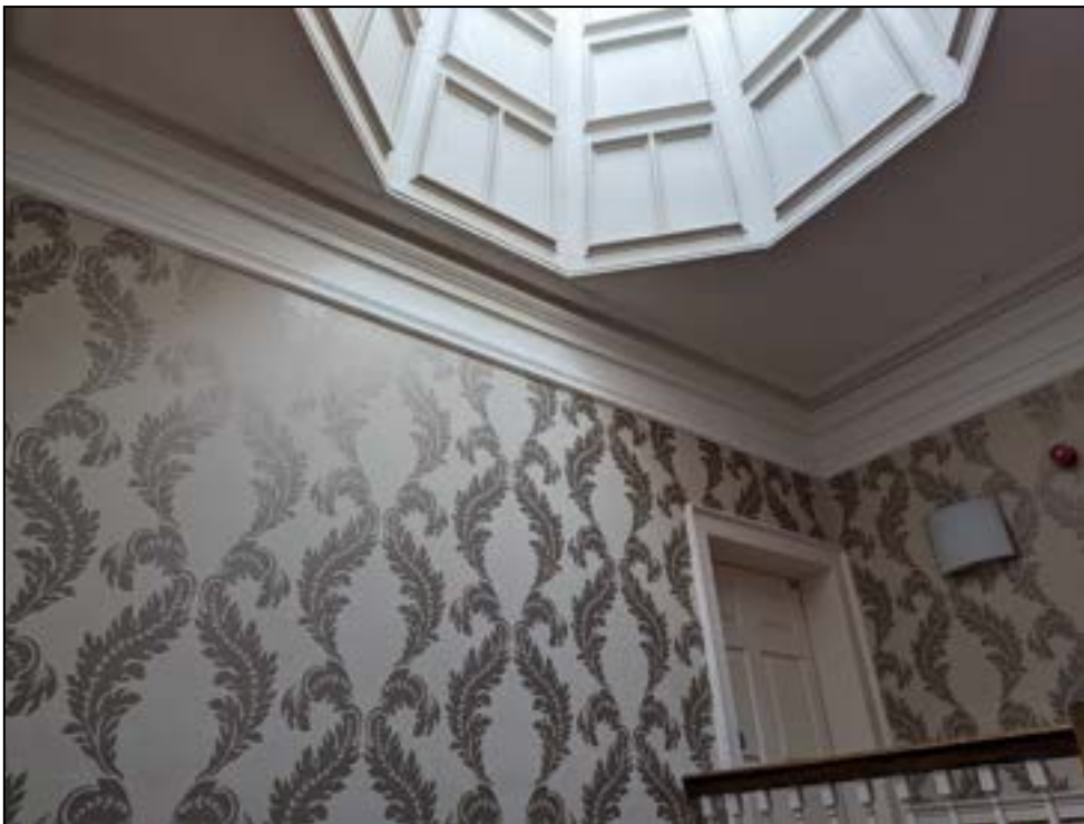
Plate 70: Lightwell over landing
