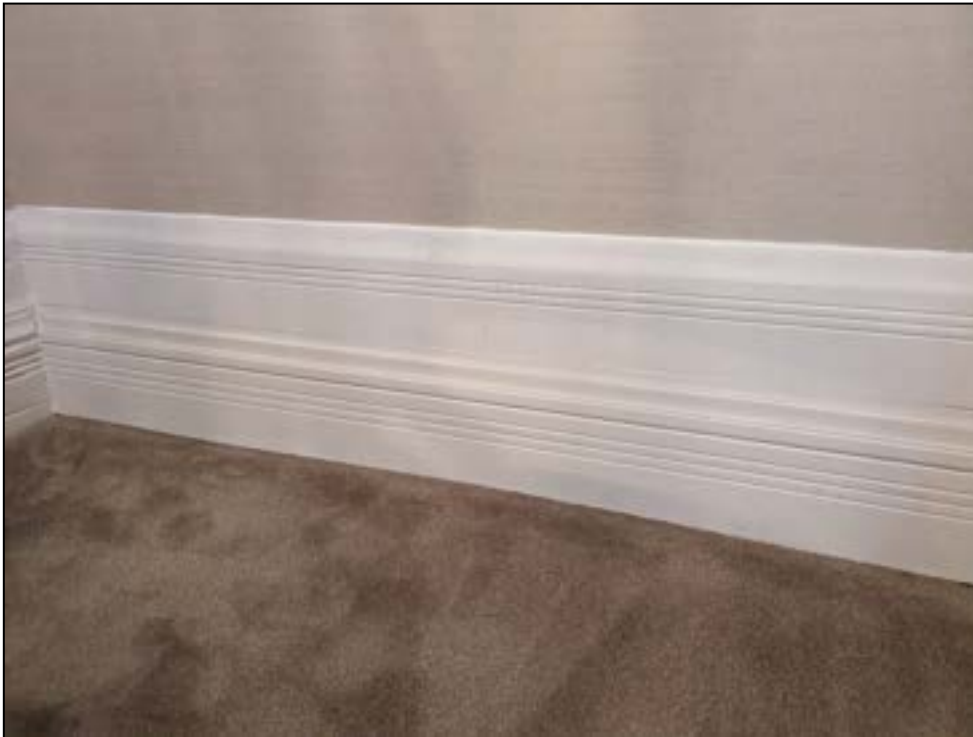
Plate 64: Detail of modern skirting to item 8
