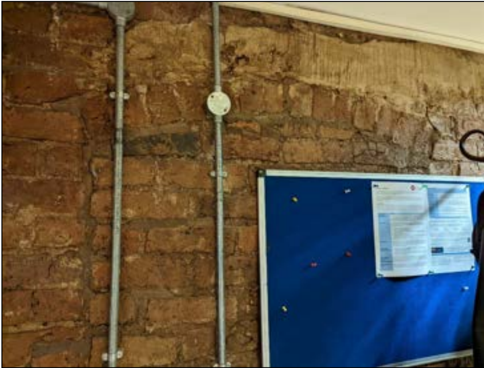
Plate 49: Blocked doorway into room 8 (item 7)
