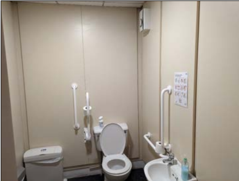
Plate 35: Inserted WC on other side of blocked doorway (item 1)
