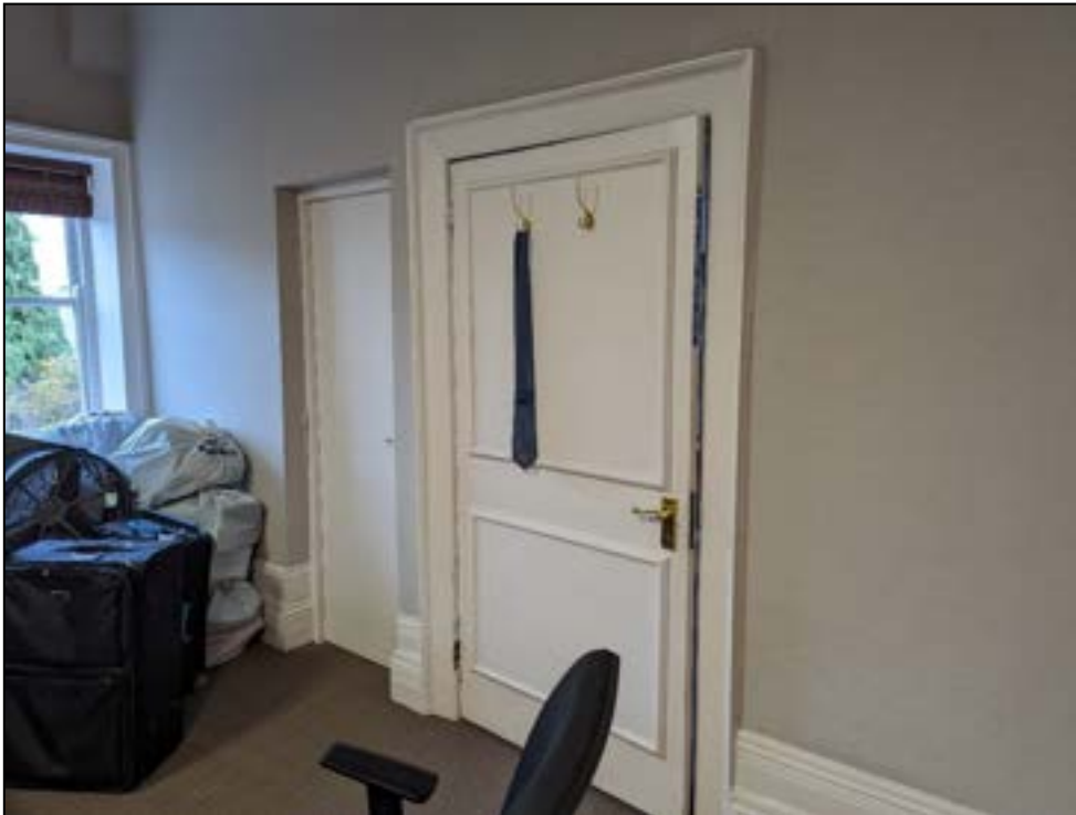
Plate 74: Doorways to room 15 (left) and landing (right)
