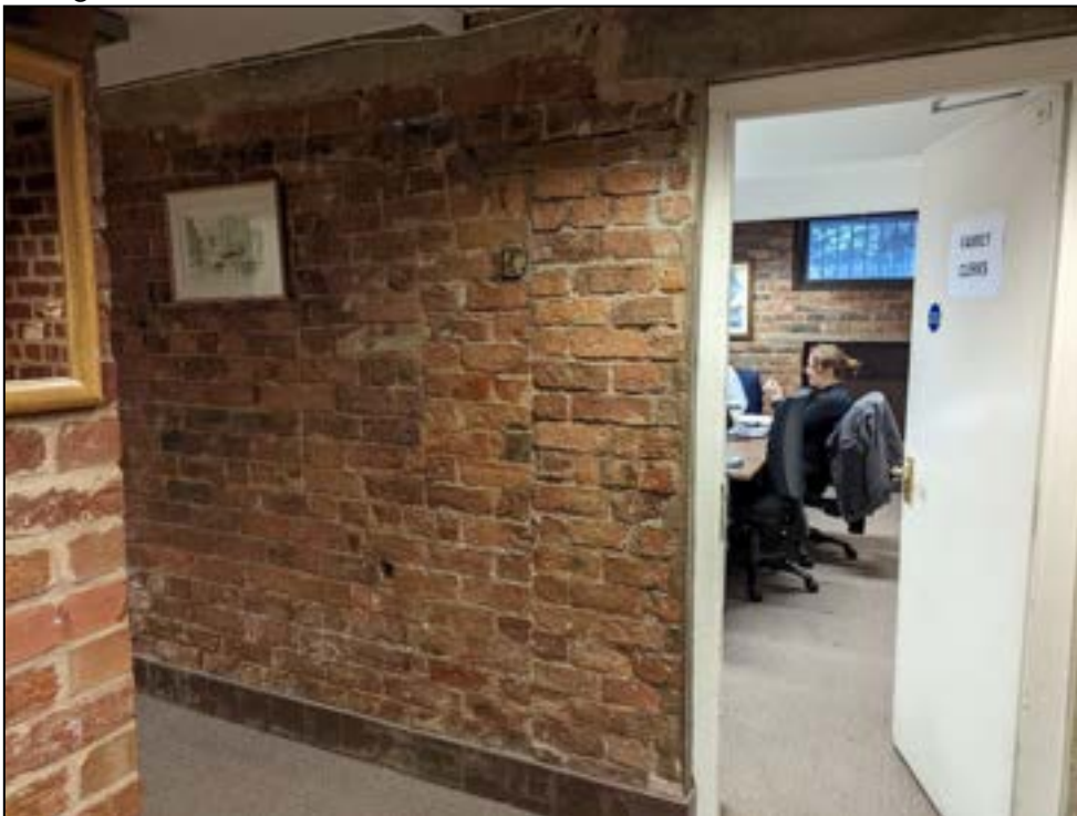
Plate 46: Item 5 as above showing straight joint from blocked doorway
