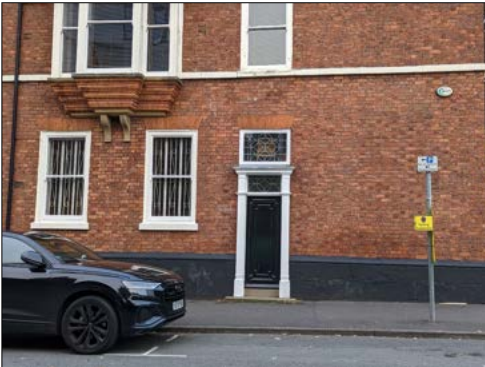
Plate 12: Ground floor doorway and windows
