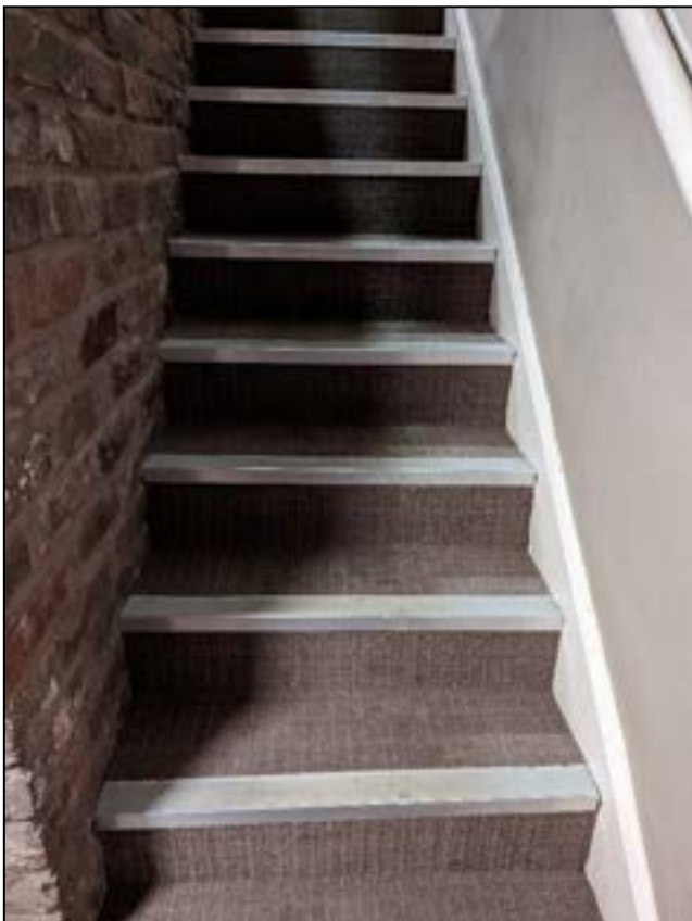
Plate 36: Basement staircase (item 3)
