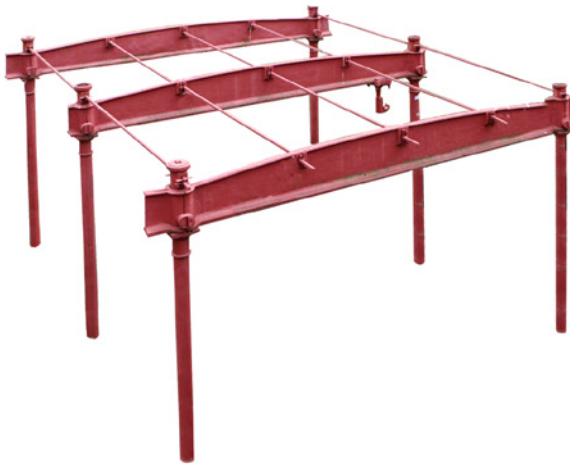
Above: A salvaged remnant of Havelock Mill's distinctive red frame was relocated to the University of Manchester Institute of Science and Technology (UMIST) as a structural monument and remains today.
