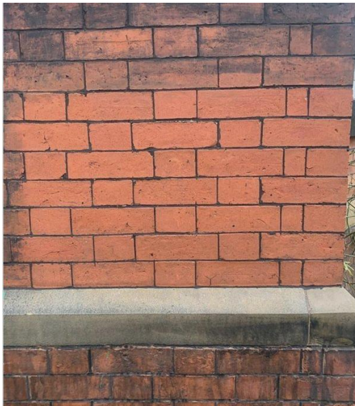
Washed existing brick on left side of the building
