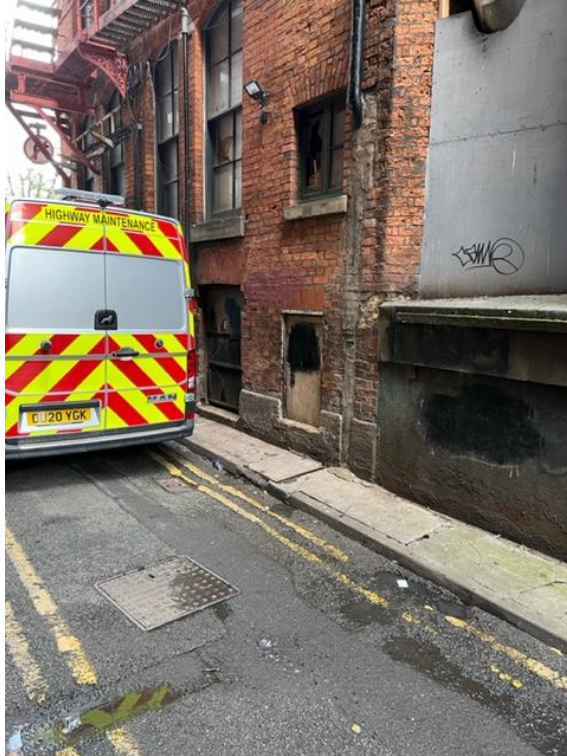
Photo 9, Public sewer manhole location
