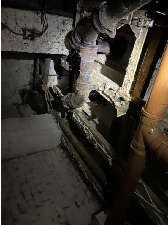
Photo 5, Drainage located in basement - RE2
