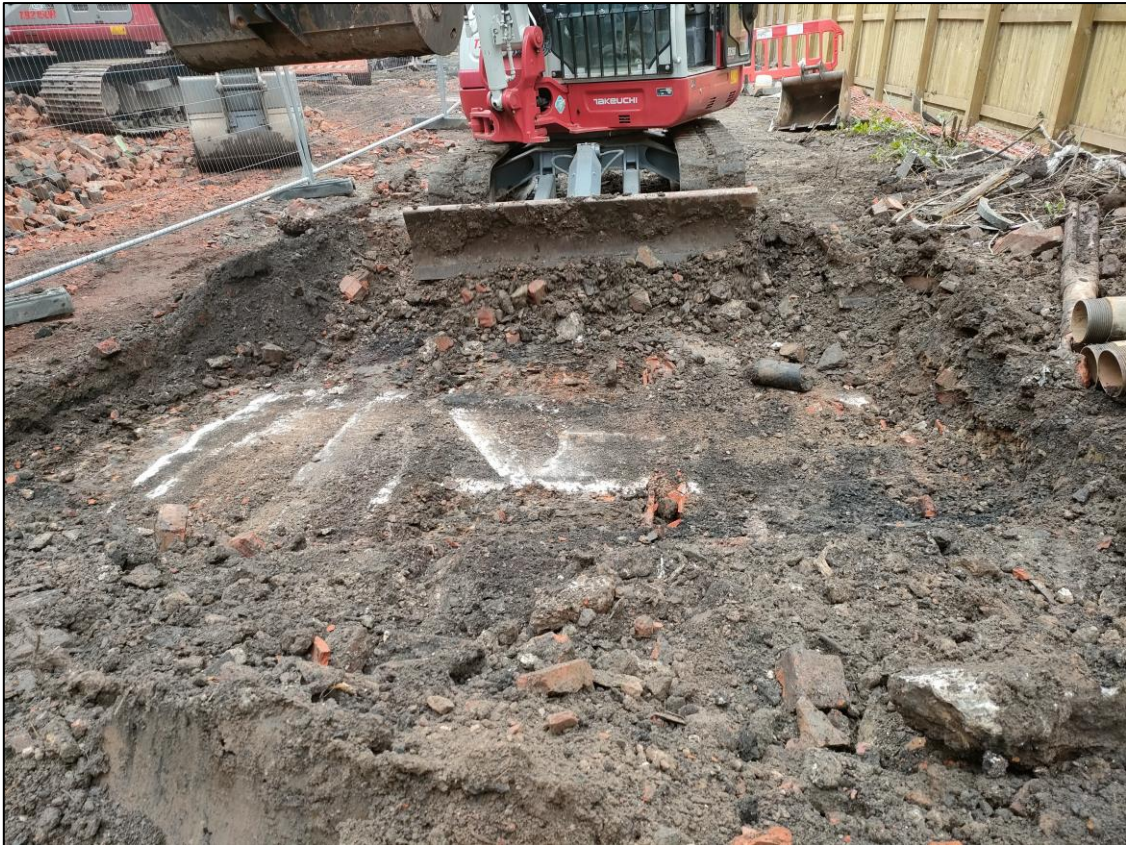
Plate 3: Concrete and rubble in the central area of the excavation
