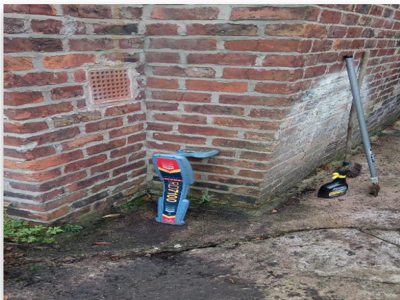
Fig 2.1: Trial Hole 2 Location
