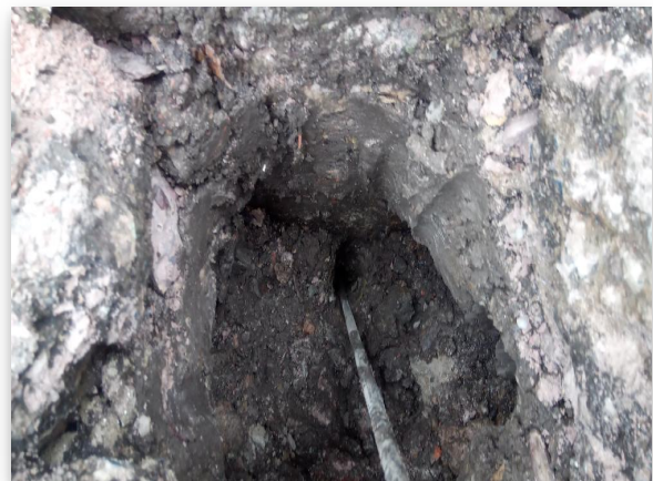
Fig 2.2: Trial Hole 2 Footing
