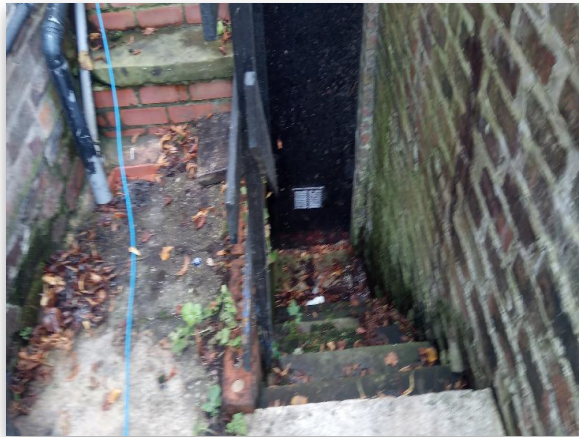
Fig 7.1: WG and steps to cellar.
