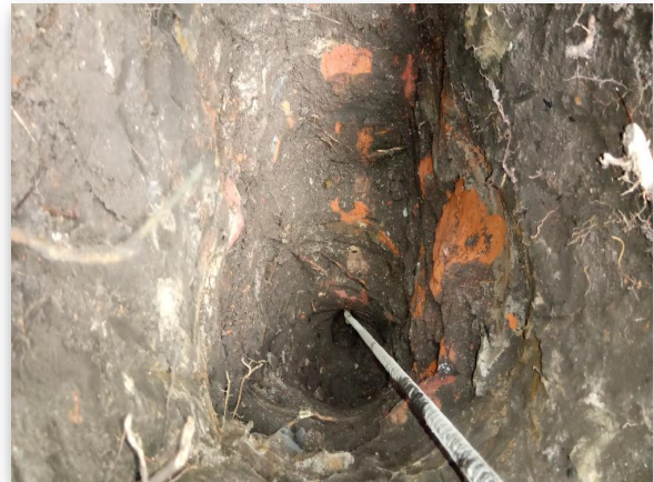
Fig 1.2: Trial Hole 1 Footing
