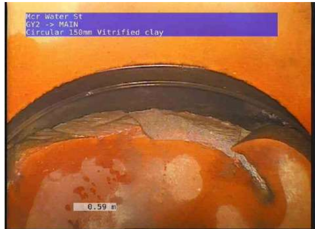
GY2X_fe931daa-49a9-48dd-afe6-b2ae47cc4b14_20221005_203856_417.jpg, 00:01:06, 0.59 m Open joint, large
