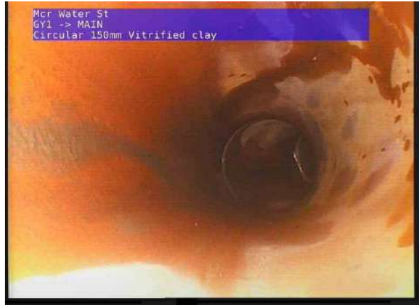
GY1X_c9148e46-e503-4938-8716-260d03f90f3f_20221005_203547_931.jpg, 00:00:47, 0.81 m Pipe material changes to vitrified clay at this point
