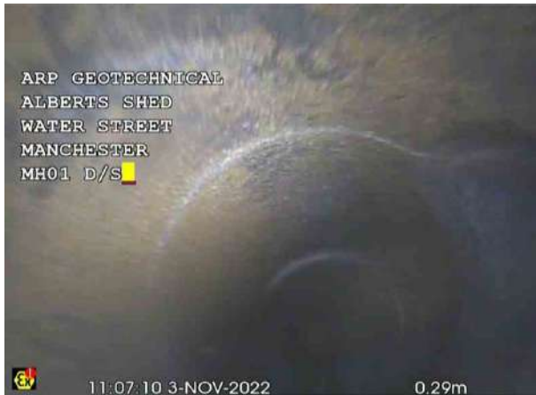
MH01X_6c986c9b-7597-4e10-bd14-b7b09cb2373c_20221103_111732_185.jpg, 00:00:04, 0.29 m Junction at 2 o'clock, 100mm dia
