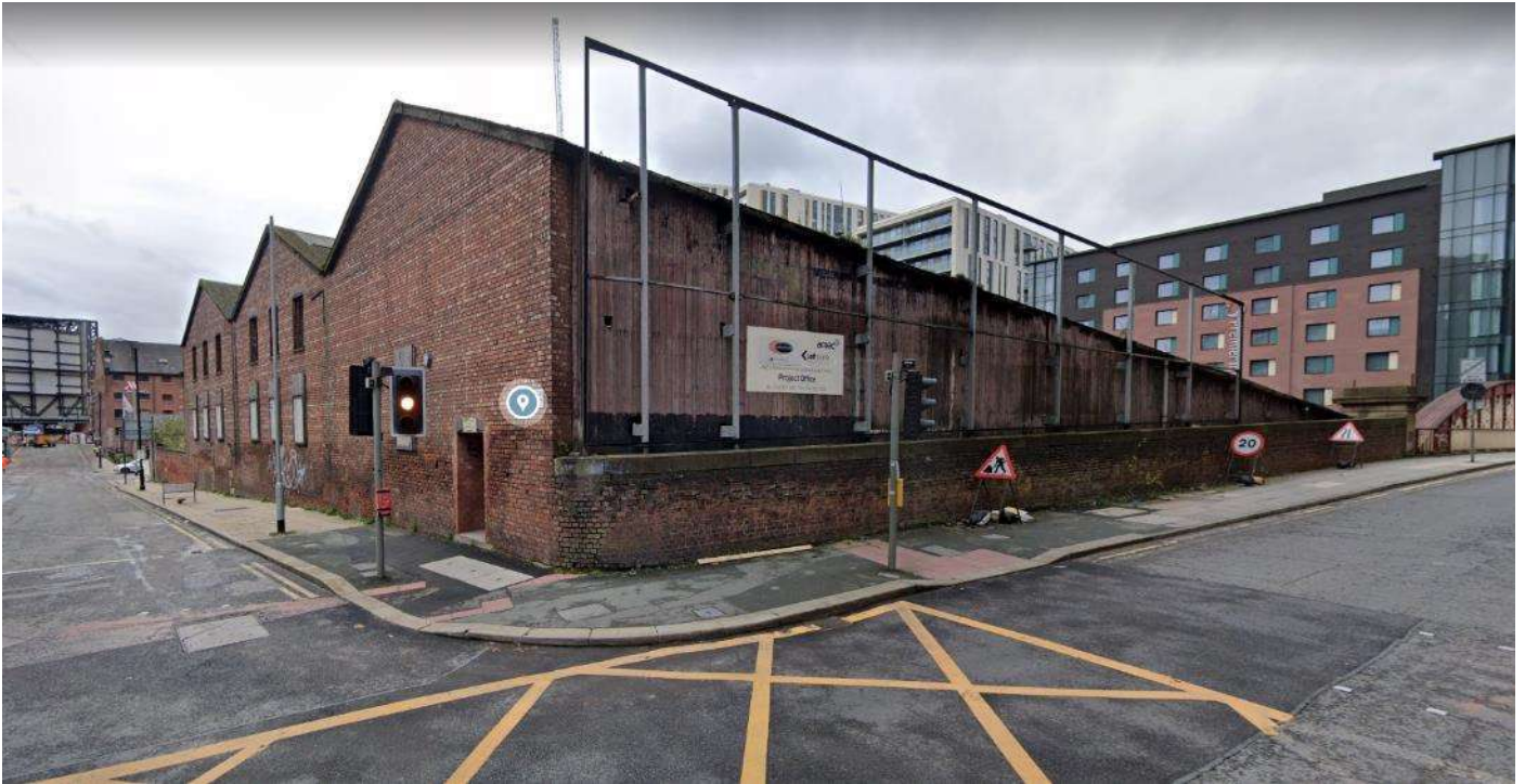
Photograph 1. View towards eastern corner of building from New Quay Street.
