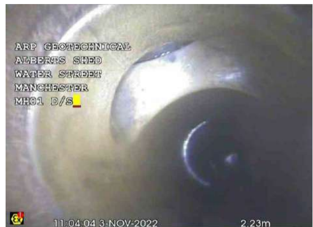
MH01X_544743af-6a54-4558-81e8-6a4bfb5db003_20221103_111557_598.jpg, 00:00:09, 2.23 m Junction at 11 o'clock, 100mm dia
