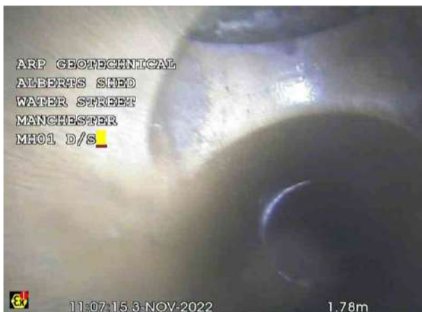
MH01X_73f03247-50e8-4c4d-a11c-fd4f8848867a_20221103_111802_241.jpg, 00:00:09, 1.78 m Junction at 11 o'clock, 100mm dia
