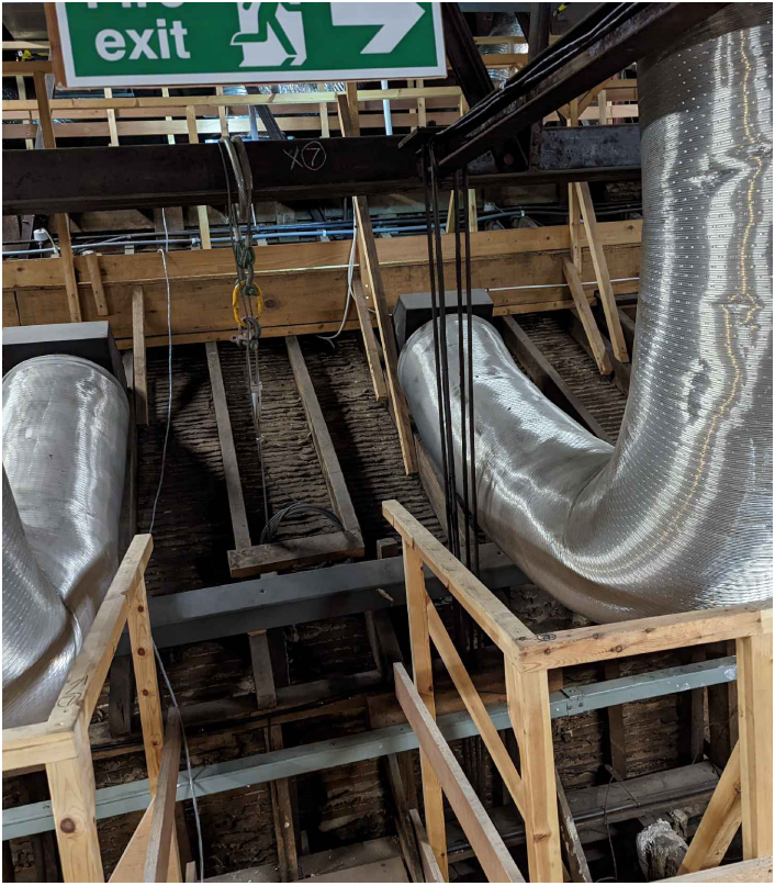
EXISTING LATH AND PLASTER PHOTOGRAPH
