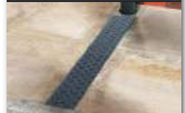
CHANNEL FOOTPATH DRAINAGE
