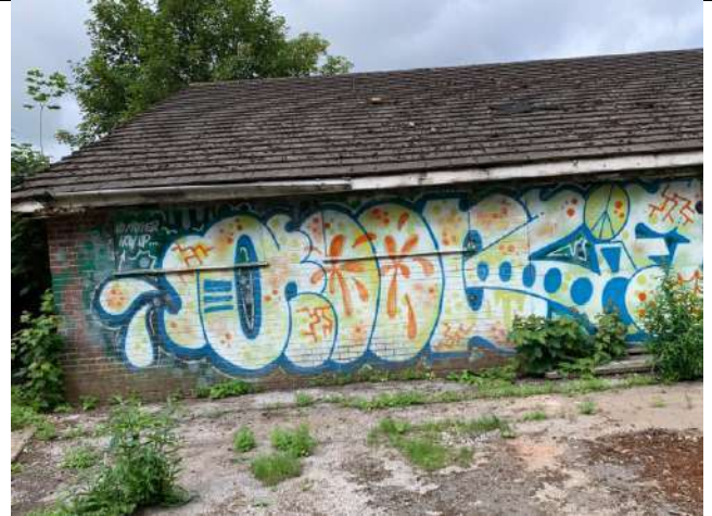
P10: Single storey building in west/south-west of site
