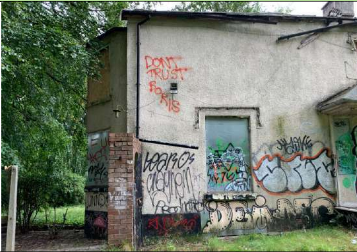
P5: Northern façade of building
