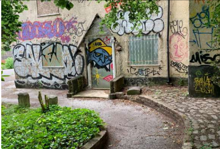
P3: View of eastern façade of two-storey building
