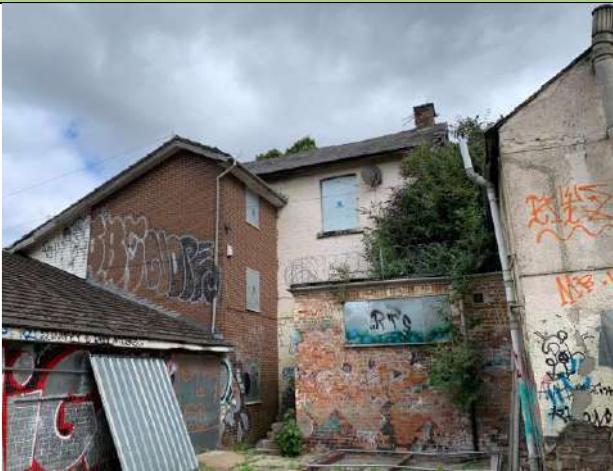
P11: Southern façade of building
