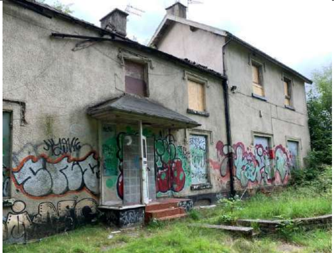
P4: Northern façade of building
