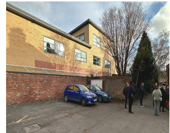
2 St Edward's site east boundary towards the Ryken Building
