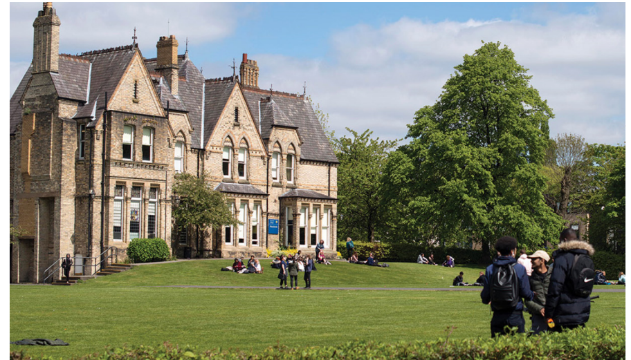
Marylands Building at Xaverian (Grade II Listed)
