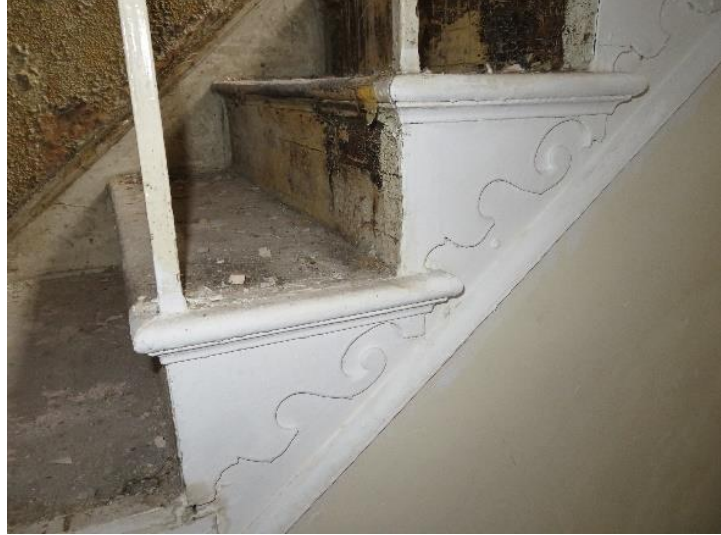
Upper ground floor decorated early 19 th century open string staircase with curved design brackets under the projecting treads.
