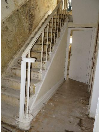
Upper ground floor decorated early 19 th century open string staircase with curved design brackets under the projecting treads.
