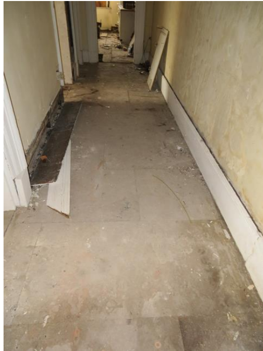
Dressed sandstone floor running to the rear of upper ground floor corridor.
