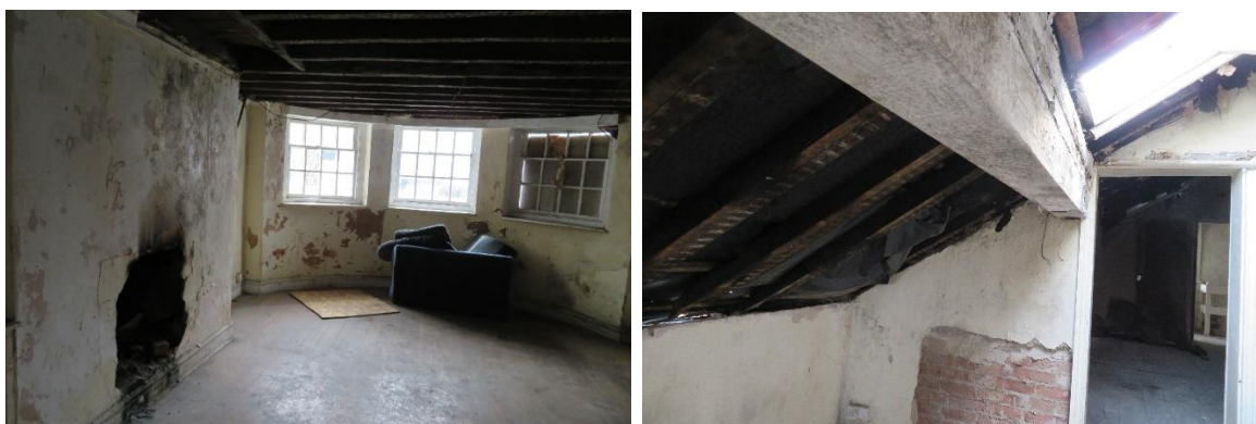
Left: Bay room in basement with 4 over 8 pane sash windows, low ceiling and simple skirting boards. Right: Attic room with smaller/lower door openings, no wall decoration.
