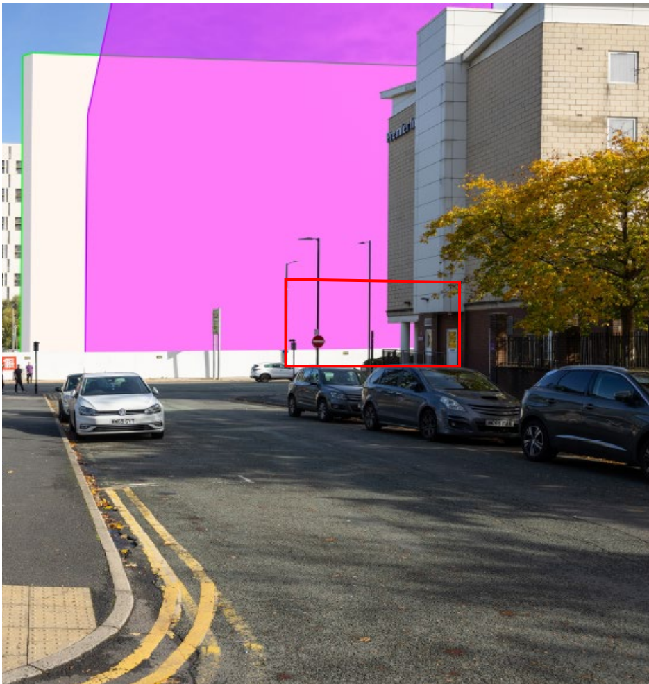
Figure 6.16 – View 11 of Chorlton Old Mill edged in red from Medlock Street in conjunction with Plot 10a edged in green and Plot 10b behind as well as Plot 9a in purple (under construction). (Planit-IE, 2023)
