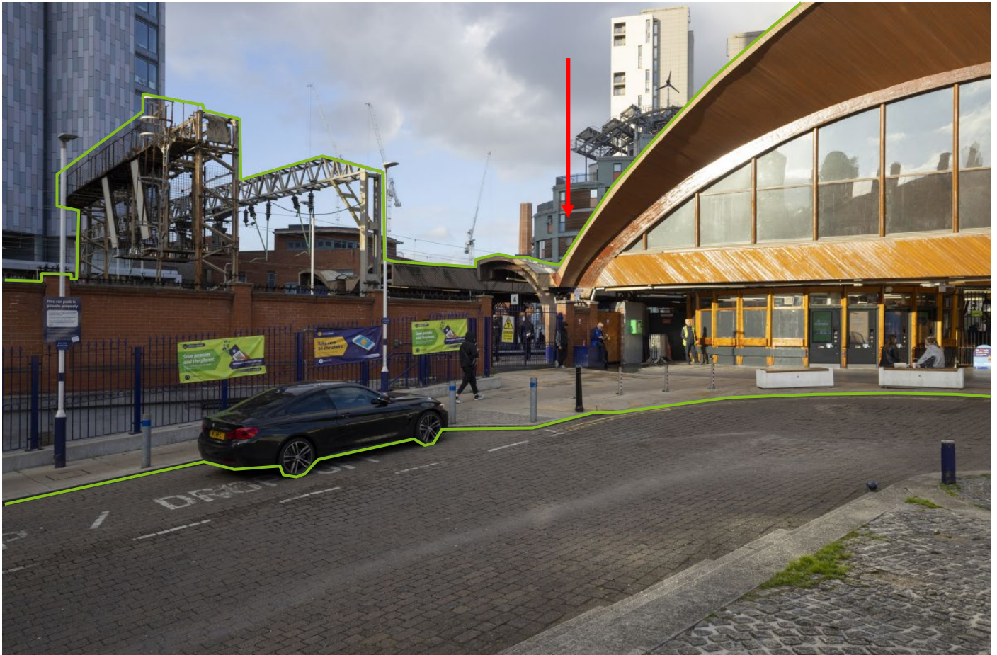
Figure 4.10 – View 9 of Manchester Oxford Road Station (including platform structures) in conjunction with the Site denoted by red arrow and heritage asset edged in green. Plot 11 is highlighted in orange (Planit-IE, 2022)
