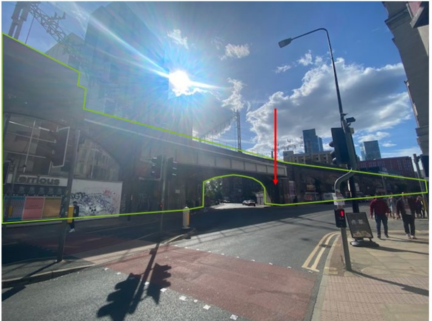
Figure 4.7– View of Manchester South Junction and Altrincham Railway Viaduct in conjunction with the Site denoted by red arrow and heritage asset edged in green. (Author's own, 2022)
