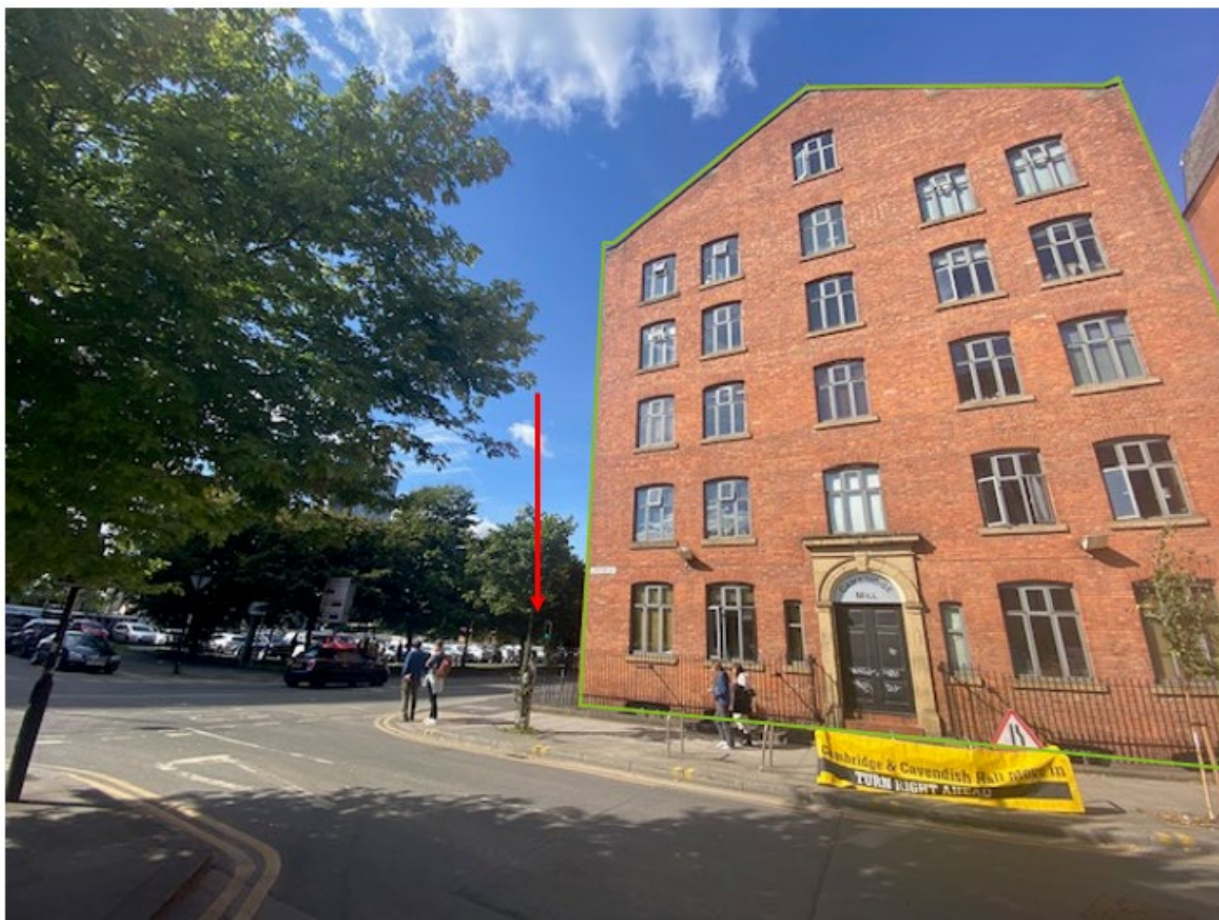
Figure 4.6– View of Mill on north east corner of junction with Chester Street in conjunction with the Site denoted by red arrow and heritage asset edged in green. (Author's own, 2022)
