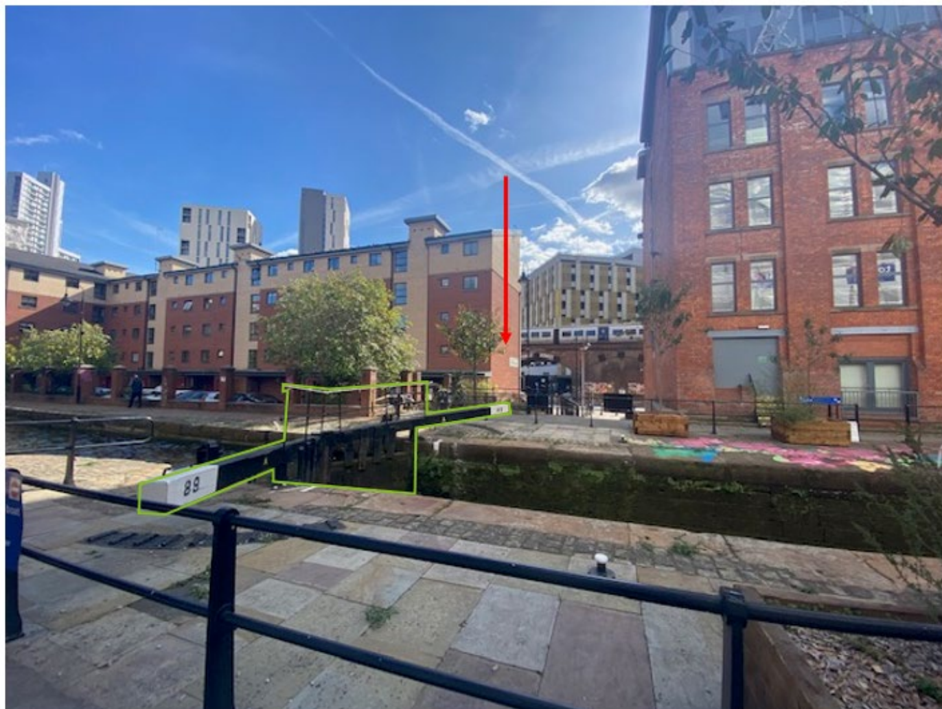
Figure 4.9 – View of Rochdale Canal lock number 89 (Tib Lock), on south side of Havelock Mills in conjunction with the Site denoted by red arrow and heritage asset edged in green. (Author's own, 2022)
