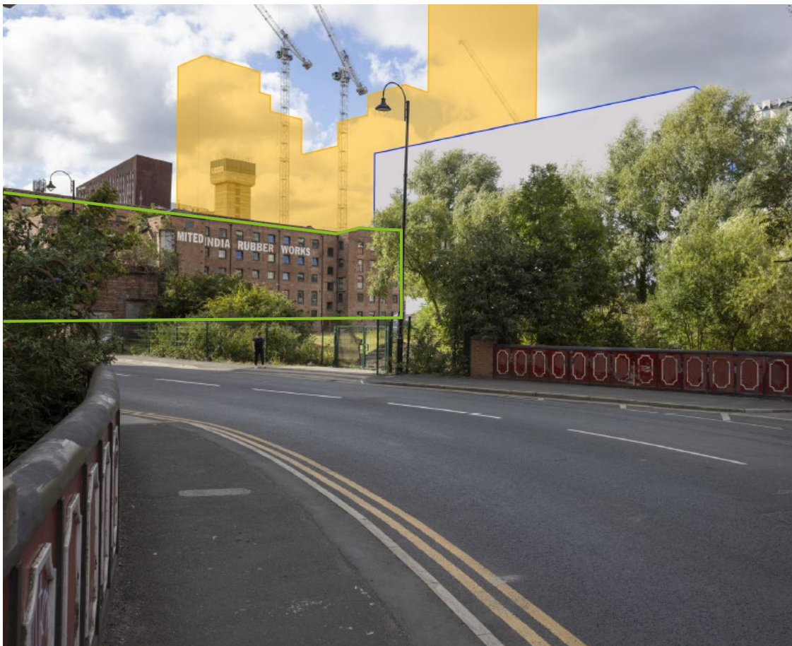
Figure 6.1 – View 4 of Macintosh Mill edged in green from the north-east in conjunction with Plot 10b edged in blue and Plot 11 in yellow (under construction). (Planit-IE, 2023)
