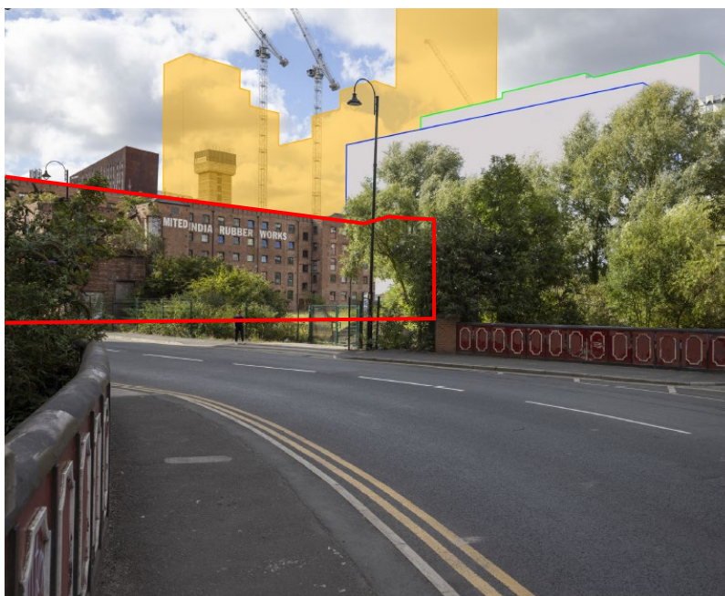
Figure 6.5 – View 4 of Macintosh Mill edged in green from the north-east in conjunction with Plot 10b edged in red, Plot 10a in green and Plot 11 in yellow (under construction). (Planit-IE, 2023)
