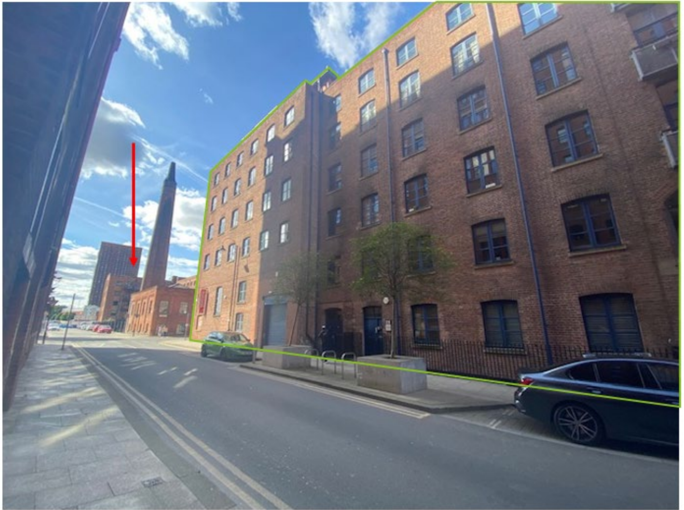
Figure 4.4 – View of Chorlton New Mill in conjunction with the Site denoted by red arrow and heritage asset edged in green. (Author's own, 2022)
