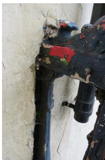
Left & Right: Rear close up views of the upper cast iron balustrades by the main entrance. Evidence of a previous plate enclosing the open rear faces of the balustrades.
