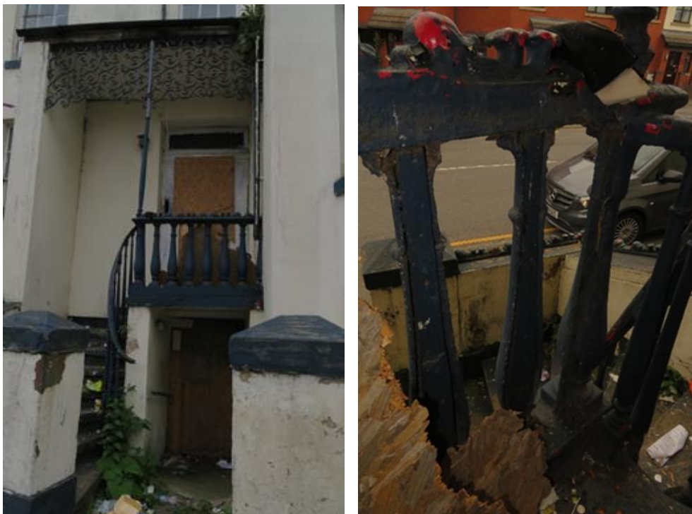
Left: Painted balustrades, handrail, support column and wrought iron screen at the main entrance fronting Higher Ardwick. Right: A rear view of the upper cast iron balustrades by the main entrance. Evidence of a previous plate enclosing the open rear faces of the balustrades.
