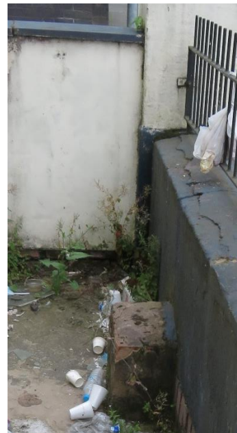
Left: The existing length of 20 th century railings to the south of the main entrance pillar. Right: An existing internal masonry plinth showing previous use as a stanchion base for railings.
