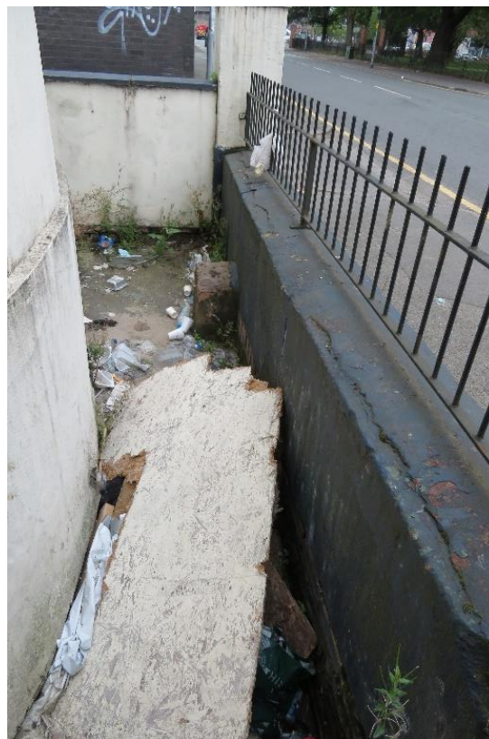
View looking south at the existing Higher Ardwick wall, Modern low railings and brick buttress survives for previous railing stanchion.
