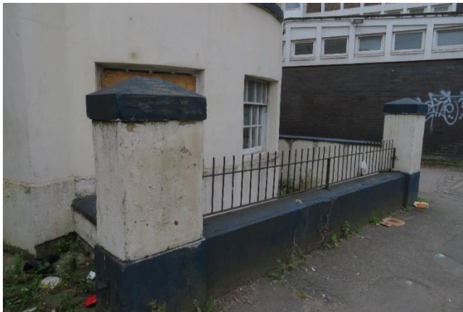
Left: The existing length of 20 th century railings to the south of the main entrance pillar. Right: An existing internal masonry plinth showing previous use as a stanchion base for railings.
