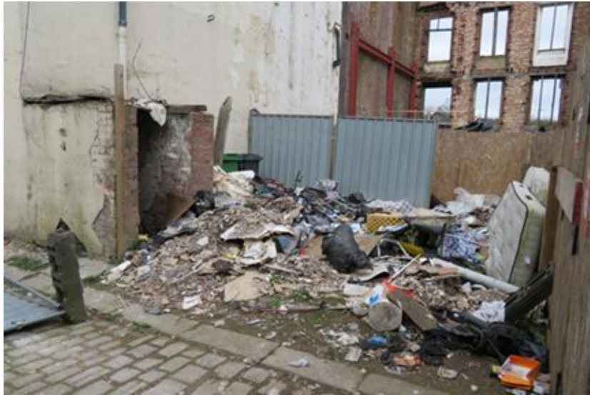
The existing compound area to the rear and south east of Fenton House. Note the preservation of historic stone setts/cobbles.
