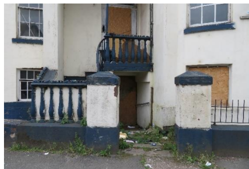
Left: Low painted boundary wall fronting Higher Ardwick. Right: The pillars flanking the main entrance. Modern low quality railings to right with cast iron balustrades to left.
