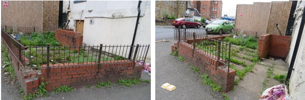
Left: Modern low poor quality red brick wall and railings to the north of Fenton House fronting Higher Ardwick and Harkness Road. Right: Enclosures viewed from Higher Ardwick with low wall by north basement entrance to the right.
