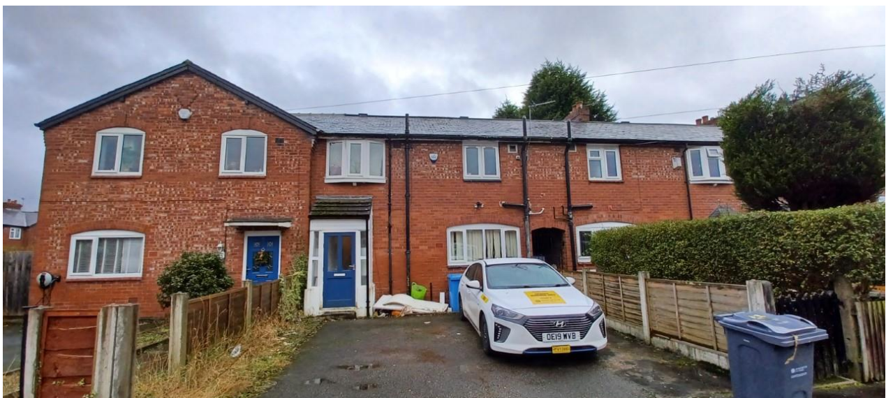
Figure 1. Photograph of the principal elevation of No.6 Abergele Road.
