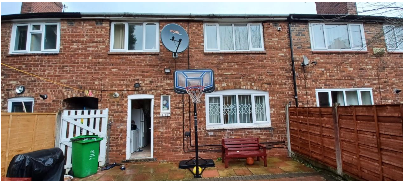
Figure 2. Photograph of the rear elevation of No.6 Abergele Road.
