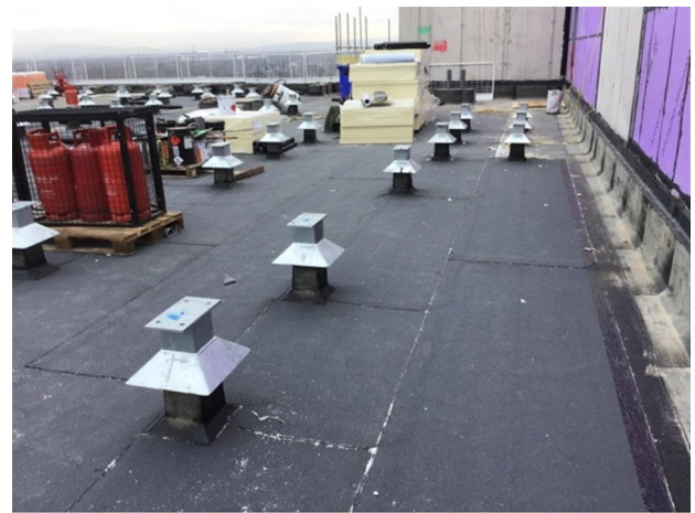
Photo 6 - View of cap sheet to level 9
