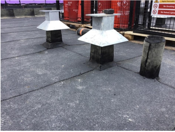
Photo 9 - View of steel support
