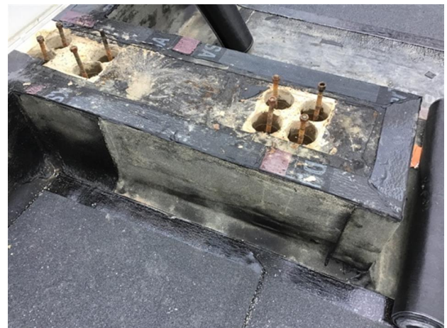
Photo 8 - View of two layer underlay up stand
