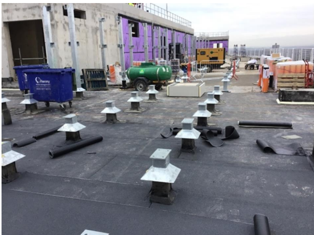
Photo 1 - View of progress to section 1
