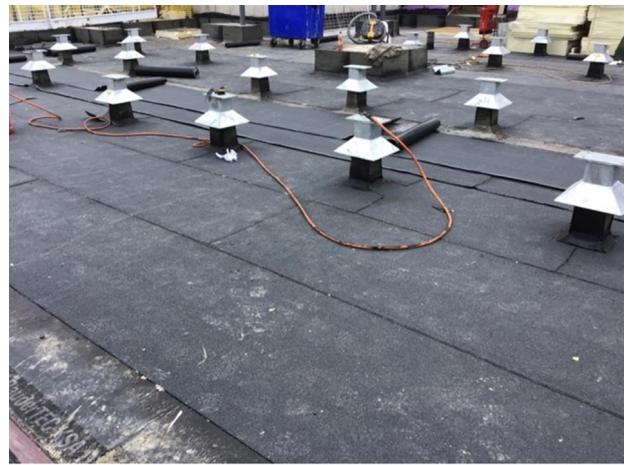
Photo 12 - View of cap sheet to level 9
