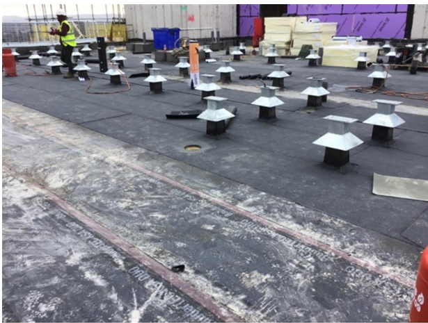
Photo 5 - View of progress to level 9
